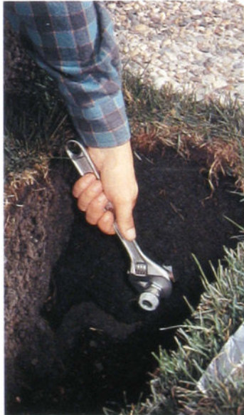
8 Attach a compression fitting and plastic bushing to each end of the conduit. The plastic fittings will prevent the sharp edges of the conduit from damaging the cable sheathing.
