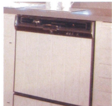
Dishwashers and food disposers require dedicated 15-amp 120-volt circuits (most local codes). Some inspectors allow these appliances to share one circuit.
