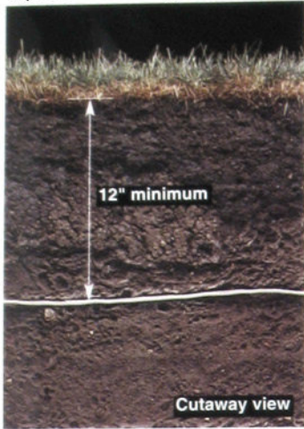
Bury UF cables deep if the by a GFCI r than 20 amps 18" deep if the ected by a GFCI 20
