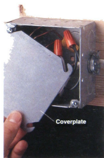
9 Carefully tuck the wires into the box and attach the coverplate. Turn on the power to the circuit at the main service panel. Make sure the box remains accessible and is not covered with finished walls or ceilings
