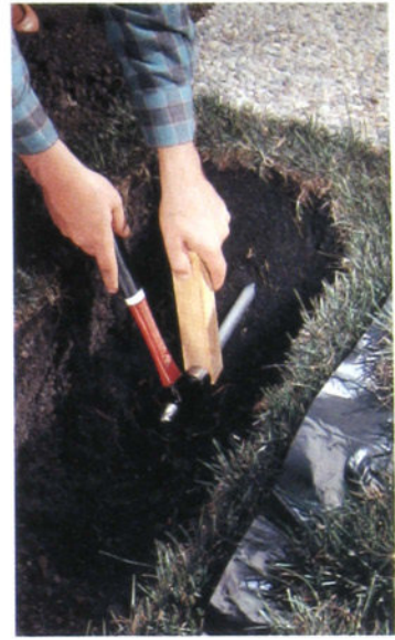
6 Drive a ball-peen hammer on the wood block to flatten the pipe.
