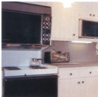
Ranges require a dedicated 40- or 50-amp 120/240-volt circuit (two circuits for separate oven and countertop units). Even if you do not have an electric range, it is a good idea to install the circuit when remodeling.
