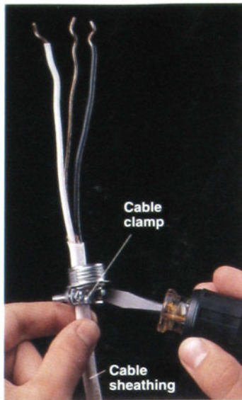
5 Thread each cable through the cable clamp. Tighten the cable clamp with a screwdriver. Do not over-tighten. OV
