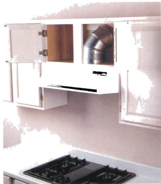
Cabinet-mounted vent hood is attached to the bot- tom of a short 12" to 18" tall wall cabinet. Metal ducts run inside this wall cabinet.
