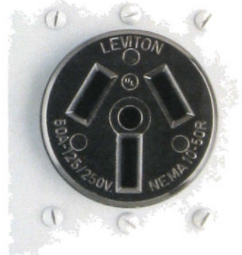
50 amps, 125/250 volts. This receptacle is used for ranges. The high-voltage current powers heating coils, and the 125-volt current runs clocks and lights.
