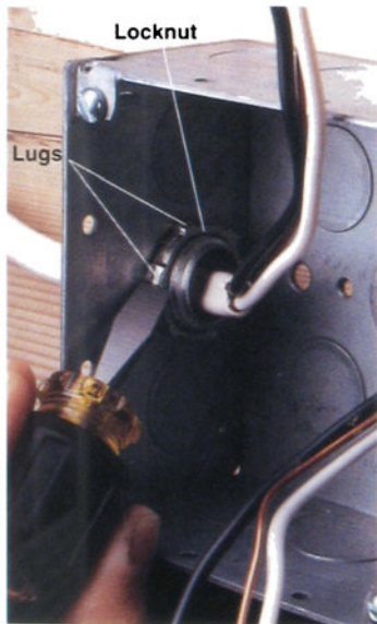
7 Tighten the locknuts by pushing the locknuts onto the lugs with the blade
