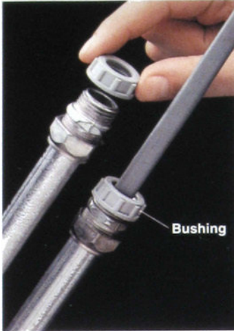
Protect cable entering conduit by attaching a plastic bushing to the end of Th
