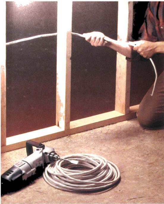
Pulling cables through studs straight holes. Use the same straightening the cable before the studs.
