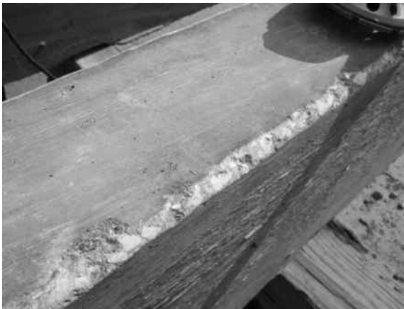
FIGURE 8.5 Rounded beam corners by grinding.
