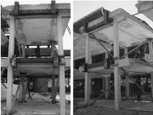
Figure 4.35 The RC structure equipped with BRBs.
