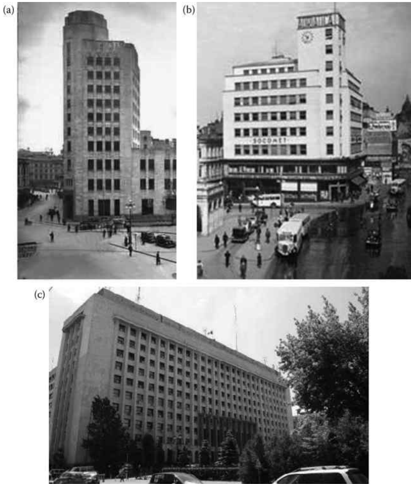
Figure 1.61 Multistoried buildings damaged during the 1977 Vrancea earthquake: (a) Victoria telephone exchange office; (b) Adriatica building; (c) Ministry of Transport building.
