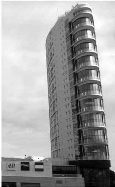
Figure 2.28 Steel structures in Lisbon, Portugal, for new buildings in the Expo area.
