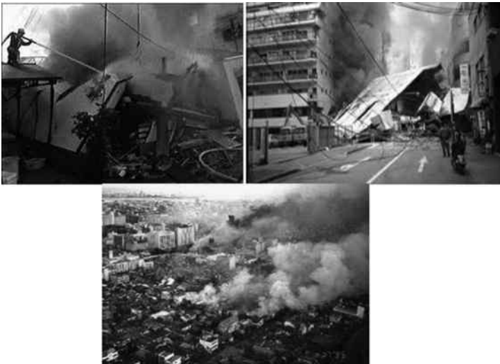
Figure 6.9 The Kobe earthquake (Japan, 1995).
