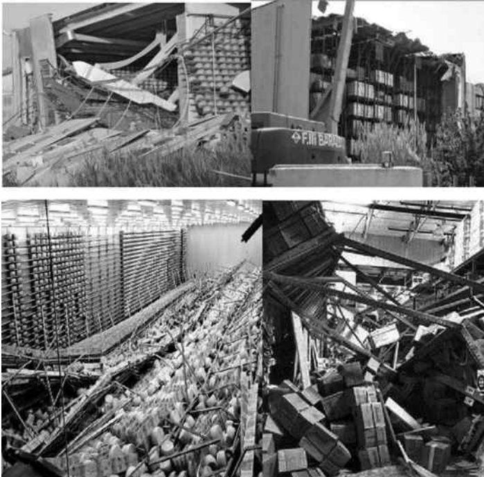
Figure 1.68 The collapse of industrial shelves during the Emilia earthquake. (Faggiano, B. et al. 2012: Steel buildings within the Emilia earthquake (in Italian). Progettazione Sismica , n.3, IUSS Press, ISSN 1973–7432.)
