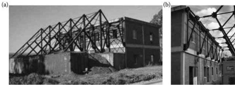
Figure 4.42 Reacting structure (a) and hydraulic jacks (b).
