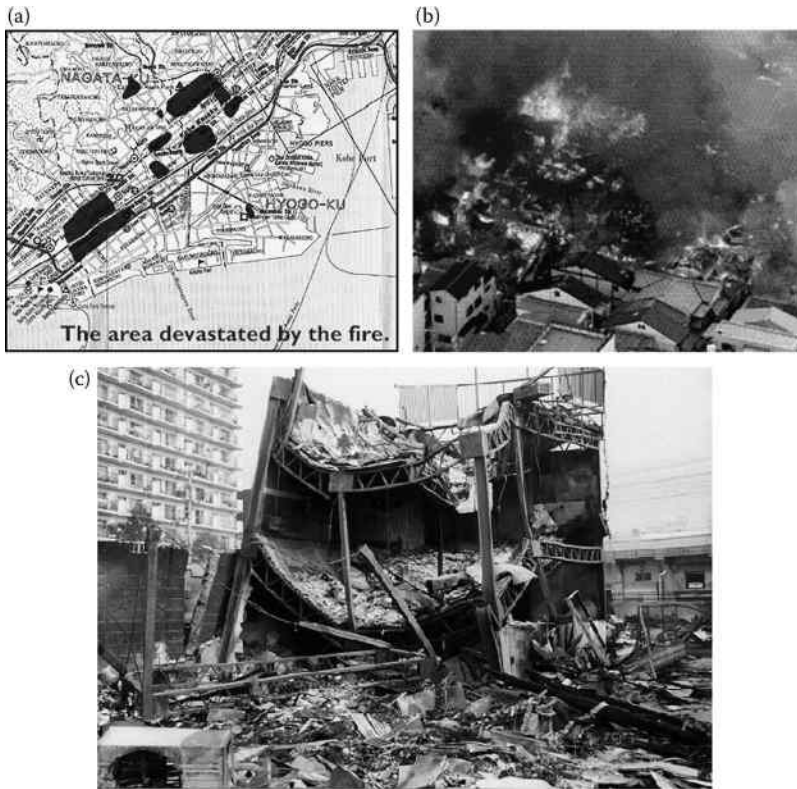
Figure 1.41 Fire after earthquake in Kobe: (a) area interested by fire; (b) aerial view of fire; (c) a building destroyed by earthquake followed by fire.
