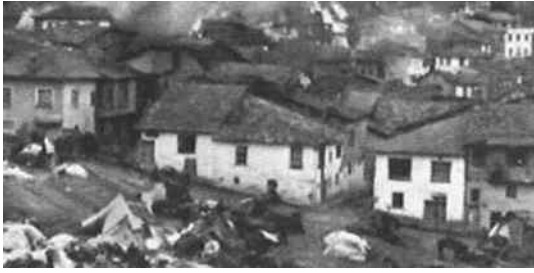
Figure 6.6 The Gediz earthquake (Turkey, 1970).
