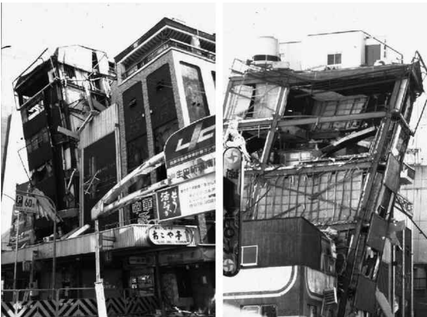
Figure 1.31 Damage of a steel structure. (Gioncu, V., Mazzolani, F.M. 2002: Ductility of Seismic Resistant Steel Structures . Spon Press, London; after Fischinger, M. 1997: EASY, Earthquake Engineering Slide Information System. FGG-IKPIP Institute Slovenia.)
