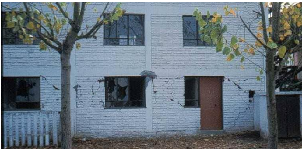
Figure 1. Three-story confined masonry building; Melipilla, Chile, on March 3, 1985.
