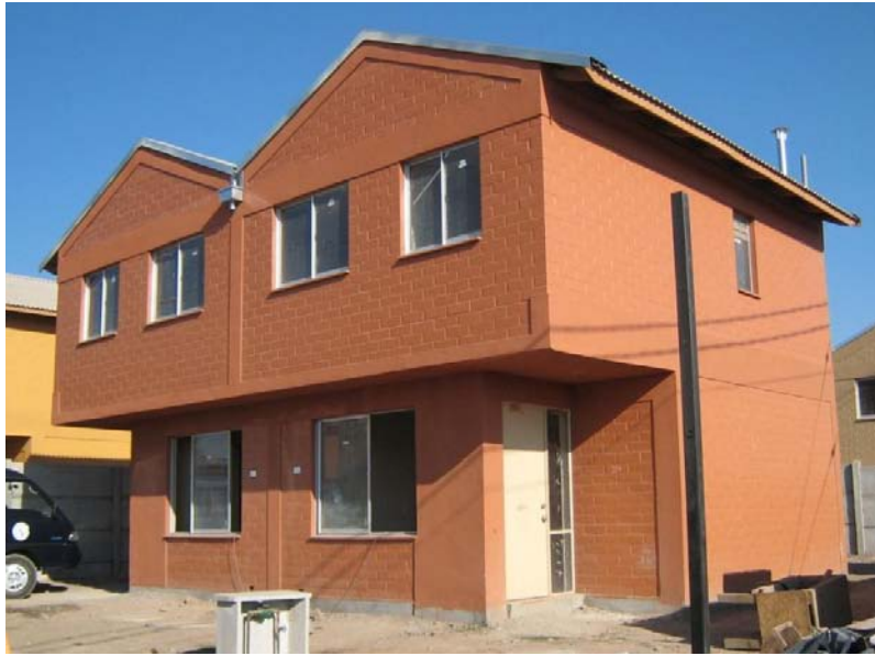
Figure 2. Front view of test structure.
