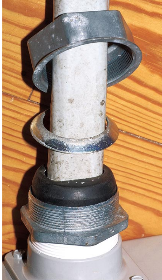
Three pieces of a seal: rubber grommet, anti-grab washer, and screw cap.
