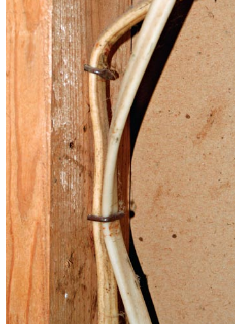
Hitting a staple one too many times can short out a single cable (top), and placing too many cables under a staple can do the same (bottom).
