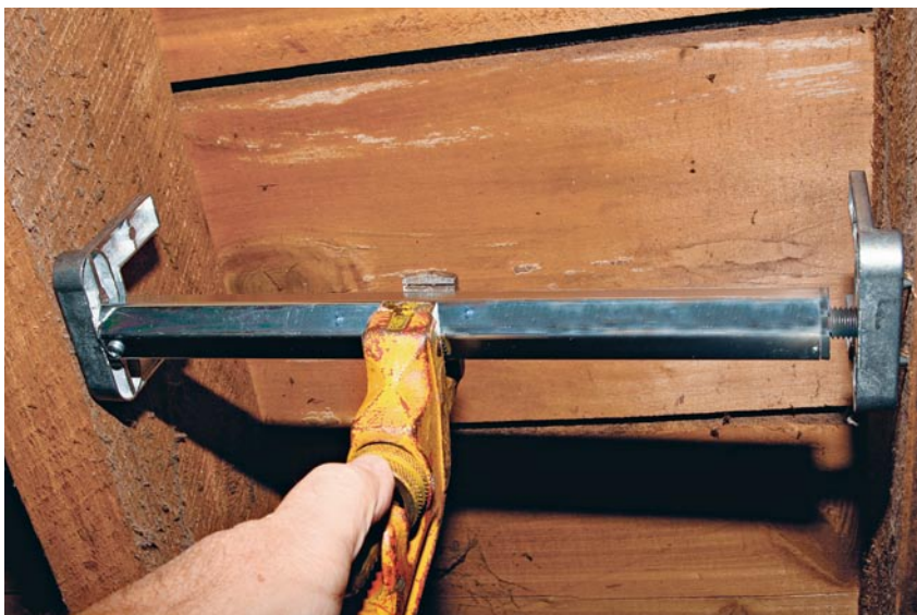
For a heavy-weight fan use a heavy-weight support. Always assume it is your head under the fan if it comes crashing down.
