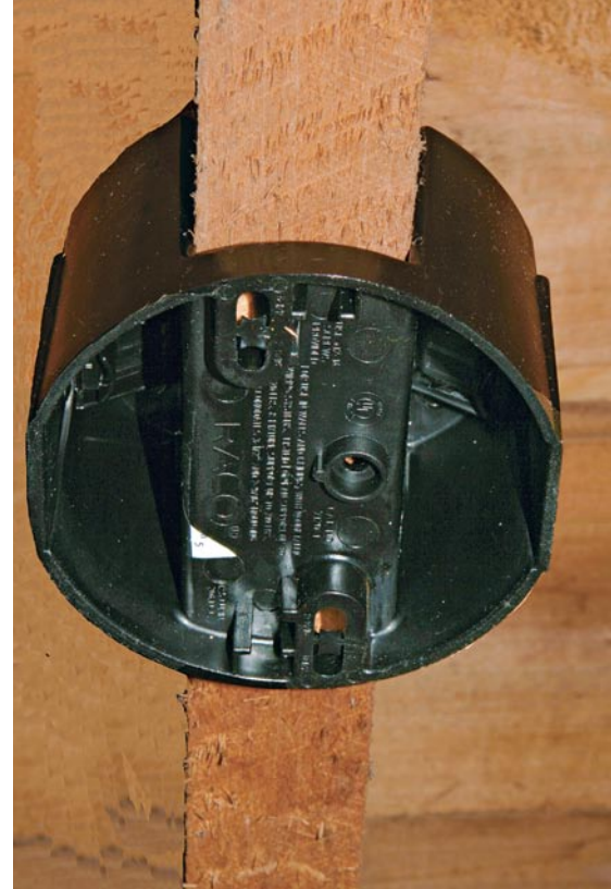
Plastic boxes are now listed for ceiling fans but I am wary of them.
