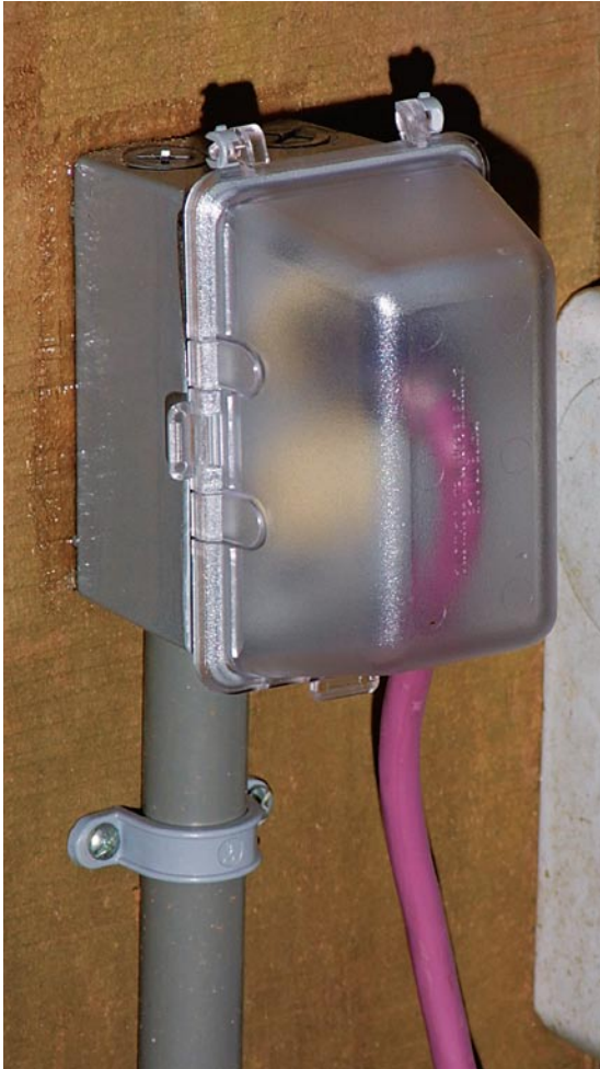
A watertight-while-in-use lid has a bubble to protect the receptacle and plug from rain and snow while a cord is plugged in.
