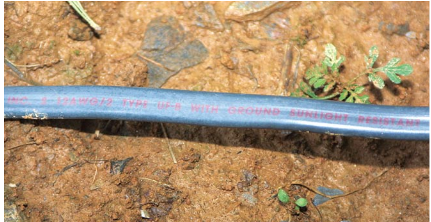
Use UF cable for wet and buried locations.
