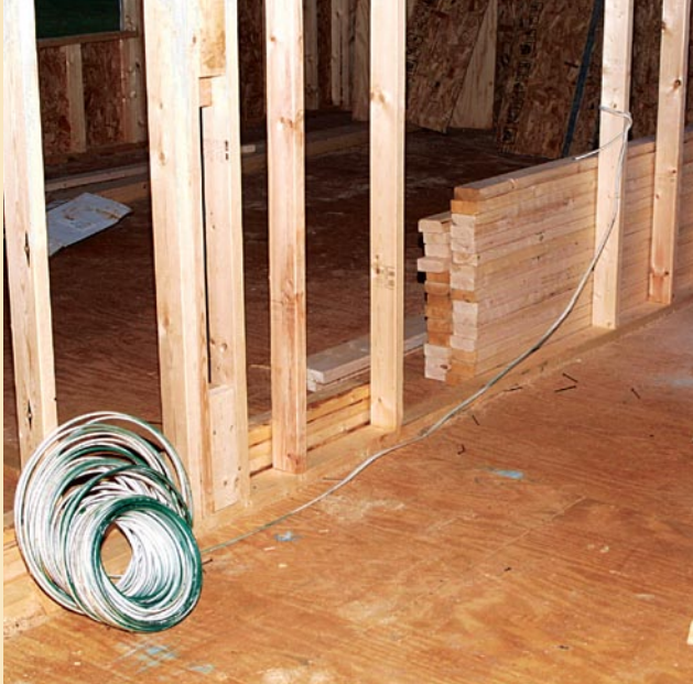
Unrolling cable like a bait-casting reel will keep it from spiraling.
