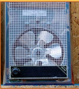
286 | Electric Wall Heaters
