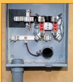
78 | Connecting Meter Base to Panel
