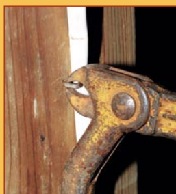
157 | Routing Wires in Renovation Work
