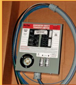
314 | Transfer-Switch Style
