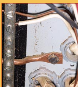
96 | Bringing Cables into the Panel
