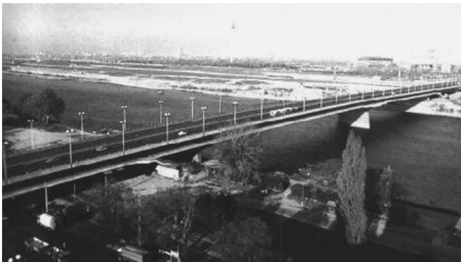
Fig. 18.15 A concrete twin-box-girder bridge was opened in November 1980. This bridge is also called the Reichsbrücke. ( www.reichsbruecke.net/geschichte_e.php )
