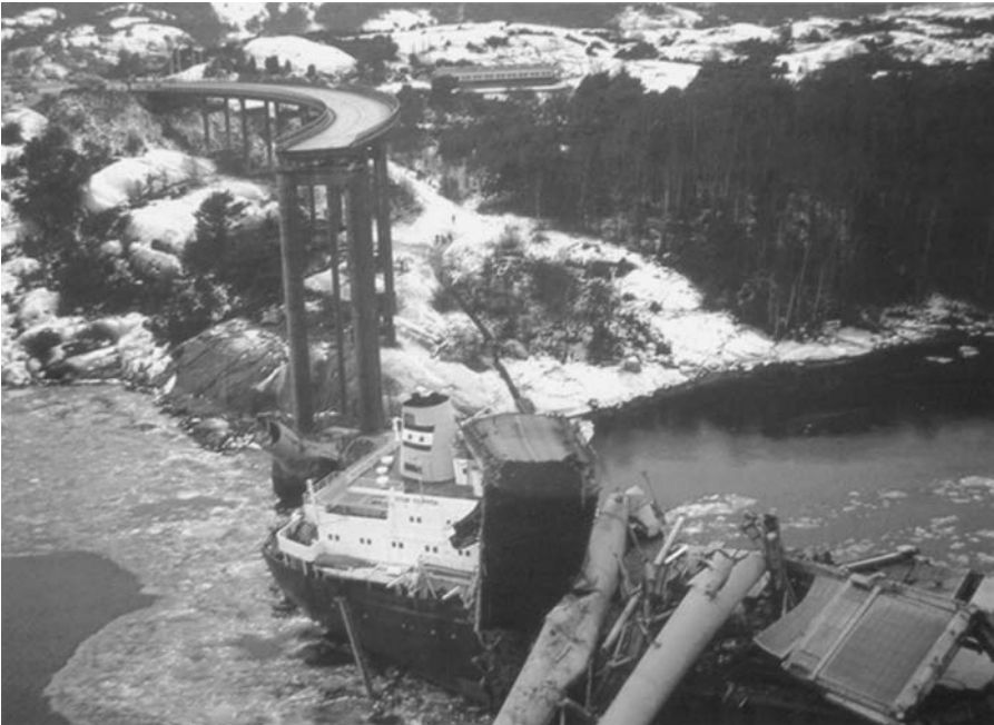
Fig. 19.8 The collapse of the Almö Bridge. (Tjörnbron. The Swedish National Road Administration. With kind permission of Lennart Lindblad)
