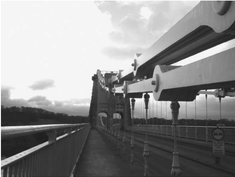
Fig. 11.5 The eye-bar chain suspension bridge at Menai Strait, Wales, similar in design to that of the Point Pleasant Bridge. ( www.anglesey.info/Menai%20Bridges.htm , with kind permission of Phil Evans)
