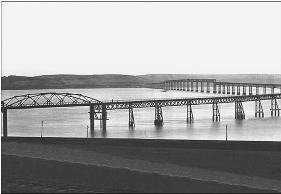
Fig. 3.2 The Tay Bridge, which was built in 1878. (Wolcott: The breaks of progress. Mechanical Engineering)
