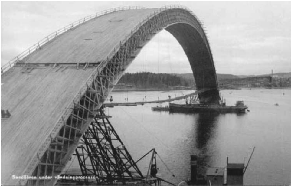
Fig. 6.2 The timber arch falsework being shipped into position. ( www.famgus.se/Gudmund/Gudm-Sandobron.htm , with kind permission of Leif Gustafsson)
