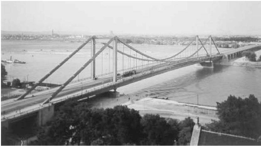
Fig. 18.2 The new bridge was opened in 1937, and replaced the old truss bridge. ( www.reichsbruecke.net/geschichte_e.php )
