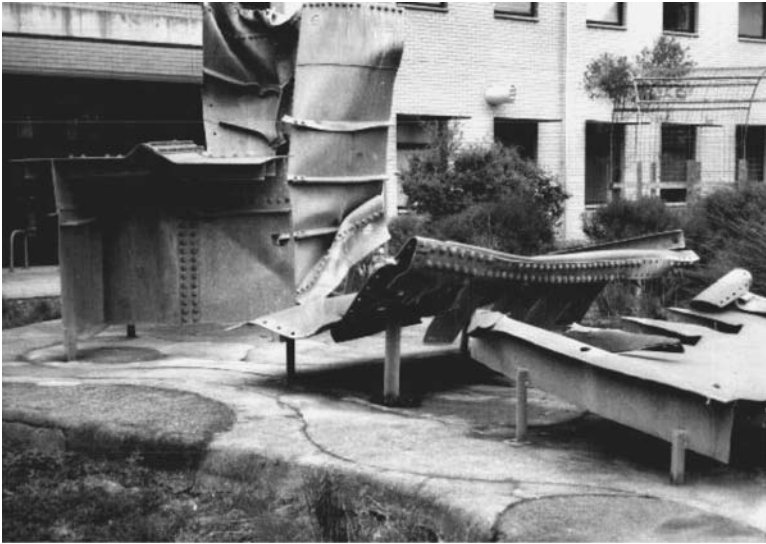
Fig. 15.20 Some removed and saved parts from the collapsed West Gate Bridge at Monash University in Melbourne, Australia. (With kind permission of Bo Edlund)
