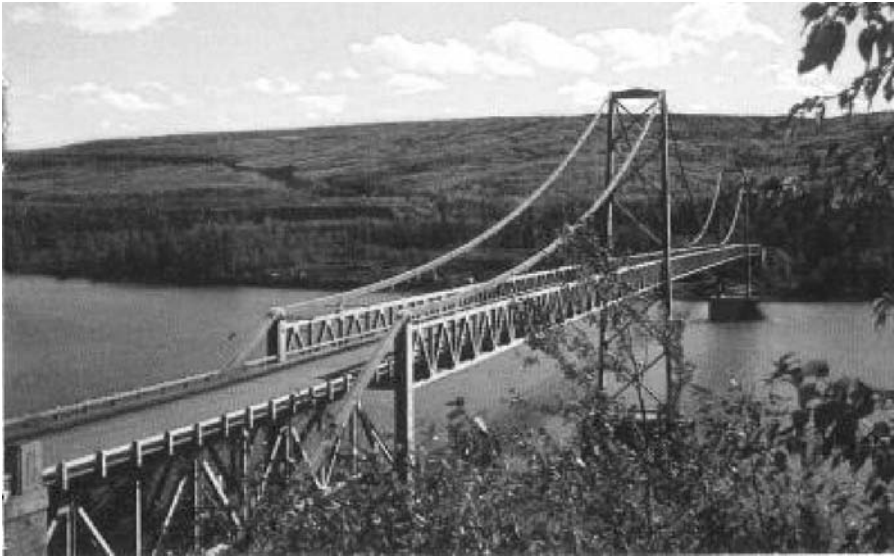
Fig. 8.4 A scenic view of the Peace River Bridge (photo taken 1950). Note the upstream sloping side of the tower piers, not only built because of increased stability in the rapid-flowing waters, but – most probably – primarily for the reduction of ice loads during winter. A nearby temporary timber bridge had in fact been damaged by ice pressure in 1942. ( www.explorenorth.com/library/akhwy/peacriverbridge.html )
