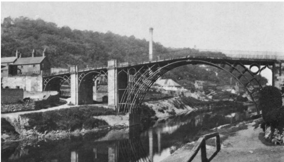
Fig. 1.1 The famous Ironbridge over the river Severn at Coalbrookdale, which was built in 1779, and is still standing intact today. (Cornell: Byggnadstekniken – metoder och idéer genom tiderna)
