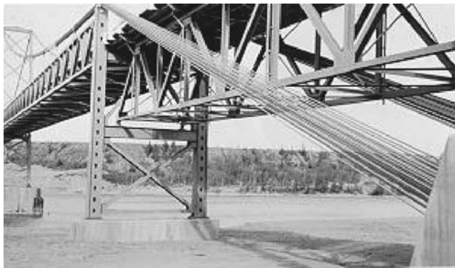
Fig. 8.8 From the cable bent down to the anchorage the strands are splayed, i.e. separated apart in order to provide necessary room for each strand to be safely and securely anchored to the gravity block. ( www.inventionfactory.com/history/RHAbri/term/ )
