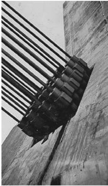
Fig. 8.9 A safe and strong anchorage of all 24 individual strands of the main cable into the gravity block. ( www.inventionfactory.com/history/RHAbbridg/term/ )
