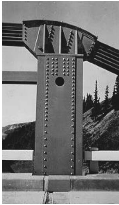
Fig. 8.7 The splay saddle on top of the cable bent. ( www.inventionfactory.com/history/RHAbri/term/ )
