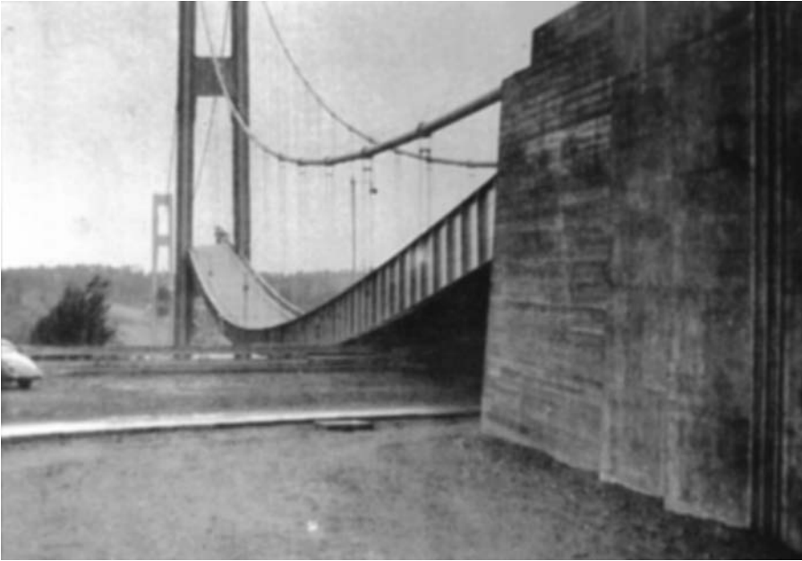
Fig. 7.7 The deflected side span on the east side, at the time of the collapse of the main span. (University of Washington Libraries, Special Collections, UW 27459z)
