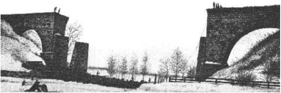
Fig. 2.4 The day after the collapse. The extra brick pier that is seen close to the left-hand abutment is from the earlier wooden bridge at this site. ( http://home.alltel.net/arhf/bridge.htm )
