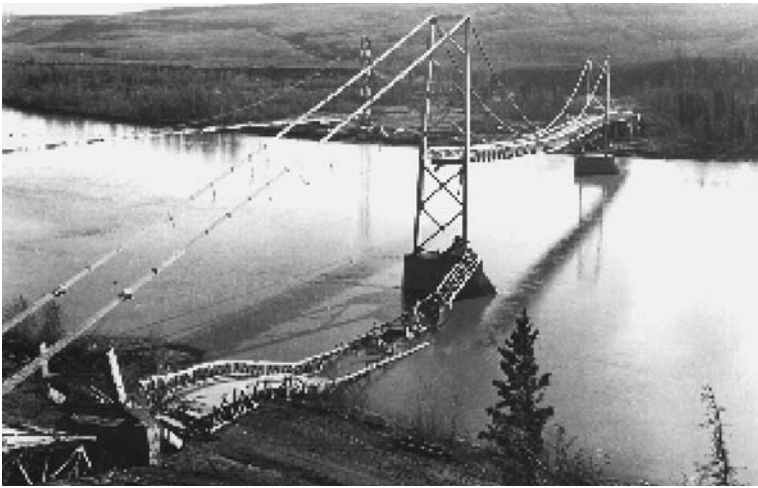
Fig. 8.11 The collapsed Peace River Bridge. ( http://collections.ic.gc.ca/north_peace/transport/02.07.html )
