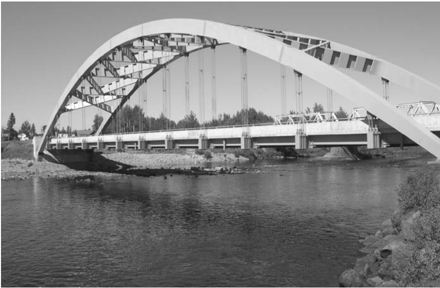
Fig. 20.17 The rehabilitated Aubrey Cosens Bridge at Latchford, September 2007 (with kind permission of Cameron Bevers, photographer and copyright holder).
