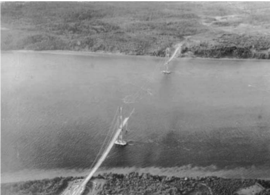
Fig. 7.8 The collapsed Tacoma Narrows Bridge – aerial view looking west, a rather sad and dreary sight. (University of Washington Libraries, Special Collections, UW 26818z)
