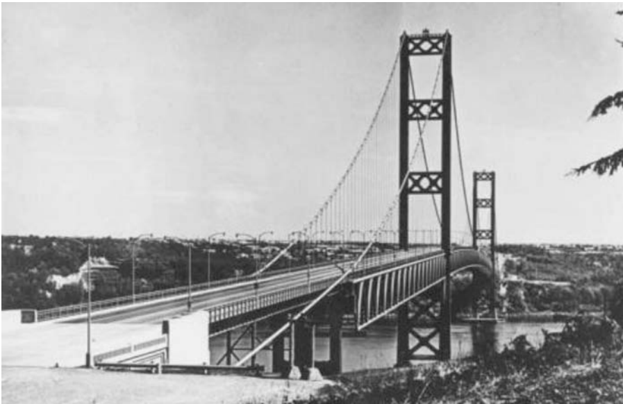
Fig. 7.17 The current Tacoma Narrows Bridge. (University of Washington Libraries, Special Collections, UW 7091)
