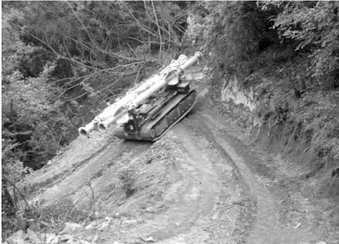
Fig. 27.20 Tower member transportation by tracked vehicles
