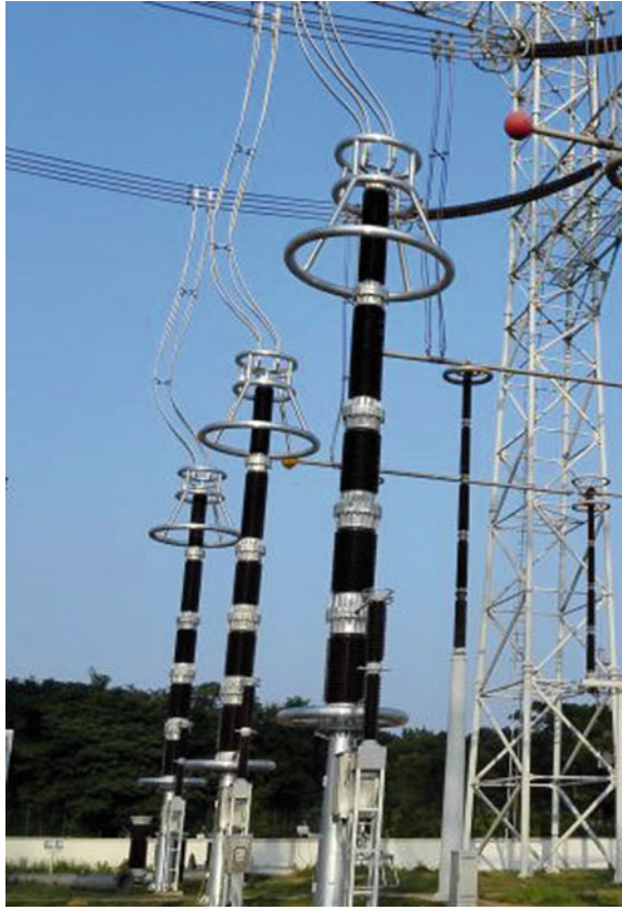
Fig. 11.13 Samples of UHVAC switch controllable arrester with controllable ratio of 15%
