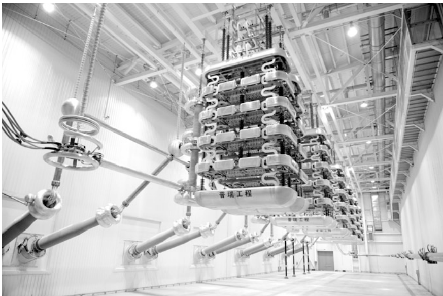
Fig. 20.2 Structure of UHV converter valve tower
