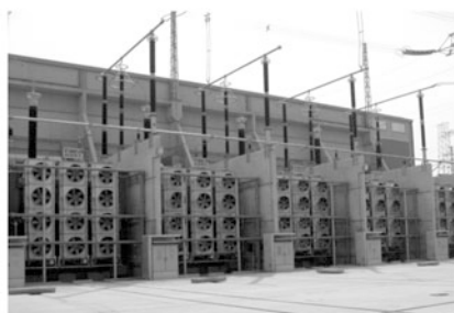
(b) Installed converter transformer
