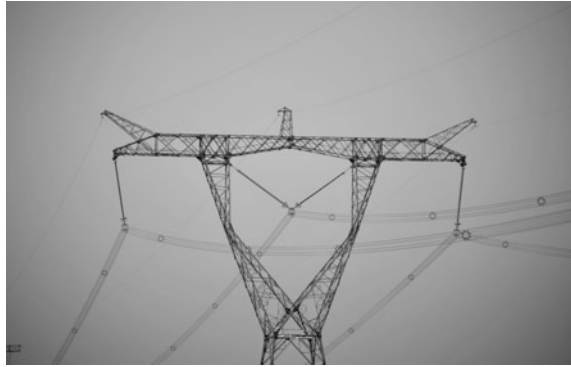
Fig. 8.33 Diagram of tower head of the tower in the incoming line section of China's UHVAC demonstration line
