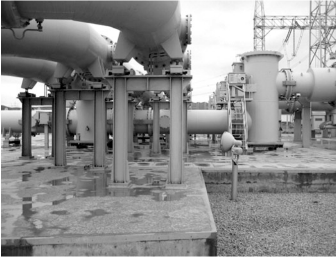
Fig. 25.21 Photo of slab raft foundation
