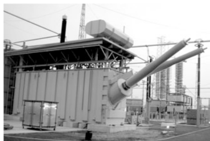
(a) Converter transformer to be installed
