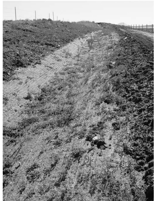
FIGURE 13.2 Synthetic blanket in ditch.
