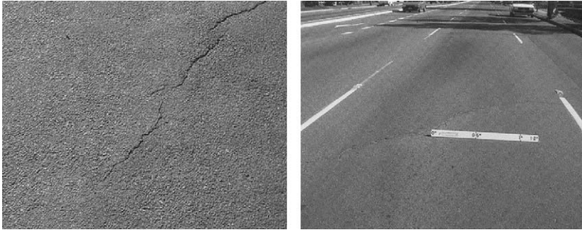
FIGURE 19.14 Diagonal cracks in flexible pavements (Source: Austroads, 1987).
