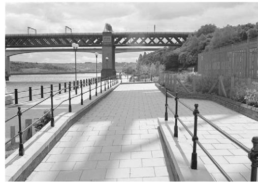
FIGURE 10.5 Footpath surfaced with concrete paving flags.
