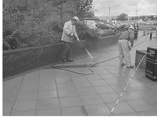
FIGURE 10.9 Cleaning and sealing concrete paving flags.
