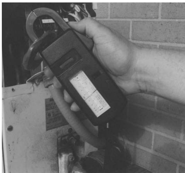
Figure 1-24 Scale divider used with clamp-on ammeter. The ammeter indicates a value of 3.25 amperes. If the scale divider has a ratio of 10:1, the actual current is 0.325 amp.
