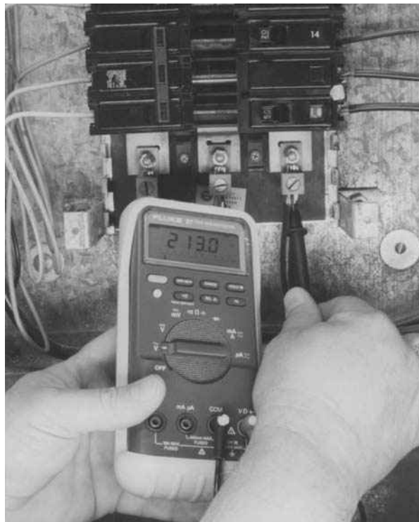
Figure 1-6 A voltmeter can be connected directly to a power source.
