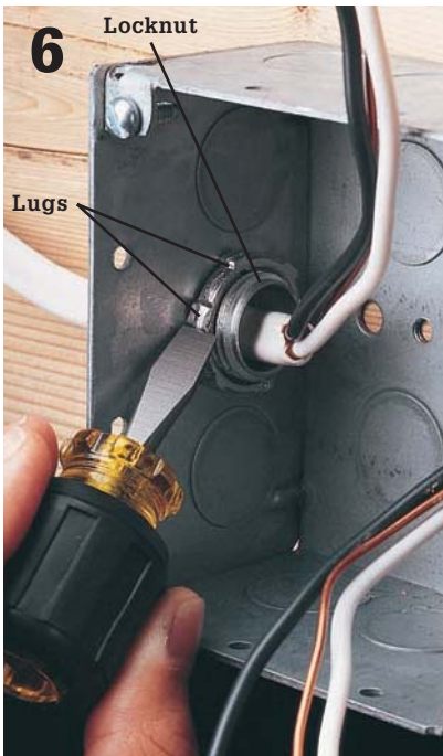
6 Tighten the locknuts by pushing against the lugs with the blade of a screwdriver.
