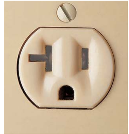
20 amps, 120 volts. This three-slot grounded receptacle features a special T-shaped slot. It is installed for use with large appliances or portable tools that require 20 amps of current.
