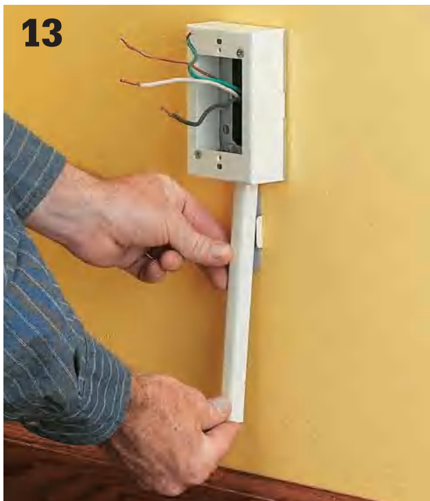
13 At the starter box slide one end of the short piece of raceway into the knockout so that about \frac{1}{8} " extends into the box. Snap the raceway into the clip below the knockout. Repeat this same procedure at the new receptacle box.
