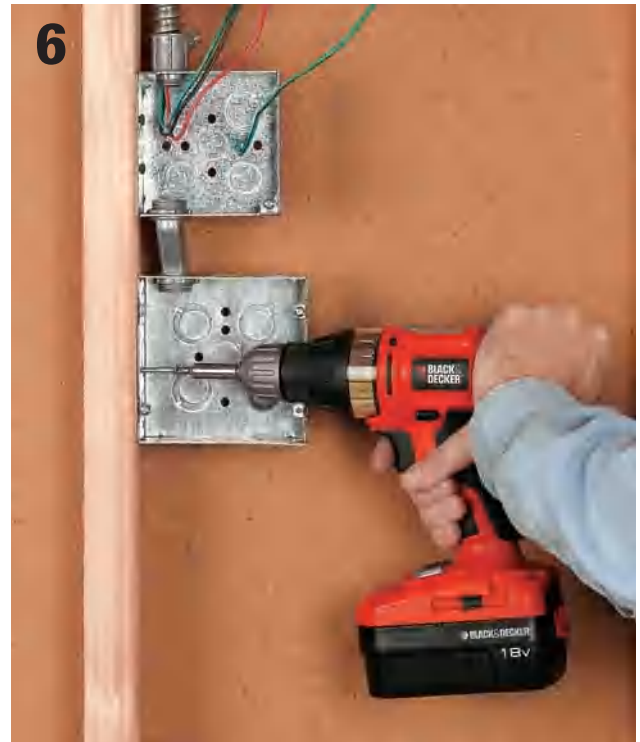
6 Attach a double gang metal junction box to the building's frame beneath the DC disconnect box to enclose the charge controller.
