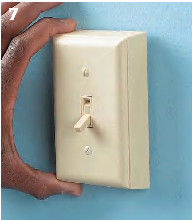
7 Stick the transmitter box to the wall at the desired location. The box should be no more than 50 ft. from the receiver switch (see manufacturer's suggestions). The box should be at the same height (usually 48") as the other switch boxes.
