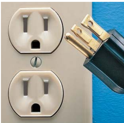
Tamper resistant three-slot receptacles are required by code for new homes. They are usually connected to a standard two-wire cable with ground.
