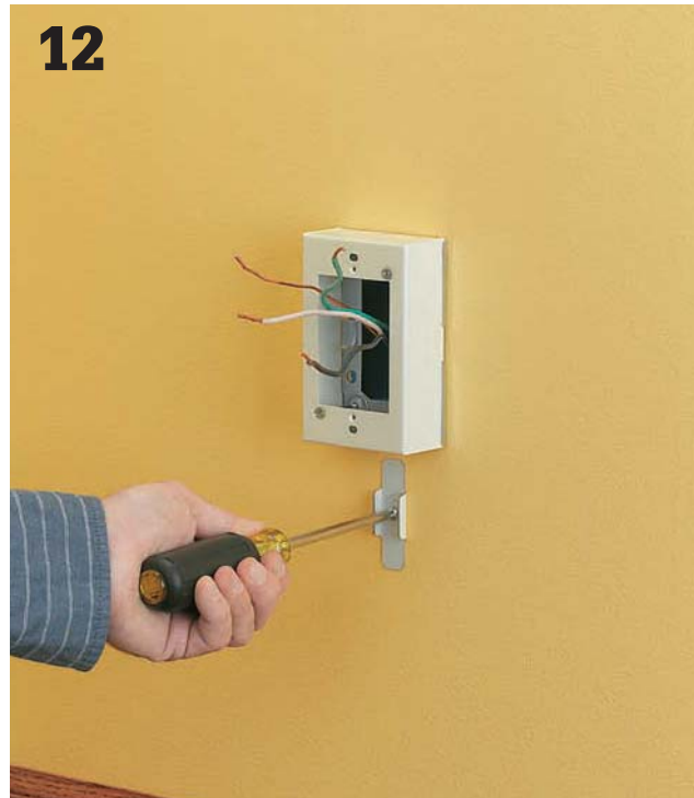
12 Install mounting clips \frac{1}{2} " or so below the knockouts on both the starter box and the new receptacle box. The clips should line up with the knockouts.
