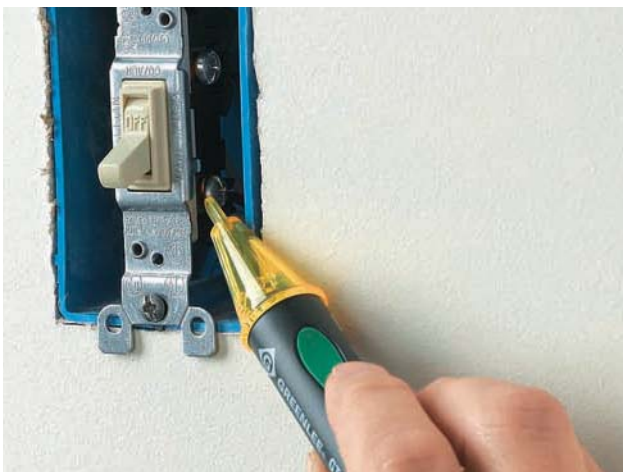
Confirm power is OFF by testing at the outlet, switch, or fixture with a voltage tester.
