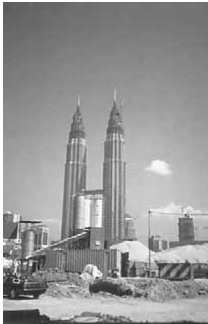
FIGURE 42.5 Towers with batch plant, Malaysia.
