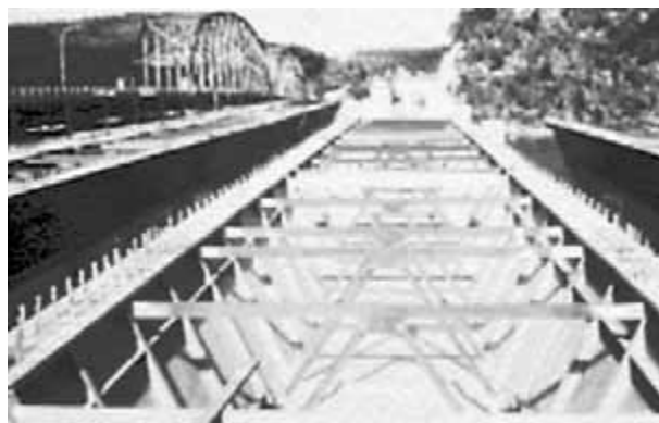
FIGURE 51.1 Composite box girders, Hawkesbury River Bridge, Australia.
