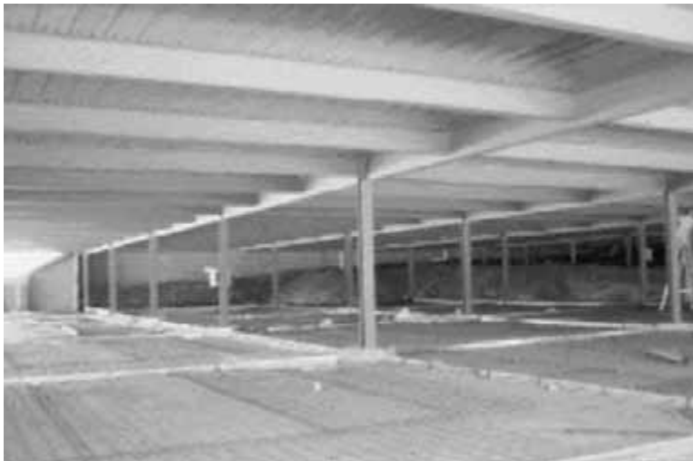
FIGURE 51.3 Composite steel–concrete beams and slabs, car park, Australia.
