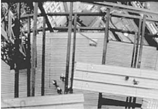
FIGURE 51.2 Composite steel–concrete floors, Grosvenor Place, Sydney.
