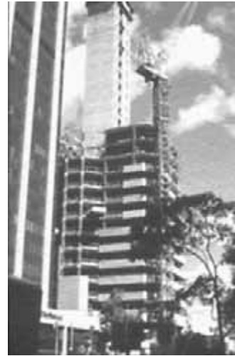
FIGURE 51.5 Composite construction, Forrest Place, Perth.
