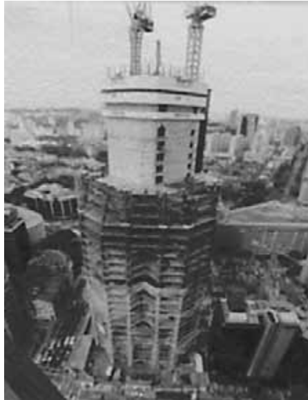
FIGURE 51.6 Composite construction, Republic Plaza, Singapore.
