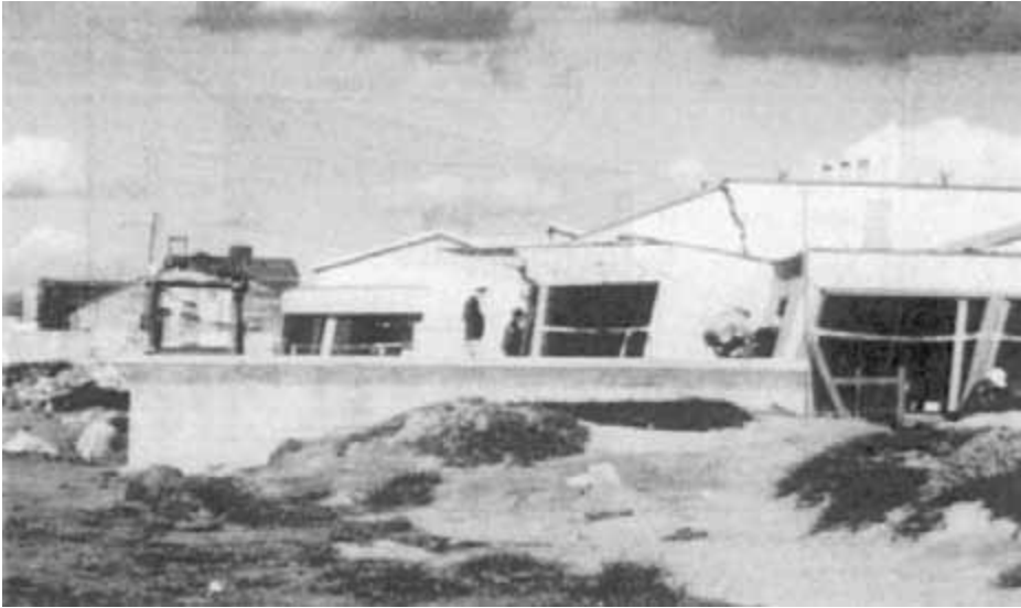
FIGURE 25.7 Liquefaction-induced damage of the Marina Research Facility at Moss Landing, California, caused by the 1989 Loma Prieta earthquake (after Seed, R. B., Dickenson, S. E., Riemer, M. F., Bray, J. D., Sitar, N., Mitchell, J. K., Idriss, I. M., Kayen, R. E., Kropp, A., Harder, L. F., and Power, M. S. 1990. Preliminary Report on the Principal Geotechnical Aspects of the October 17, 1989 Loma Prieta Earthquake. Earthquake Engineering Research Center, Report No. UCB/EERC-90/05, University of California).
