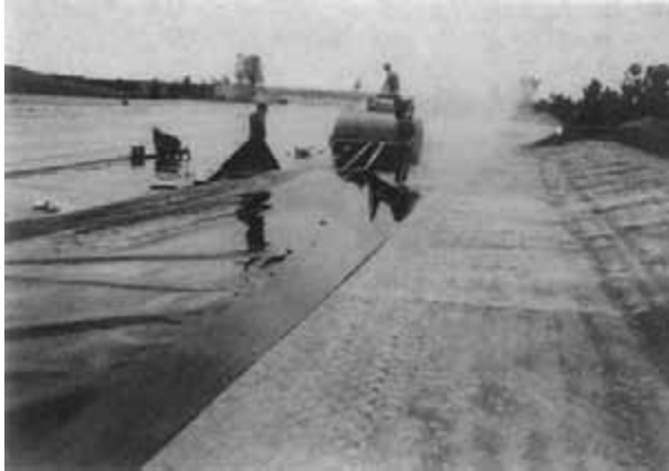
FIGURE 14.3 Geosynthetic fabric liner installation conforms to composite liner federal requirements for MSWLFs at the expansion site of Caldwell Sanitary Landfill. (Source: Caldwell Sanitary Landfill. With permission.)
