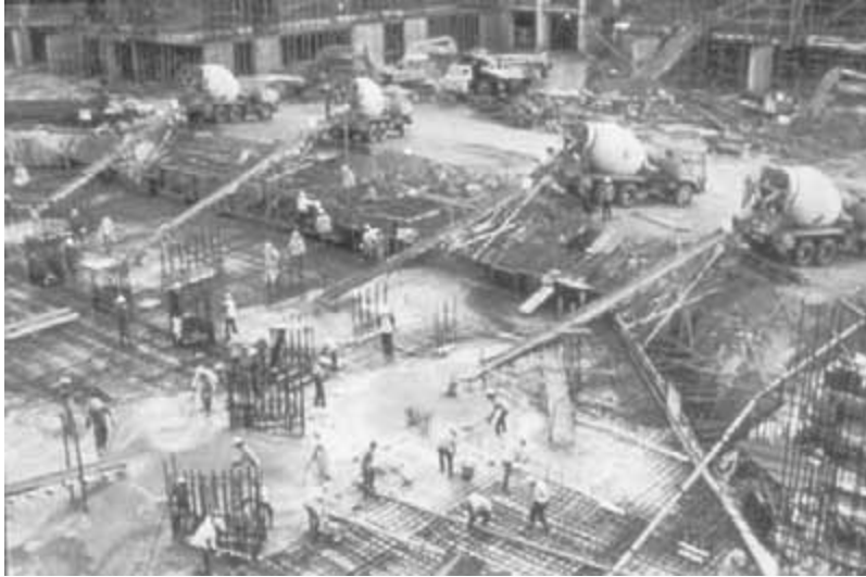
FIGURE 42.3 Concrete placing at Raffles City, Singapore.
