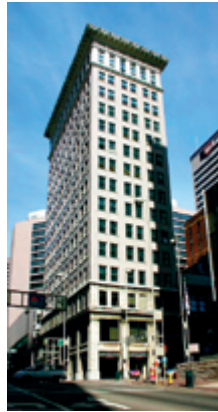
FIGURE 3.1 Ingalls Building, Cincinnati, USA, 1903
