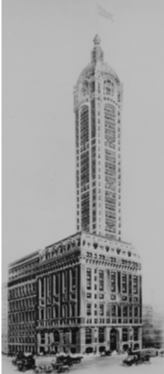
FIGURE 1.4 Singer Building, New York, USA, 1908
