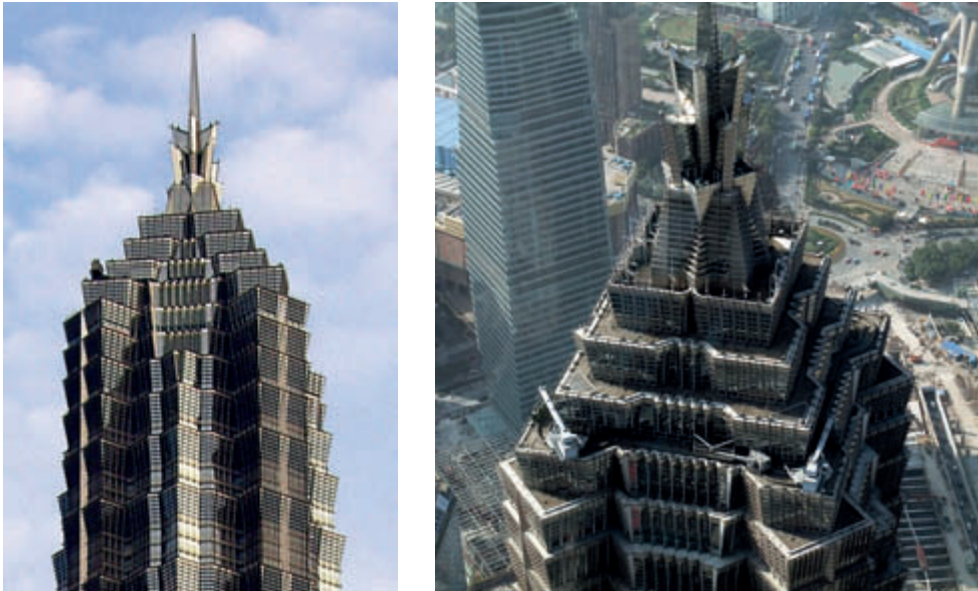
FIGURE 6.8 Jin Mao Building, aerodynamic top (photo on right courtesy of Niels Jakob Darger)
