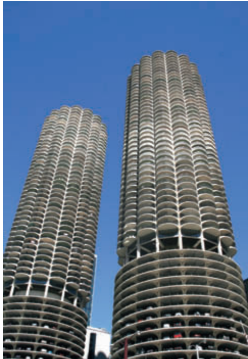
FIGURE 6.2 Marina City Towers, Chicago, USA, 1964 (courtesy of Antony Wood/CTBUH)
