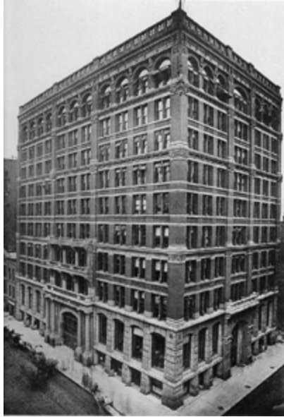
FIGURE 1.2 Home Insurance Building, Chicago, USA, 1885
