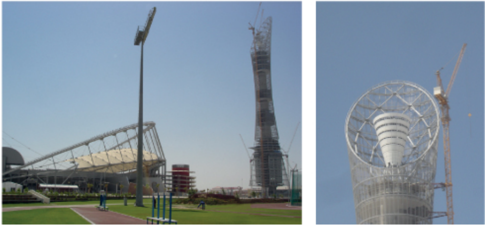
FIGURE 4.8 Aspire Tower (credit for photos: MIDMAC Contracting Co. WLL)
