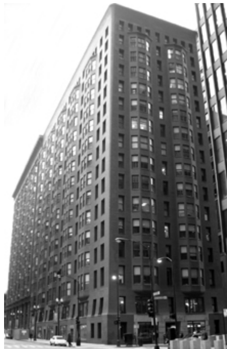
FIGURE 1.1 Monadnock Building, Chicago, USA, 1891
