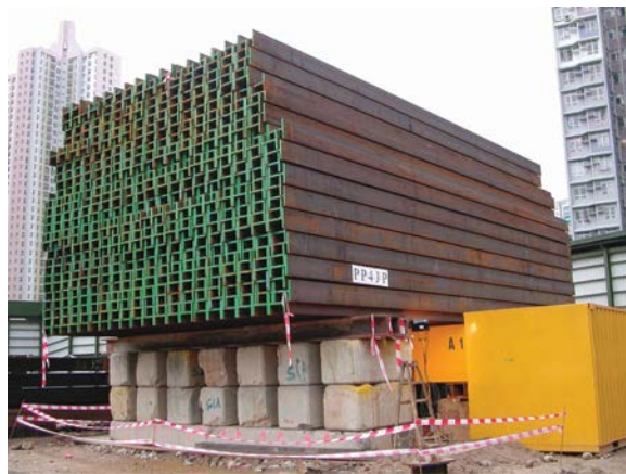
Figure 13.4 Example of use of kentledge for pile load test reaction.
