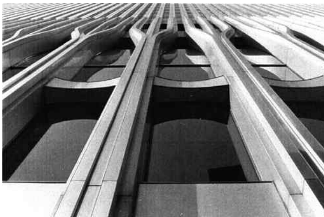
FIGURE 9.49 WTC vertical fenestration: box columns.
