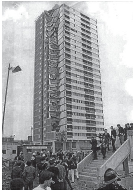
FIGURE 9.35 Ronan Point, a 22-story large precast panel building suffered a partial collapse when a gas explosion demolished a load bearing corner wall.
