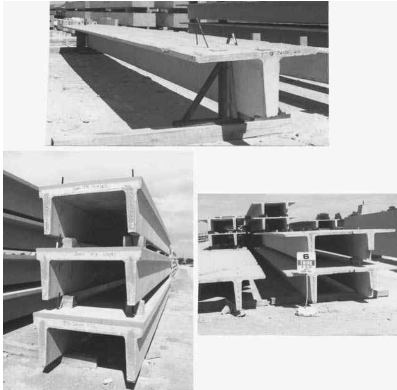
Precast, prestressed concrete sections: (a) single T-section, (b) double T-section, and (c) U-section.
