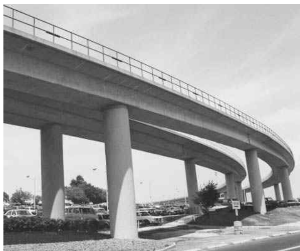
Concrete bridge for the city transit system, Washington, D.C.
