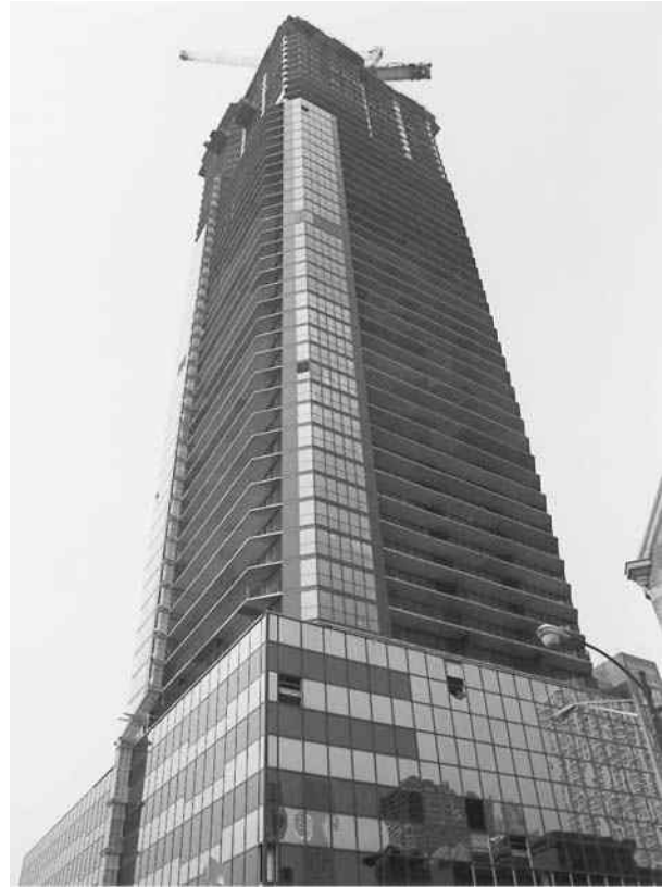
Office building under construction, Chicago, Illinois.
