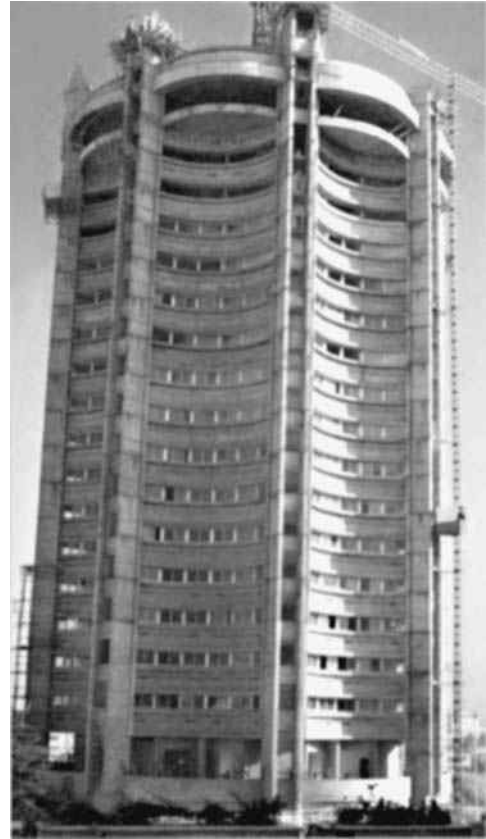
Curved beams in an office building.
