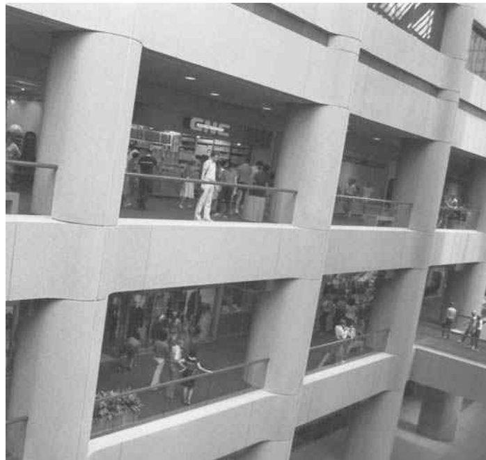
Columns supporting 52-story building, Minneapolis, Minnesota. (Columns are 96 \times 64 in. with round ends.)
