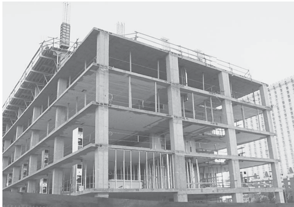
Flat-plate floor system.
