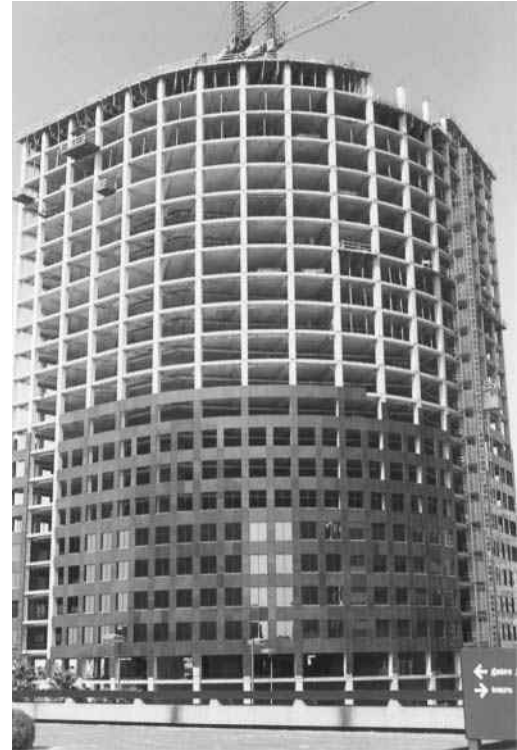
Office building under construction, New Orleans, Louisiana.
