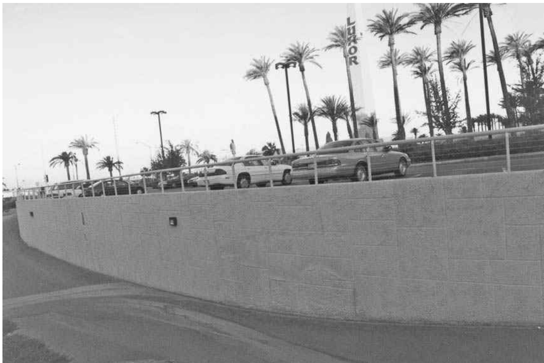
Retaining wall in a parking area.
