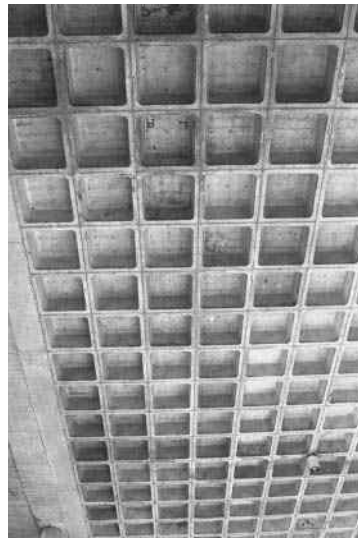
Waffle slab (looking upward).
