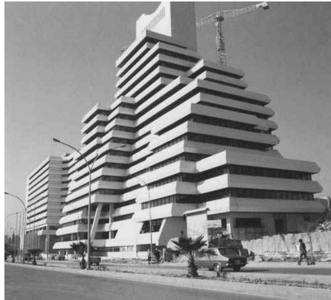
Reinforced concrete office building, Amman, Jordan.
