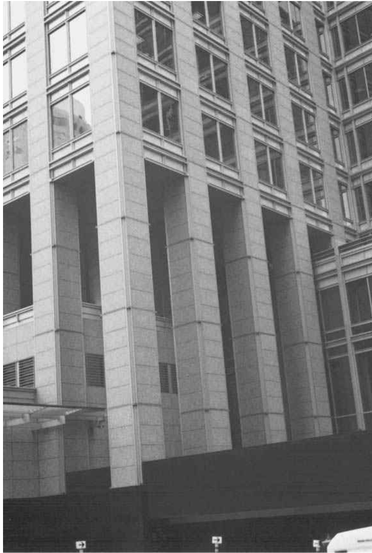
Long columns in an office building
