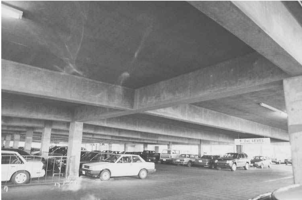
Slab on beams.
