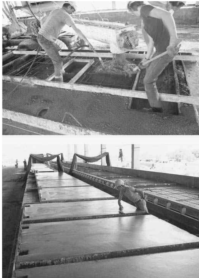
Casting and finishing precast concrete wall panels.
