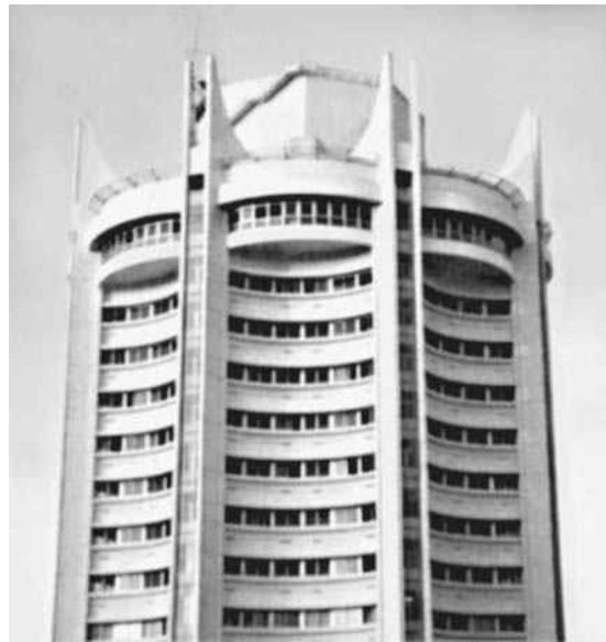
Circular beams in an office building.
