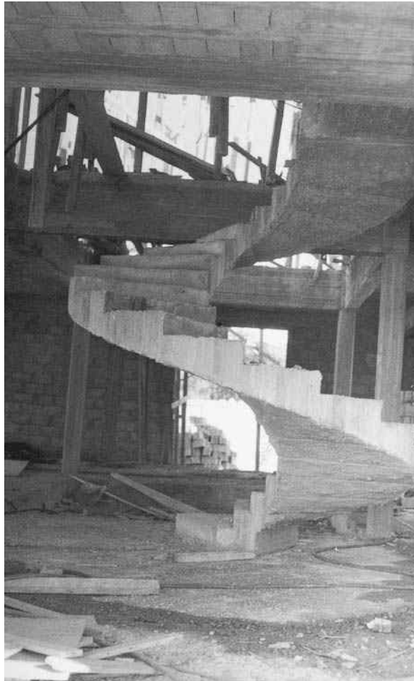
Reinforced concrete helical staircase.
