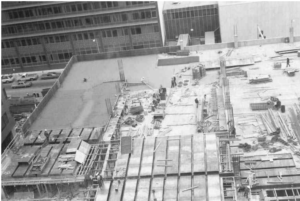
Rectangular steel pans used in one-way ribbed slab construction.
