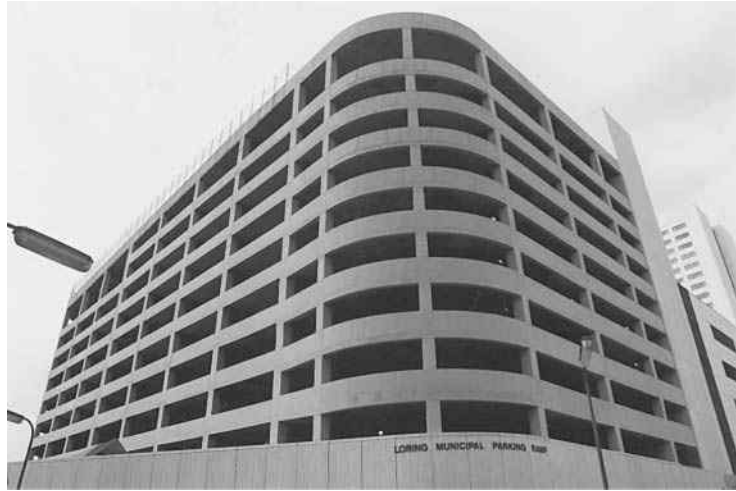
Reinforced concrete parking structure, Minneapolis, Minnesota.
