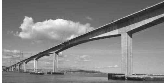
Benicia-Martinez Bridge, California.
