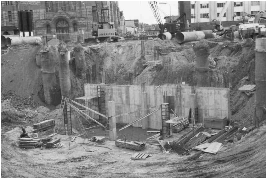
Wall and column footings, partly covered.
