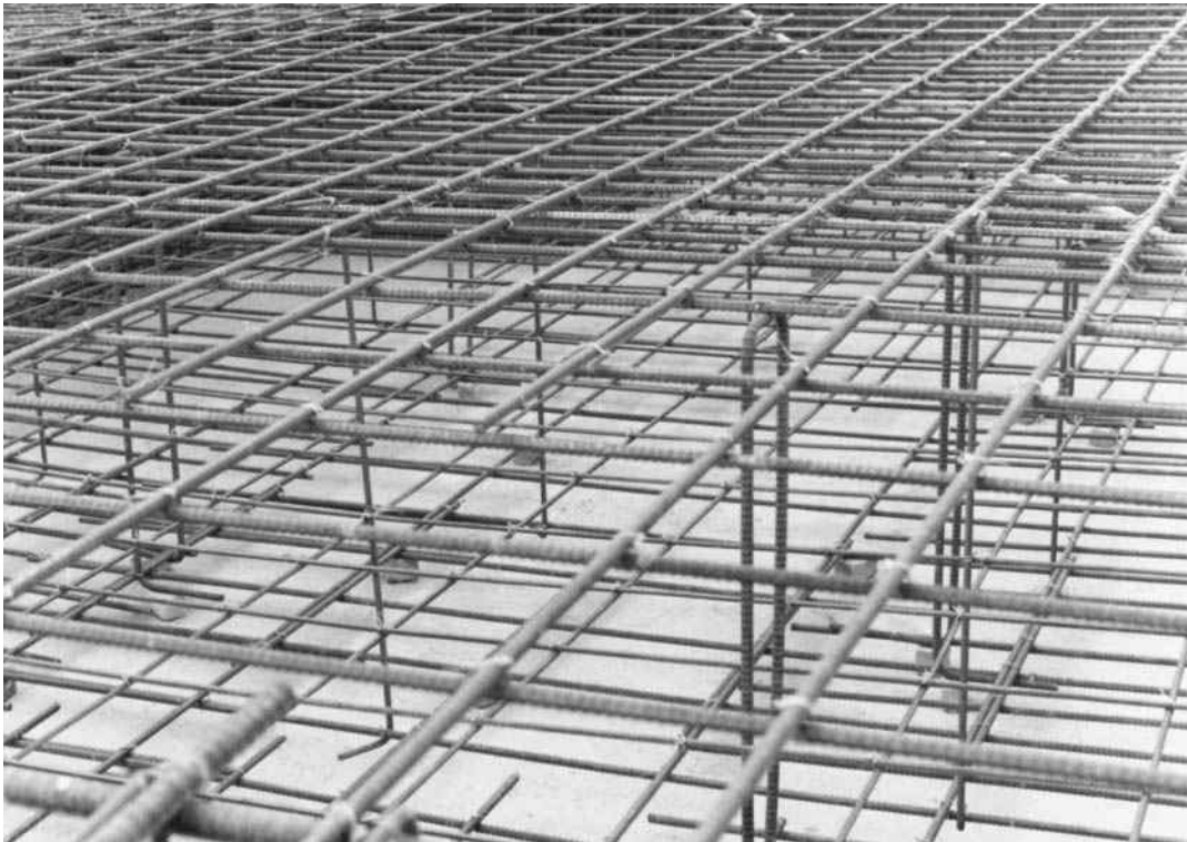
Reinforcing rebars placed in two layers in a raft foundation.
