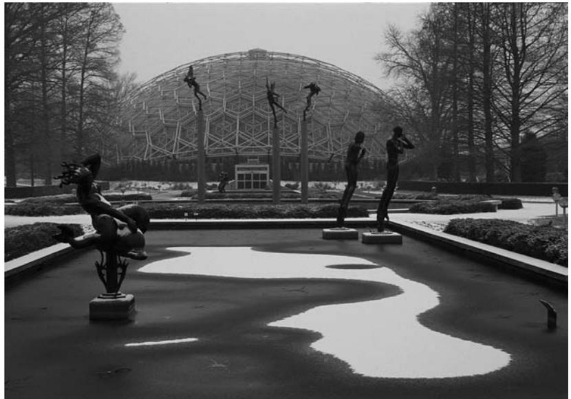
FIG. 4.6 Geodesic Dome Climatron Showing Glass-and-Aluminum Geodesic Design Missouri Botanical Garden, St. Louis, Missouri
