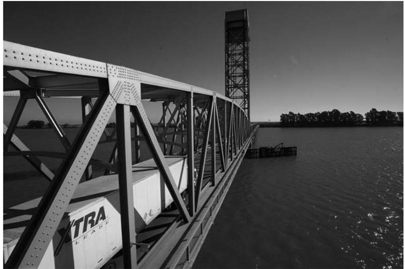
**FIG. 4.8** Truss Bridge with Bolted Connections Rio Vista Bridge
