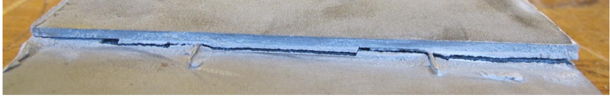
Figure 31.3: Connection 1 – side 1 – direction x+ – delamination of adhesive layer 2
