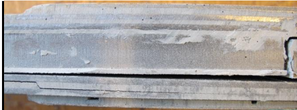
Figure 31.20: Connection 2 – direction y- – end of third lap and middle part
