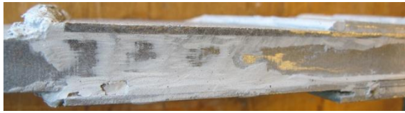
Figure 31.18: Connection 2 – direction y- – end of first lap
