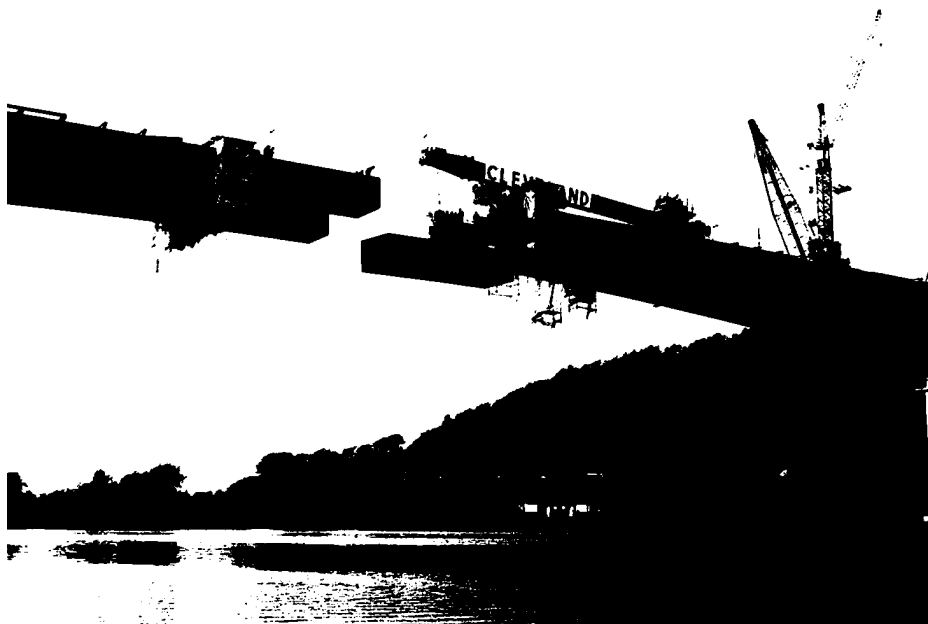
Fig. 33.14 A purpose-made lifting beam for cantilever erection
