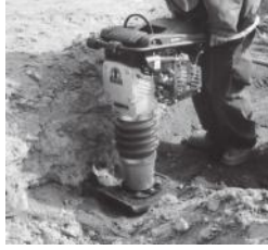
(a) Hand-operated vibratory tamper
