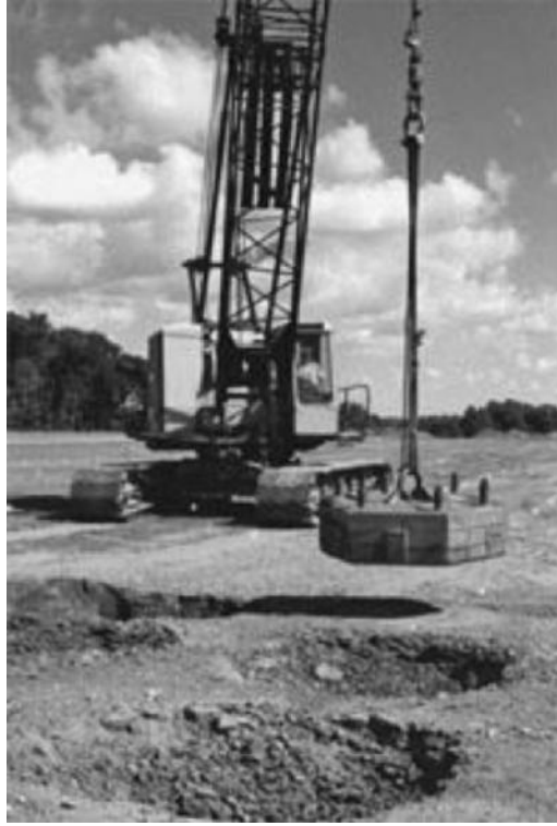
FIGURE 5.9 Dynamic compaction. (Photo courtesy of Terra Systems, Inc.)
