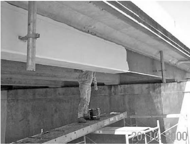
FIGURE 5.15 Application of finishing coat (Muddy Creek Bridge, West Virginia).
