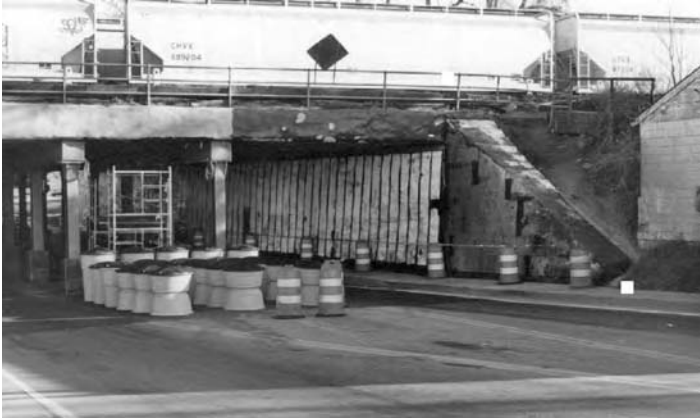
FIGURE 5.5 View of the wing wall and concrete girder being restored with GFRP fabric and the abutment wall with moisture-trap channels (East Street Viaduct, West Virginia).
