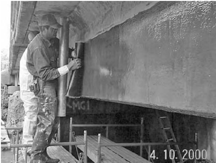
FIGURE 5.12 Wrapping of the beam side with CFRP fabrics (Muddy Creek Bridge, West Virginia).
