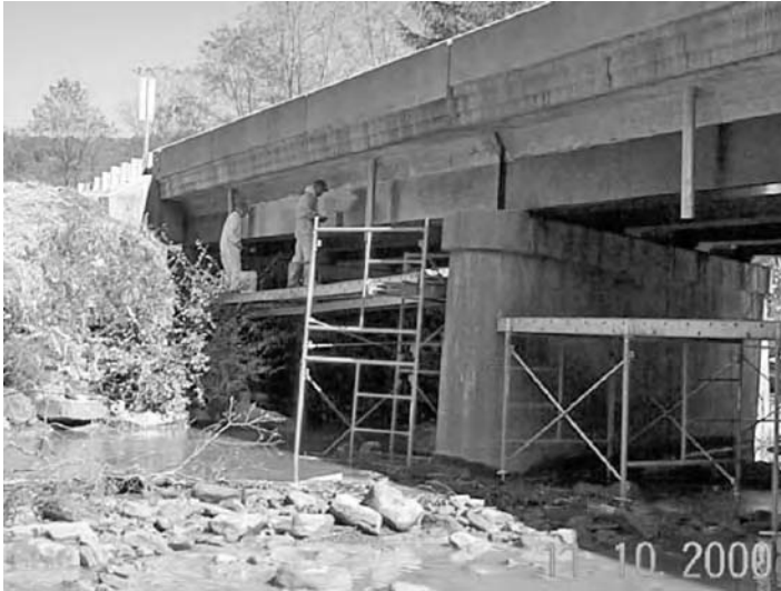
FIGURE 5.11 Primer application on Muddy Creek Bridge (West Virginia) beams before wrapping.
