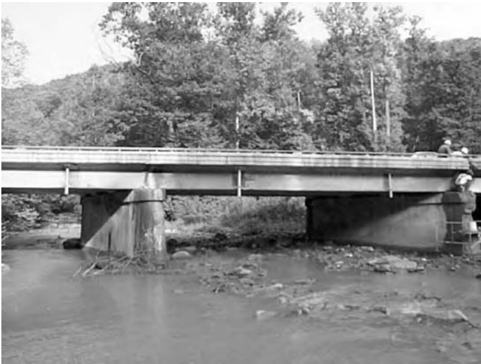
FIGURE 5.10 Muddy Creek Bridge (West Virginia) before wrapping.
