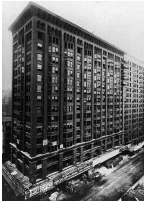
FIGURE 8.5 Monadock Building, Chicago.
