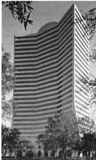
FIGURE 3.17 A 28-story haunch girder building, Houston, Texas. (a) Typical floor plan and (b) photograph. (Structural engineers, Walter P. Moore and Associates.)
