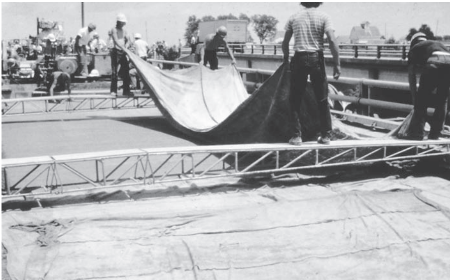
FIGURE 7.28 Curing concrete with impervious fabrics.
