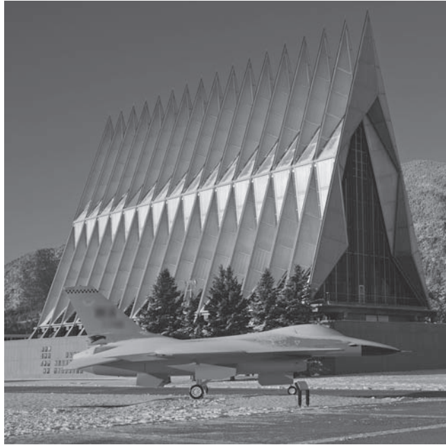
FIGURE 1.19 An example of artist-engineer collaboration in an engineering project: Air Force Academy, Colorado Springs, Colorado.
