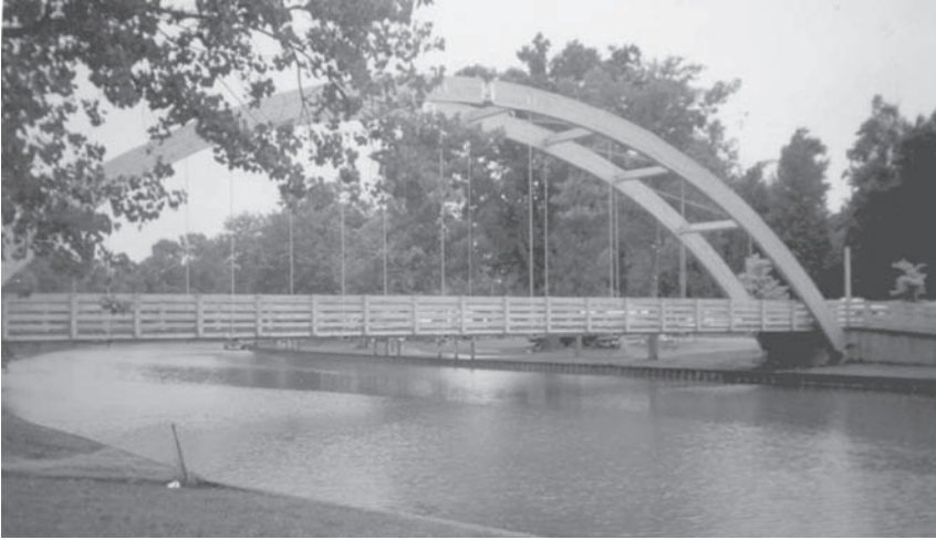
FIGURE 10.7 An arch bridge made of structural glued laminated timber (glulam). (Courtesy of the American Institute of Timber Construction)
