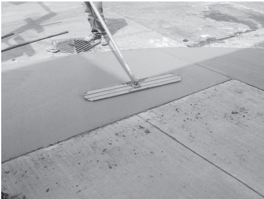
FIGURE 7.19 Finishing concrete manually with a straightedge. (Fotolia/alisonhancock)
