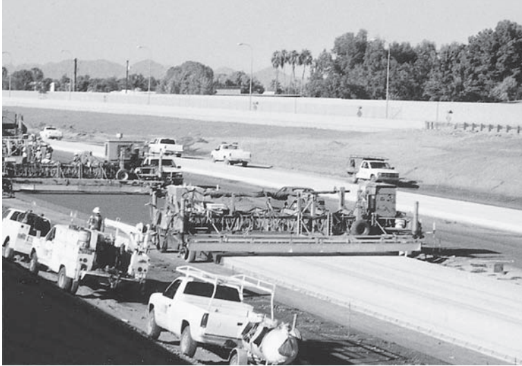
FIGURE 7.31 Curing concrete by machine applying membrane forming compound.
