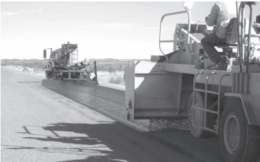
FIGURE 9.9 Applying chip seal (emulsion followed by aggregates) for preserving existing pavement. (Courtesy of FHWA)
