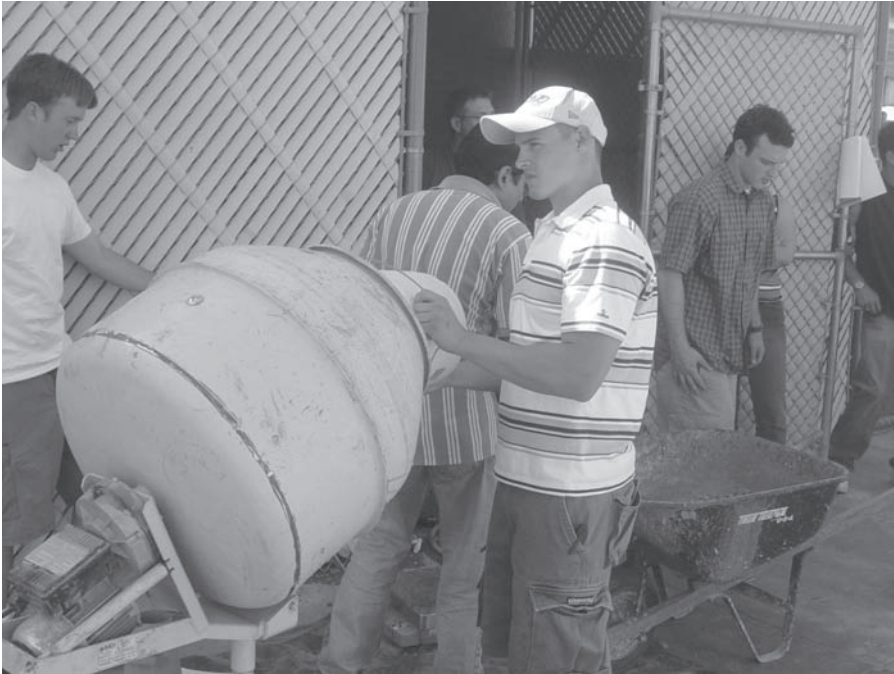
FIGURE A.30 Mixing concrete in a mixer.
