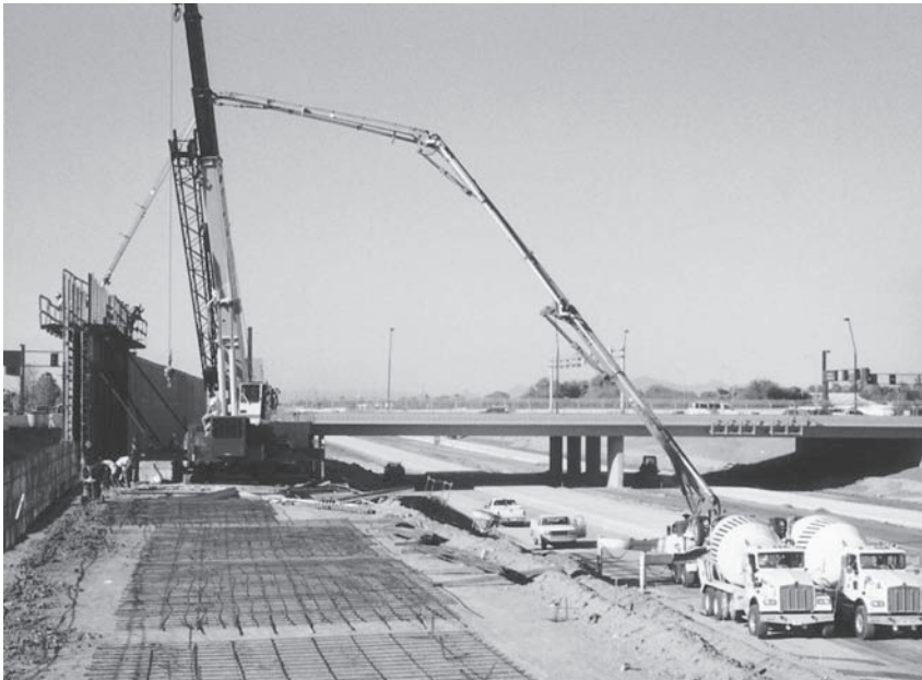
FIGURE 7.12 Pumping concrete in a retaining wall.
