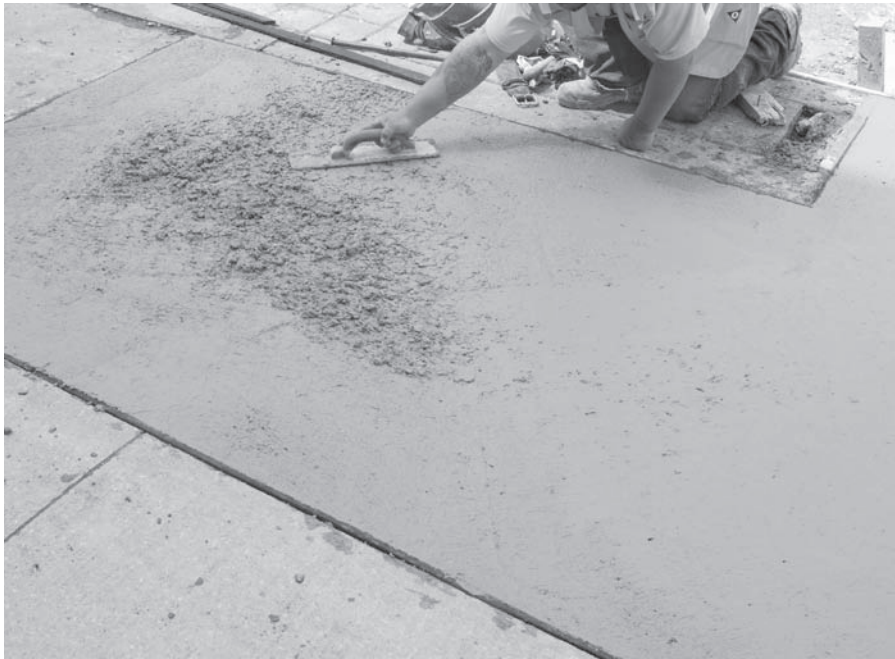
FIGURE 7.18 Finishing concrete with a trowel. (Fotolia/alisonhancock)
