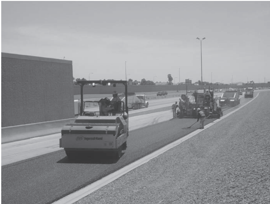
FIGURE 9.6 Compaction of asphalt concrete.
