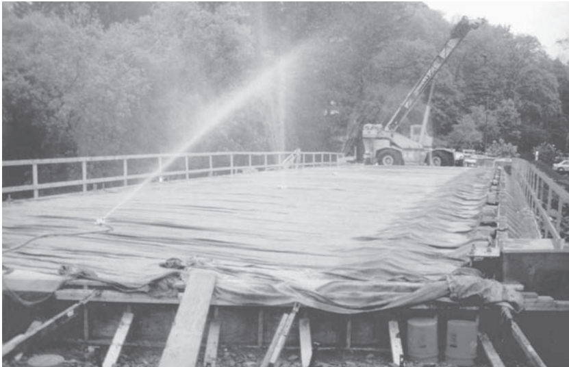
FIGURE 7.27 Curing concrete by wet covering. (Courtesy of FHWA)
