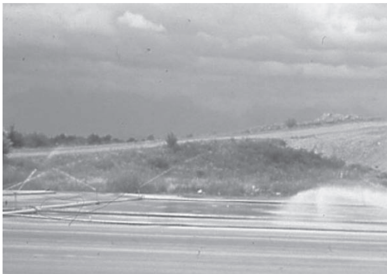
FIGURE 7.25 Curing concrete by spraying. (Courtesy of FHWA)
