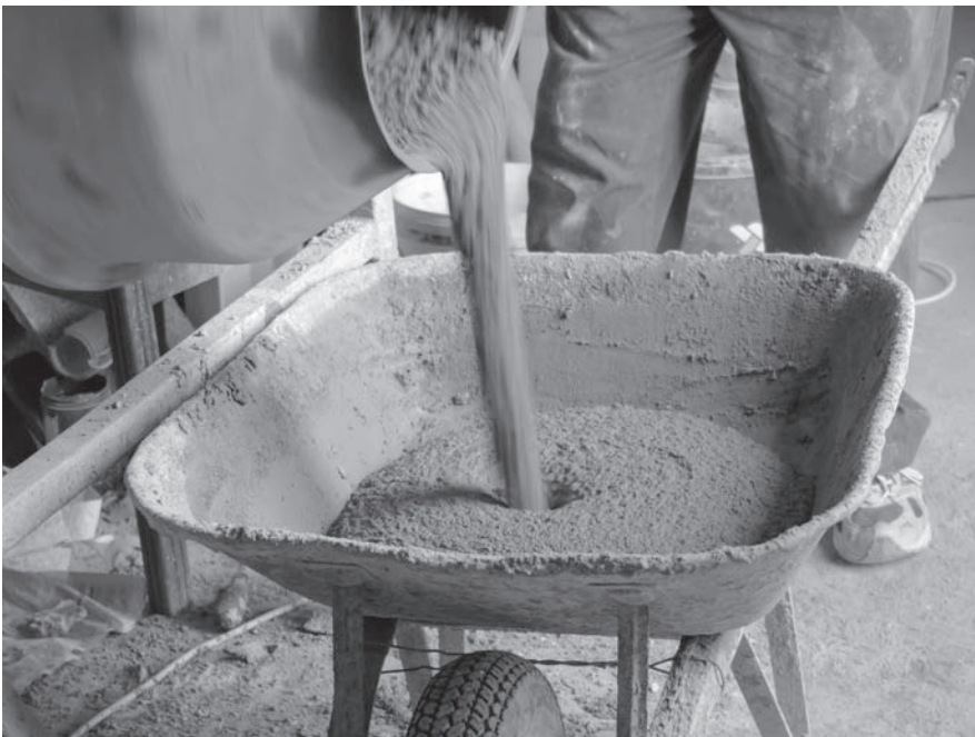
FIGURE 7.7 Loading concrete in a wheelbarrow. (Fotolia/Laure F)
