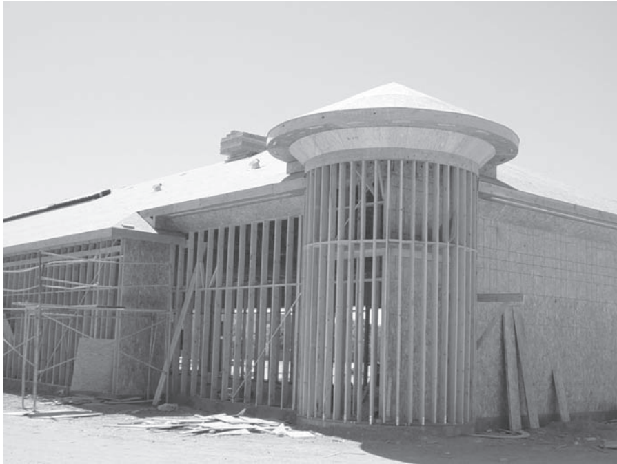
FIGURE 10.1 Wood frame used for building structural support.
