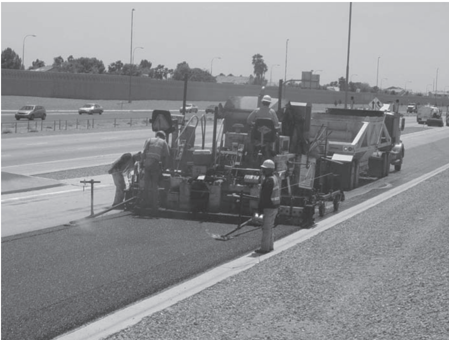
FIGURE 9.5 Placing asphalt concrete used for the surface layer of asphalt pavement.
