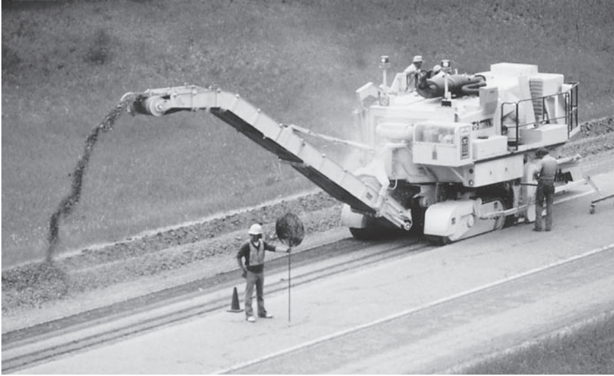
FIGURE 9.41 Milling old pavement.
