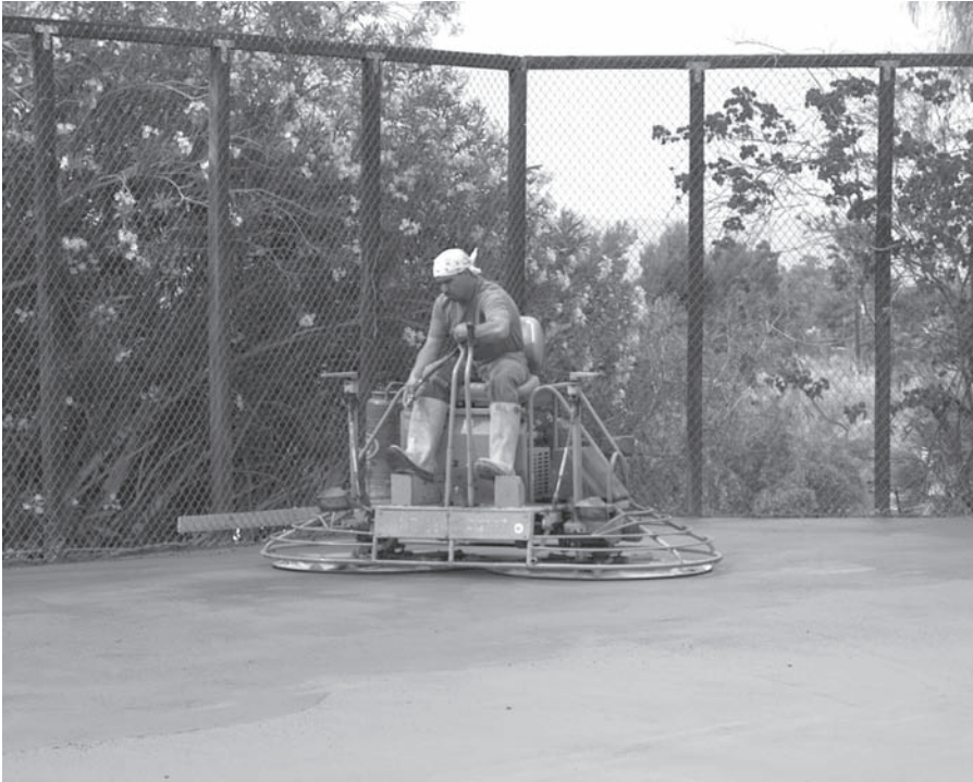
FIGURE 7.20 Finishing concrete with a power float.
