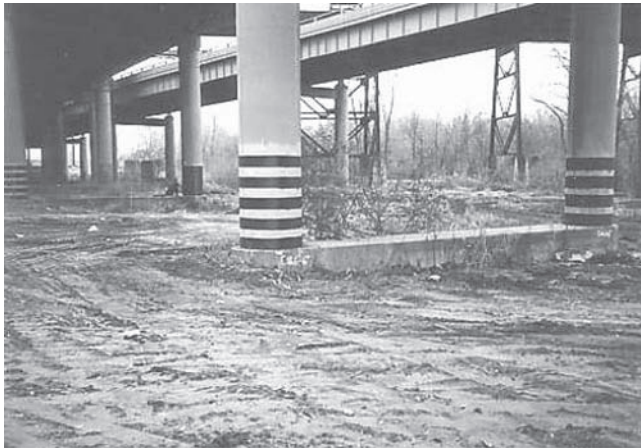
FIGURE 11.11 Wrapping columns of a bridge with FRP composites.
