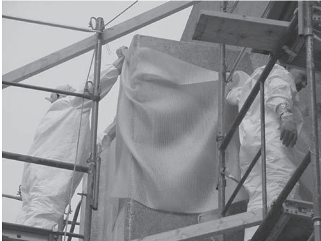
FIGURE 11.10 Wrapping an old structure with glass fiber-reinforced polymer composite. (Courtesy of R.J. Watson)
