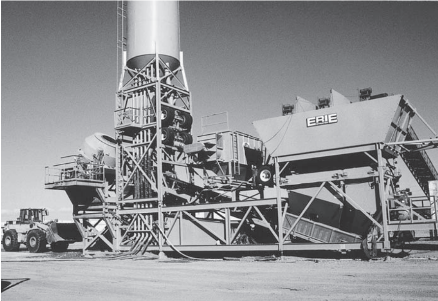
FIGURE 7.6 Mobile batcher mixer at the job site.
