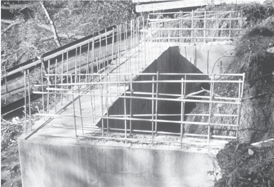
FIGURE 11.1 FRP reinforcing bars used for bridge abutment. (Courtesy of West Virginia University Constructed Facilities Center)
