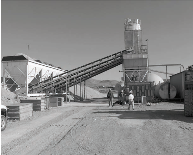
FIGURE 7.5 Concrete ready mix plant.
