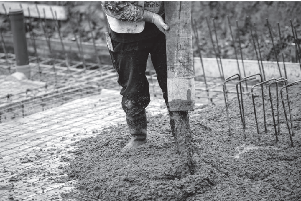
FIGURE 7.9 Placing concrete with Chute. (Fotolia/Hoda Bogdan)
