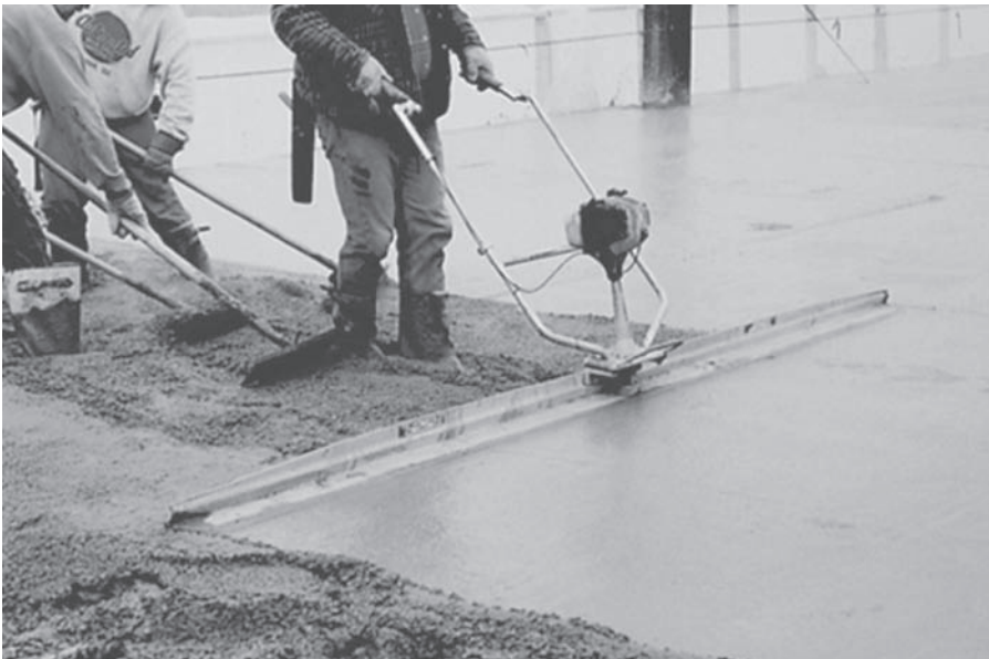
FIGURE 7.21 Finishing concrete with a vibratory screed. (Courtesy of FHWA)
