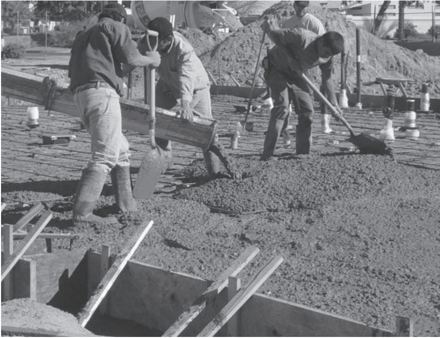
FIGURE 7.8 Placing concrete slab.
