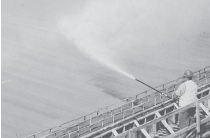
FIGURE 7.26 Curing concrete by fogging. (Courtesy of FHWA)
