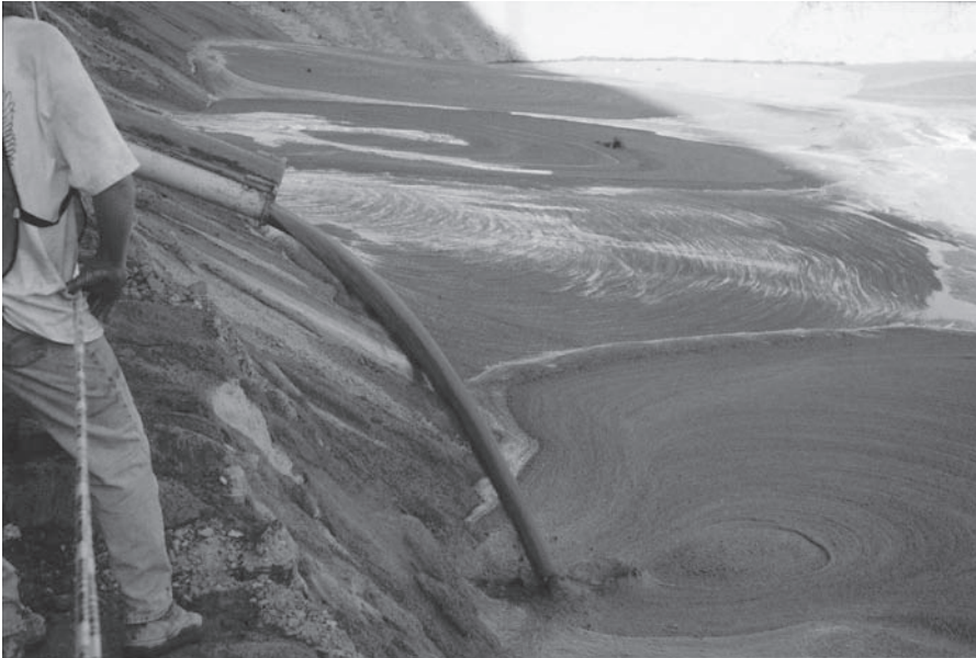
FIGURE 7.45 Filling a sink hole with flowable fill.
