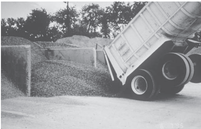
FIGURE 5.20 Aggregate bins used to stockpile aggregates with different sizes.
