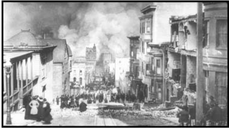
FIGURE 6.2 Fire spread in 1906 San Francisco after the Great Earthquake.
