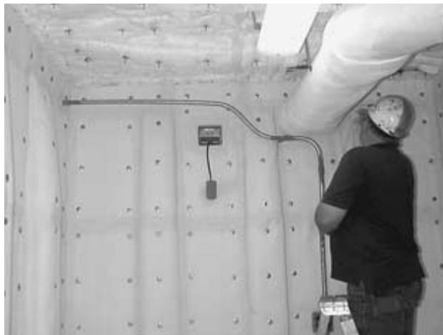
FIGURE 9.50 Fire insulation installation on composite interior spaces of a prototype deckhouse.
