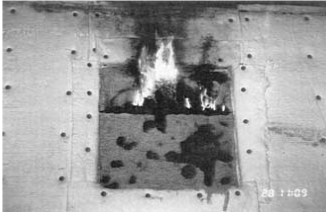
FIGURE 9.29 Intumescent mat bulkhead test (Test 3) at the end of 30-min fire test.
