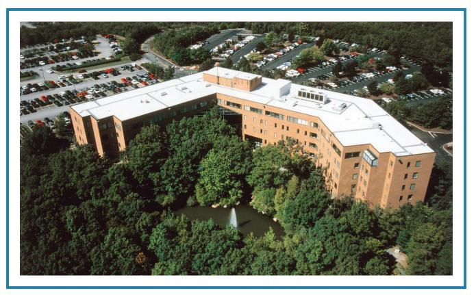
and 81% for low-slope only, when the product is initially installed. (For more information go to www.energystar.gov and click on Roof Products.) It should be noted that durability and maintenance influence reflectance, as the percentage can be reduced by surface weathering and dirt accumulation.
