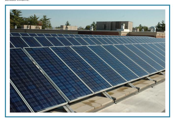
type of PV cells, converting as much as 17% of incoming solar energy into electricity. The main disadvantage of single crystal silicon cells is their production costs; growing large crystals of silicon and then cutting them into thin (0.1–0.3 mm) wafers is slow and expensive.
