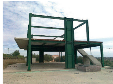
Fig. 7.35. Example of a steel building with steel shear panels
