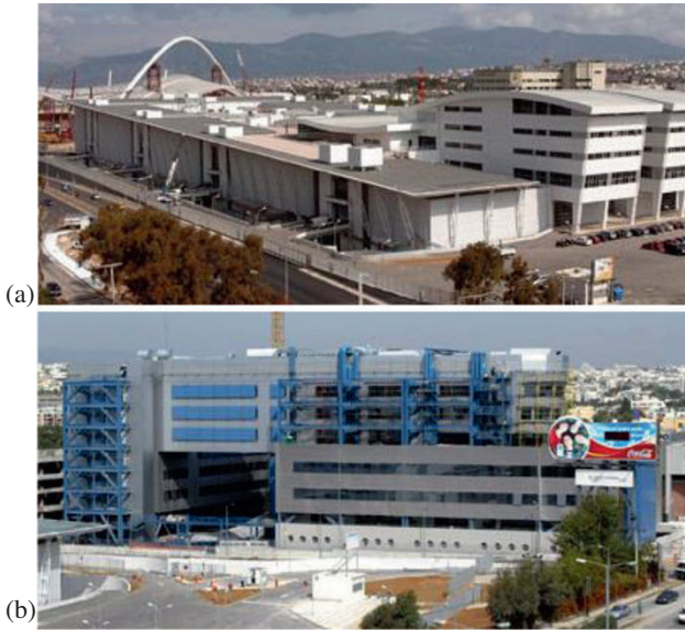
Fig. 7.1. Multi storey steel buildings constructed for the Olympic games of Athens on 2004 (a) International Television Centre and (b) Main Press Centre
