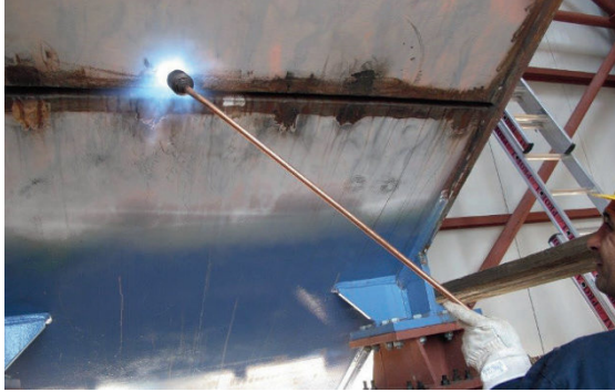
Fig. 8.4. Preheating of a butt weld groove before welding
