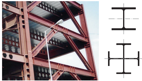
Fig. 7.2. Steel buildings column with crossed double I-section
