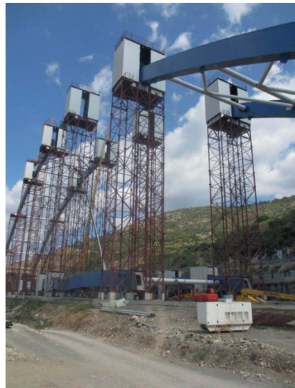
Fig. 8.3. Protection cabins for on-site welding between arch segments of a bridge
