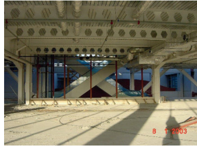
Fig. 7.9. Castellated beams in steel buildings
