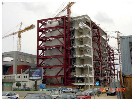
Fig. 7.31. Steel building with eccentric bracings
