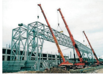
Fig. 8.21. Erection of a pair of plane latticed frames
