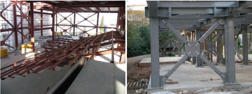
Fig. 7.29. Examples of buildings with concentric bracing systems
