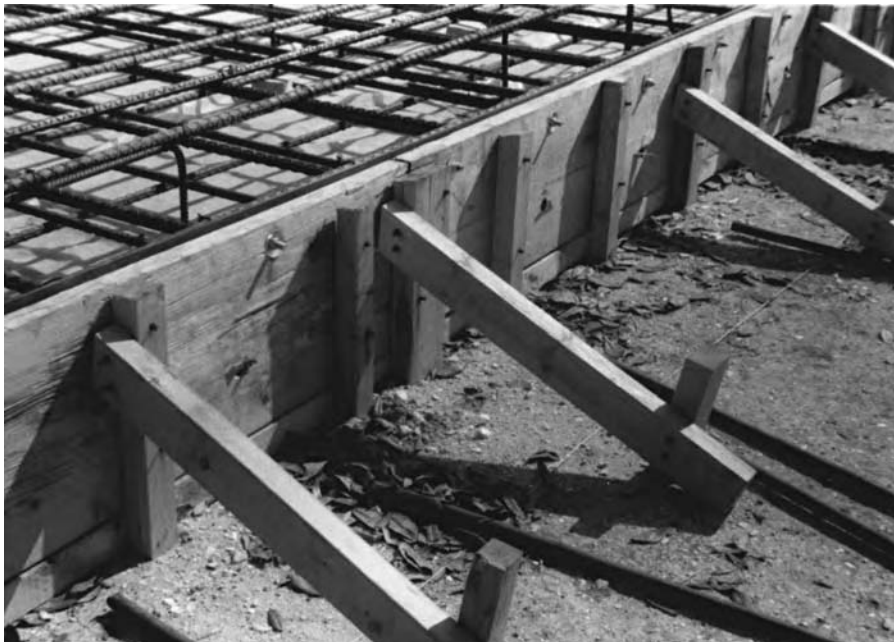
Figure 11.13 Heavily braced timber form
