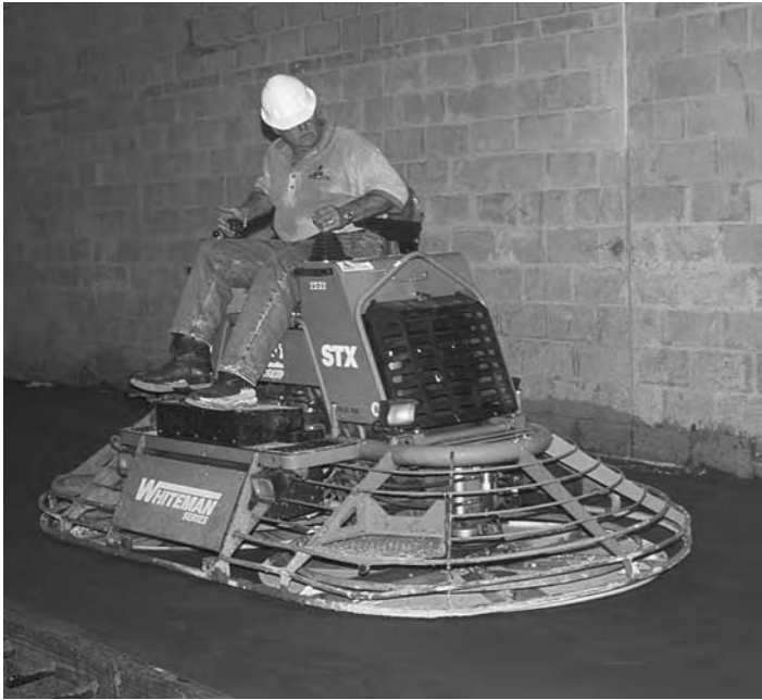
Figure 17.8 Riding trowel machine fitted with float pans
