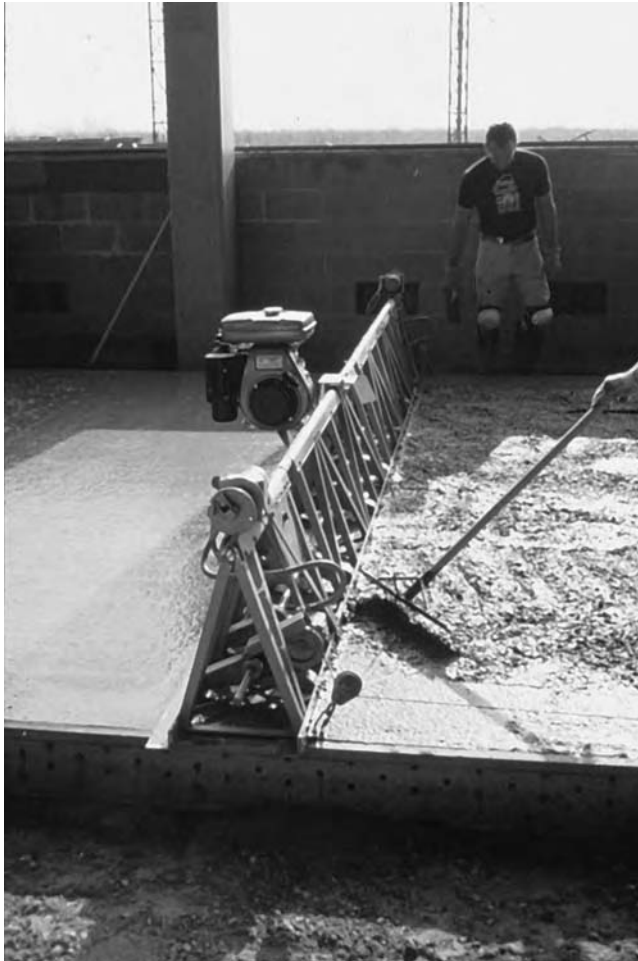
Figure 17.4 Truss-type vibrating screed
