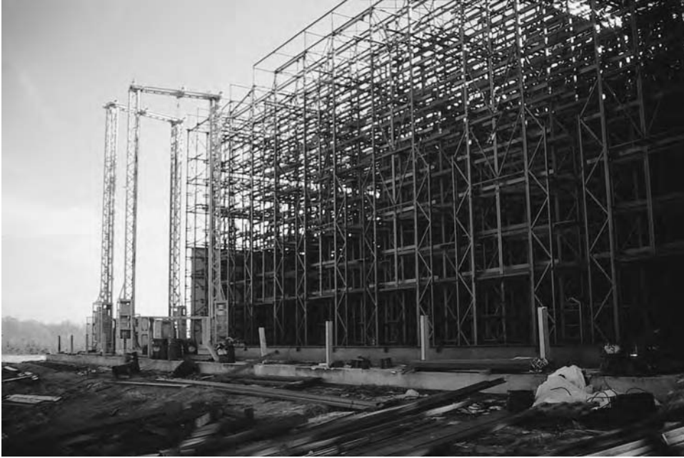
Figure 3.5 A clad-rack (also called rack-supported) warehouse under construction
