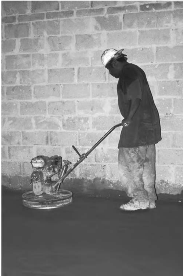
Figure 17.7 This small trowel machine is used at the slab's edge
