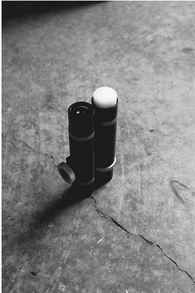
Figure 13.3 Measuring crack width with a 50x microscope
