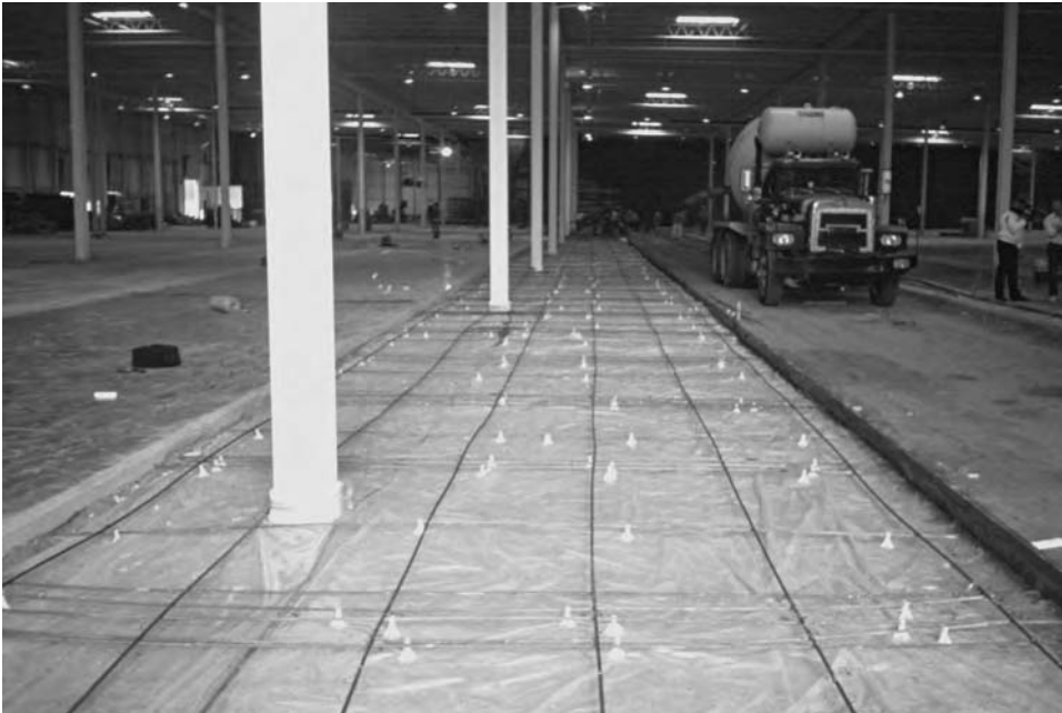
Figure 16.4 One-way post-tensioned floor with unbonded tendons
