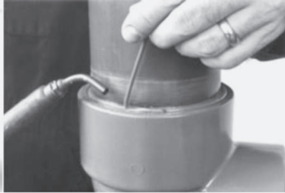
Apply additional weld beads; number of beads depends on pipe size.
