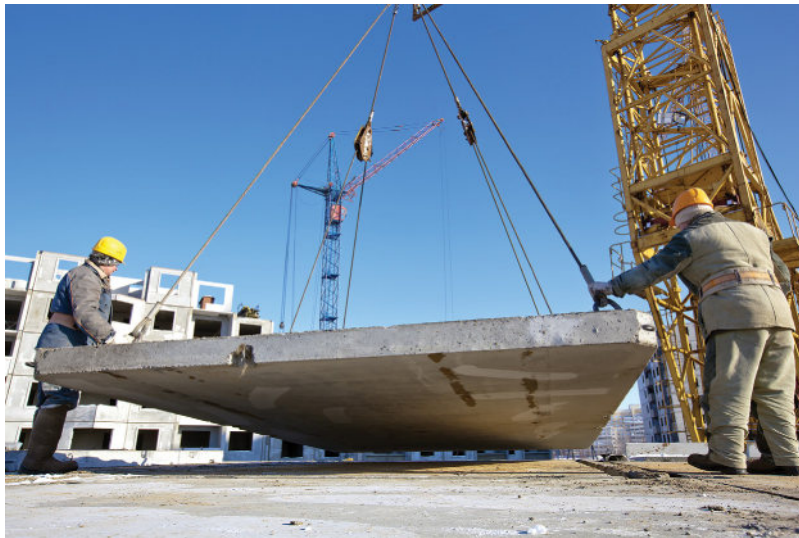
FIGURE 1-1 The concepts of strength of materials are critical in many applications, including this one where workers assure that this concrete element is ready to be lifted into place where it will serve as a critical piece of a multistory structure.
