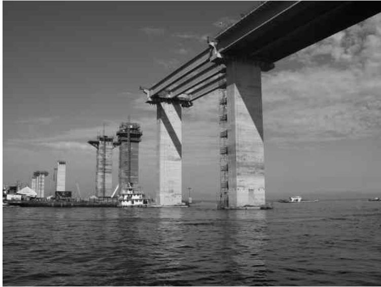
FIGURE 5–1 (See color insert.) A bridge under construction shows vertical supports in place where beam reactions will occur. One can see that the effect on each beam in the completed bridge will vary with respect to position relative to those supports. In this chapter, we will learn to quantify what is happening internally along the length of a loaded beam so that, in a subsequent chapter, we will be able to calculate stress and deflection in beams.
