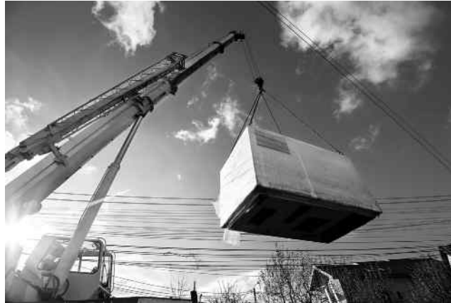
FIGURE 10-2 Crane boom loaded in bending and compression.
