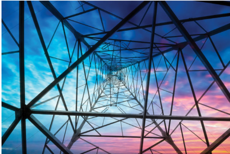
FIGURE 11-1 Trusses are rigid networks of simple two-force members and provide the framework for many structures such as this tall tower. Each member of this tower is long relative to its cross section, so any that is loaded in compression is susceptible to buckling. Care must be taken to ensure that no single member of this structure buckles resulting in a sudden and catastrophic failure of the entire structure.
