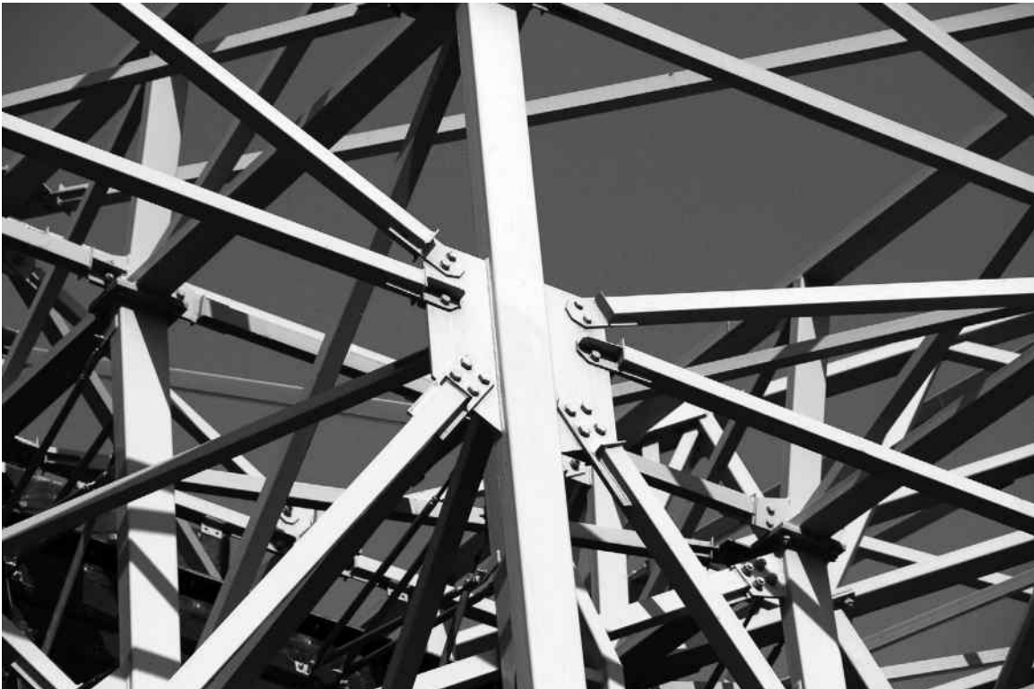
FIGURE 13–1 (See color insert.) Much time and effort is invested in the design and analysis of loads and stresses on machine elements and structural components. Since that loading must be safely transferred to neighboring components, similar diligence must be exercised with regard to connections.
