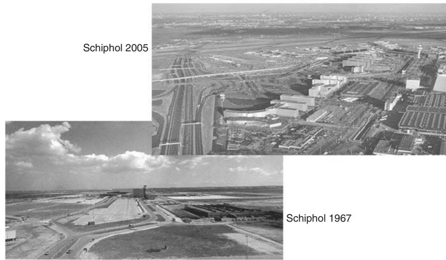
Figure 16.4 Schiphol Airport between 1967 and 2005.
