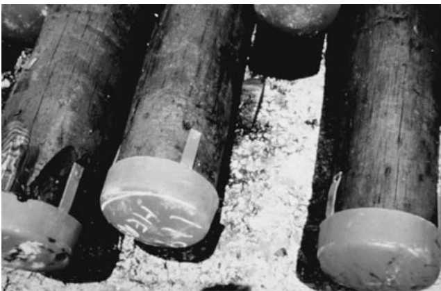
FIGURE 2.53 Wood pile with steel cap.
