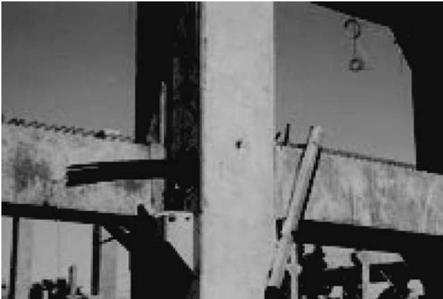
FIGURE 2.15 Pre-stress bridge girder.
