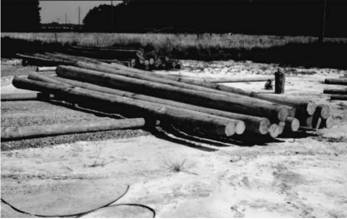
FIGURE 2.52 Preparing wood piles.
