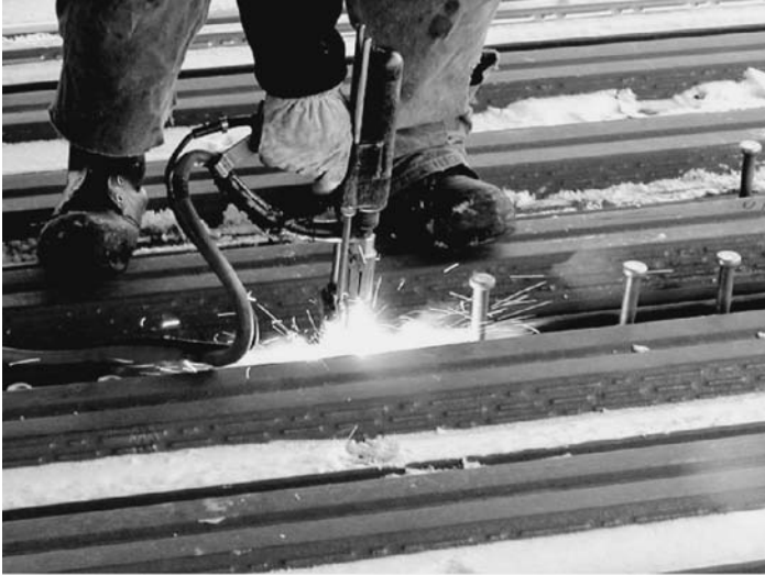
FIGURE 2.27 Fixing stud to floor steel sheet.
