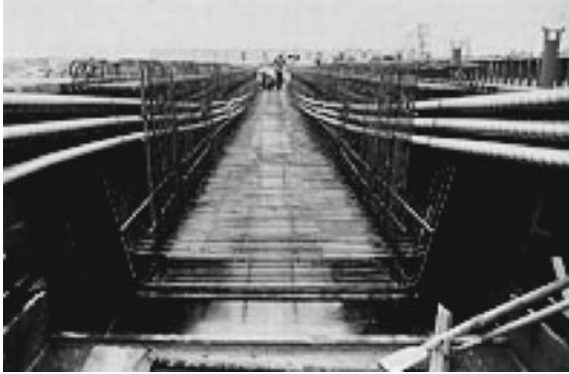
FIGURE 2.11 Pre-tensioned cables.
