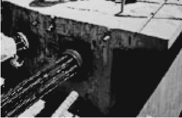
FIGURE 2.14 Placing tensioning wire in bridge girder.
