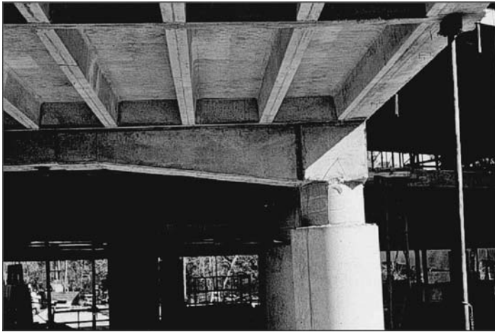
FIGURE 2.7 Pan joist floor system.
