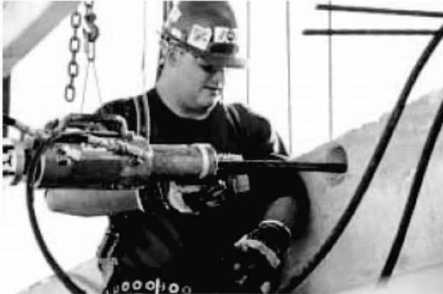
FIGURE 2.12 Tensioning tendon.
