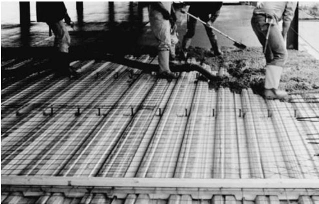
FIGURE 2.30 Pouring concrete after fixing studs.
