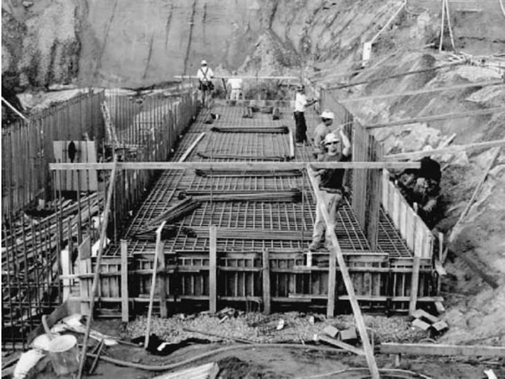
FIGURE 7.14 Steel bars between foundation and wall.
