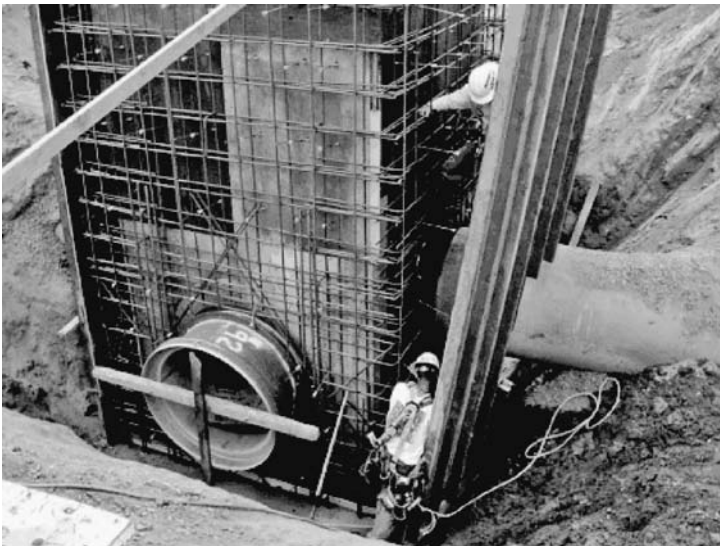
FIGURE 7.13 Wall steel bars with pipe sleeve.
