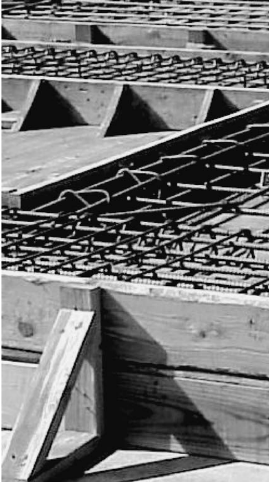
FIGURE 7.4 Strengthening wood form for ground slab.
