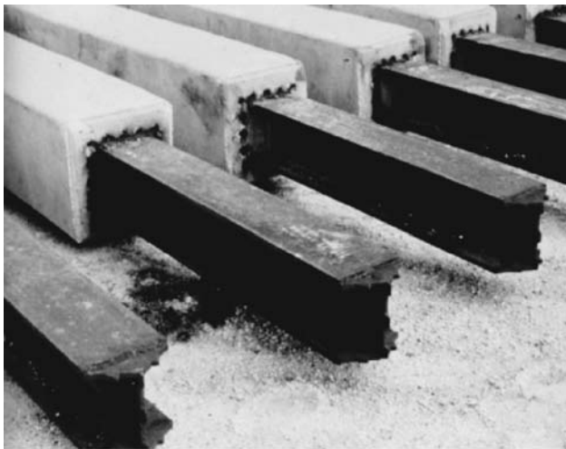
FIGURE 2.58 Composite section piles.
