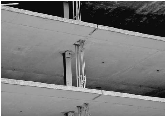
FIGURE 7.10 (Top) Lift slab. (Bottom) Anchoring lift slab.
