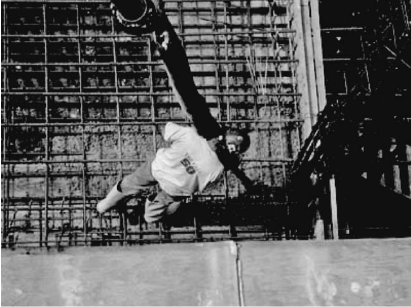
FIGURE 7.26 Pouring concrete slab by pump.
