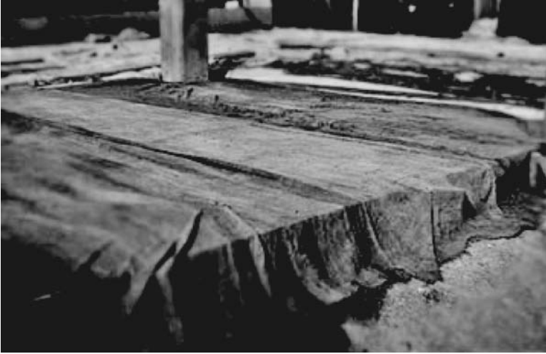
FIGURE 7.35 Curing by using textile.
