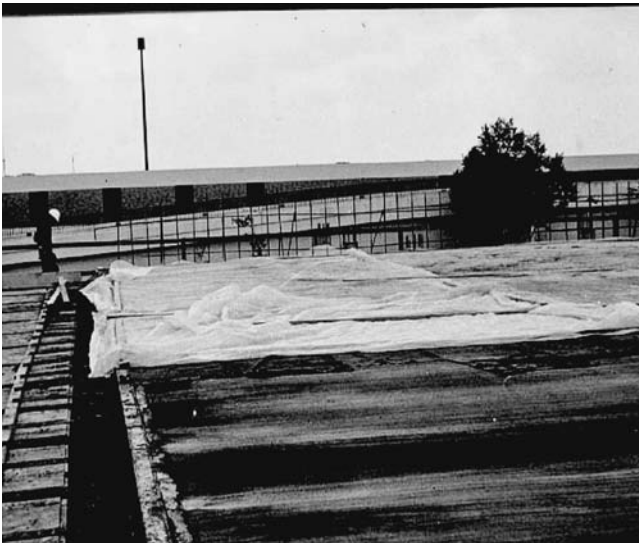
FIGURE 6.17 Curing by using plastic sheet.
