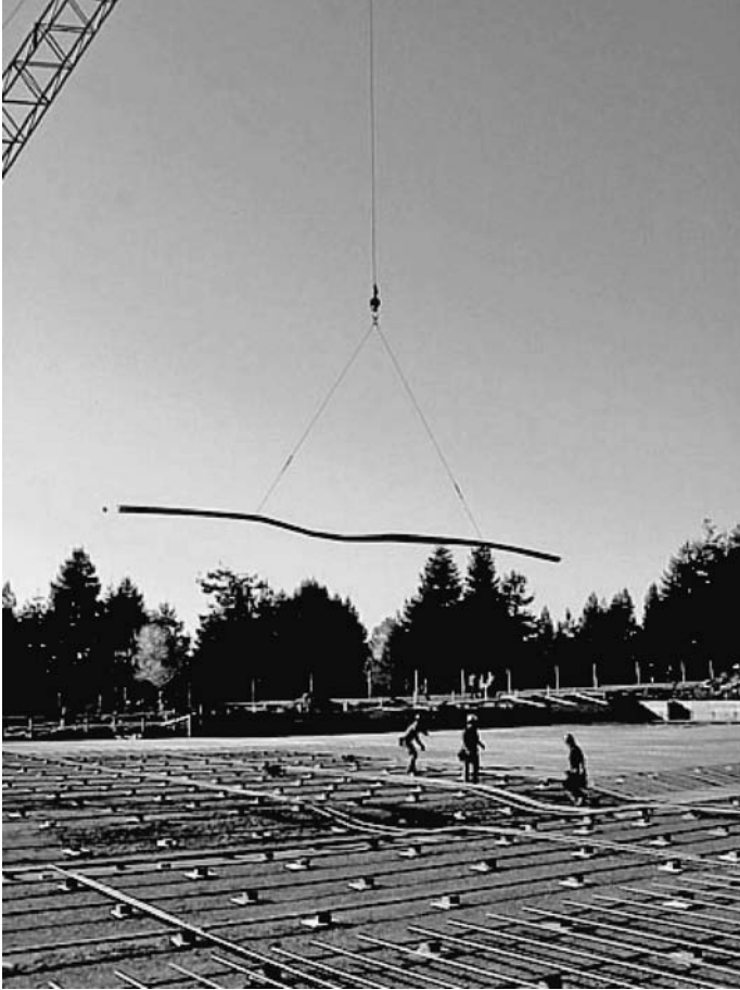
FIGURE 7.11 Distributing steel bars on ground slab.
