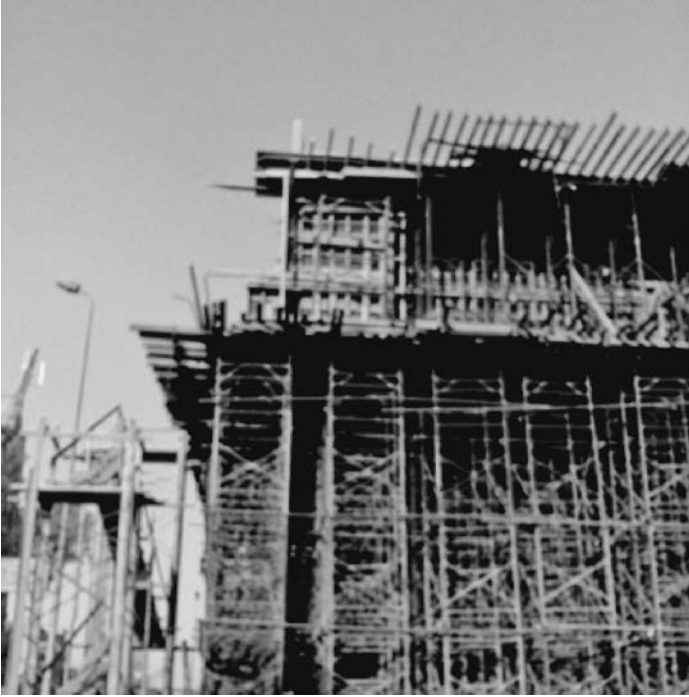
FIGURE 7.2 Bridges slab form support.
