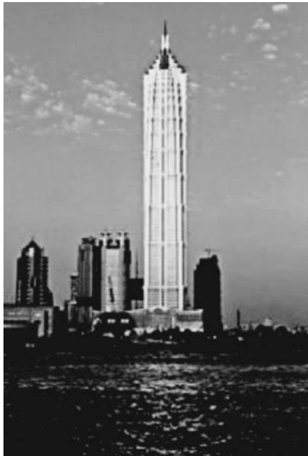
FIGURE 2.44 Jin Mao Building.
