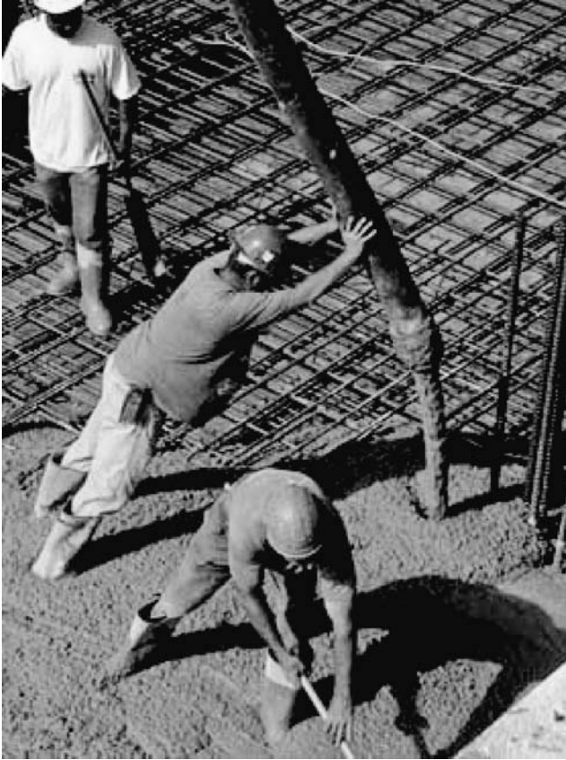
FIGURE 7.28 Preparing concrete surface.
