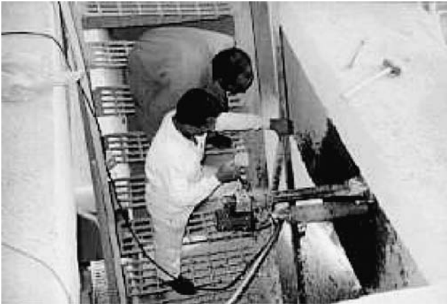
FIGURE 4.12 Core sampling. Note reinforced girder.
