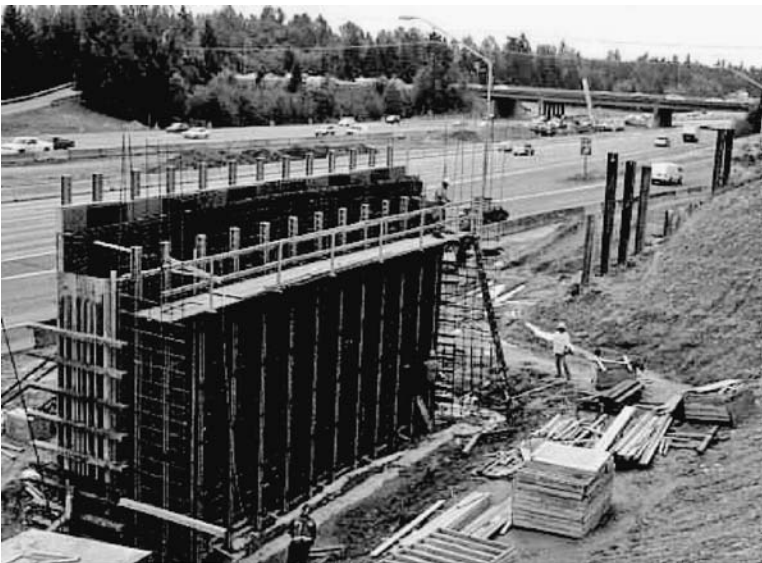
FIGURE 7.1 Formwork for reinforced concrete wall.
