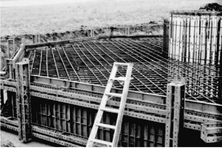
FIGURE 7.5 Steel form for raft foundation.
