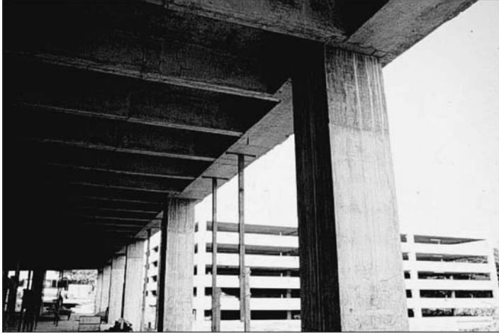
FIGURE 2.6 Pan joist floor.
