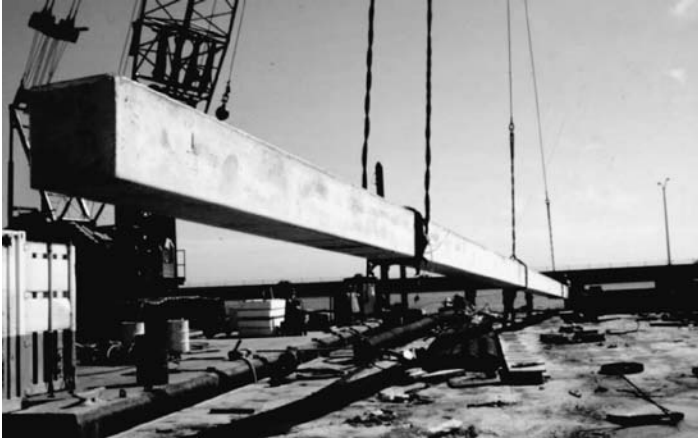
FIGURE 2.56 Lifting of concrete pile.
