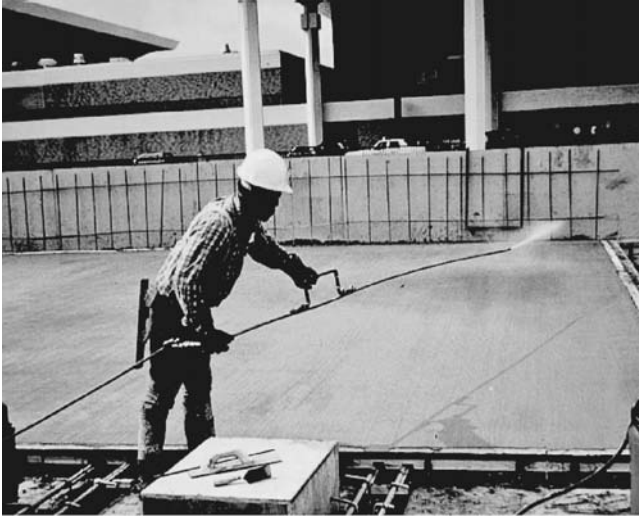
FIGURE 6.16 Spraying chemical compounds.
