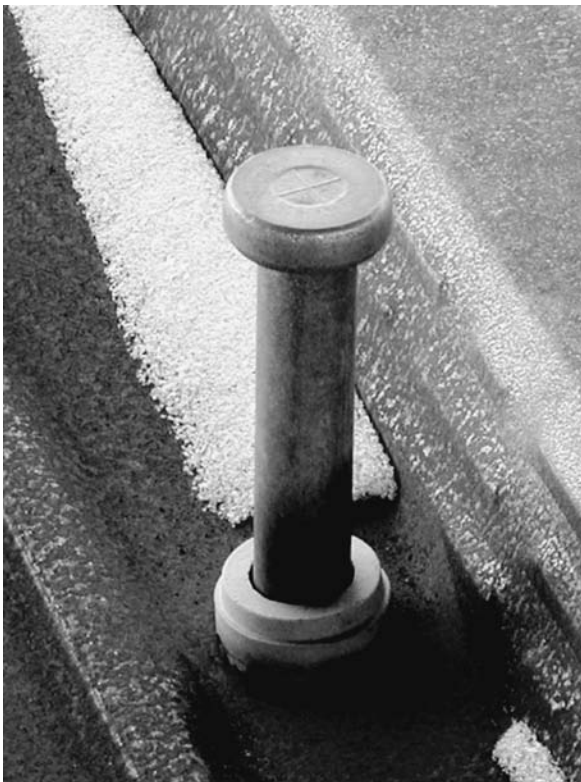
FIGURE 2.28 Fixation of stud.
