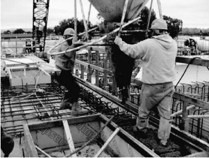
FIGURE 7.27 Pouring beam by using caisson.
