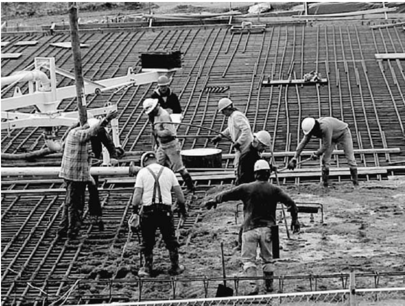
FIGURE 7.25 Pouring part of raft foundation.
