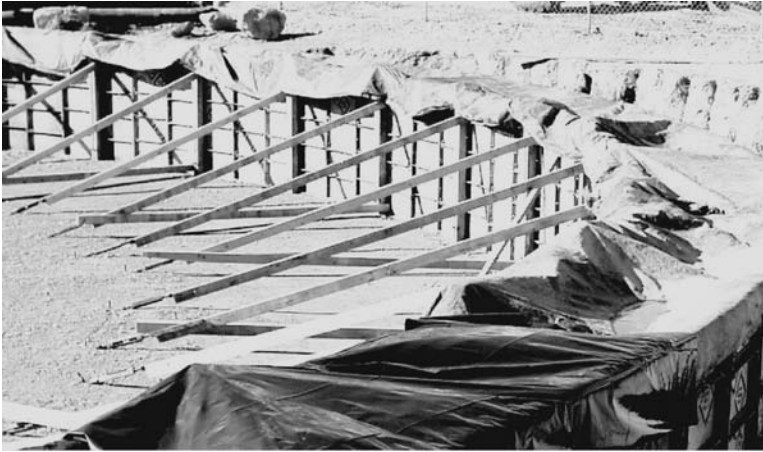
FIGURE 7.37 Plastic sheet to protect from evaporation.
