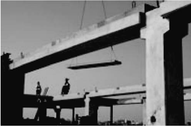
FIGURE 2.17 Installing pre-stress bridge girder.
