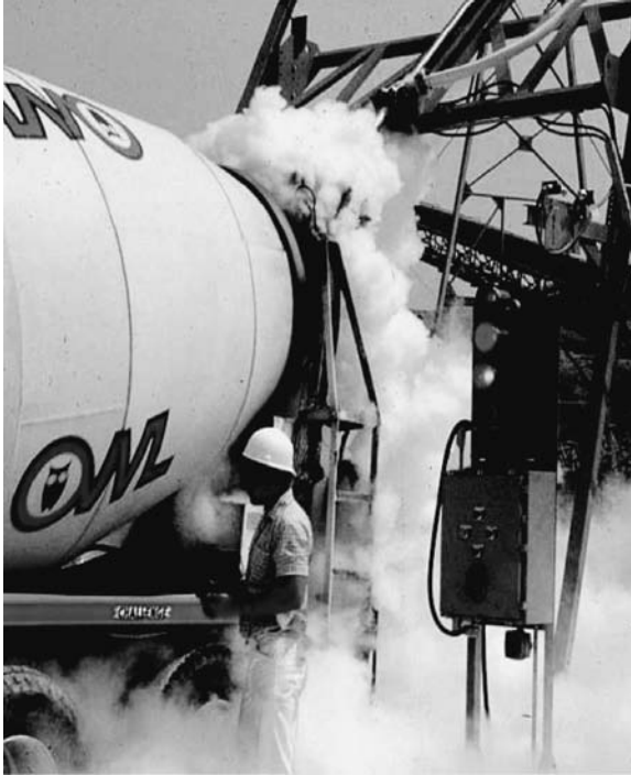
FIGURE 6.4 Using nitrogen for cooling.
