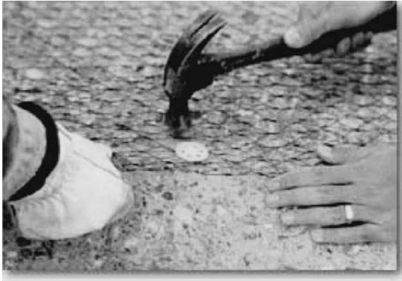
FIGURE 6.26 Fixing titanium mesh with plastic binder.
