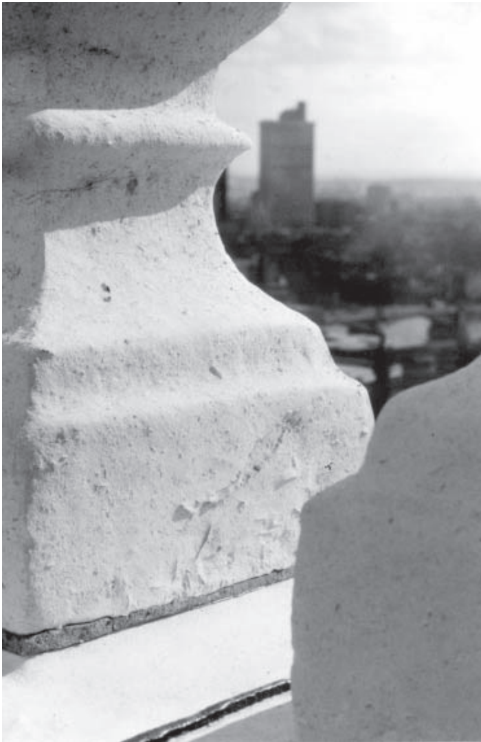
Figure 19.14 Effect of acid precipitation on Portland stone.
