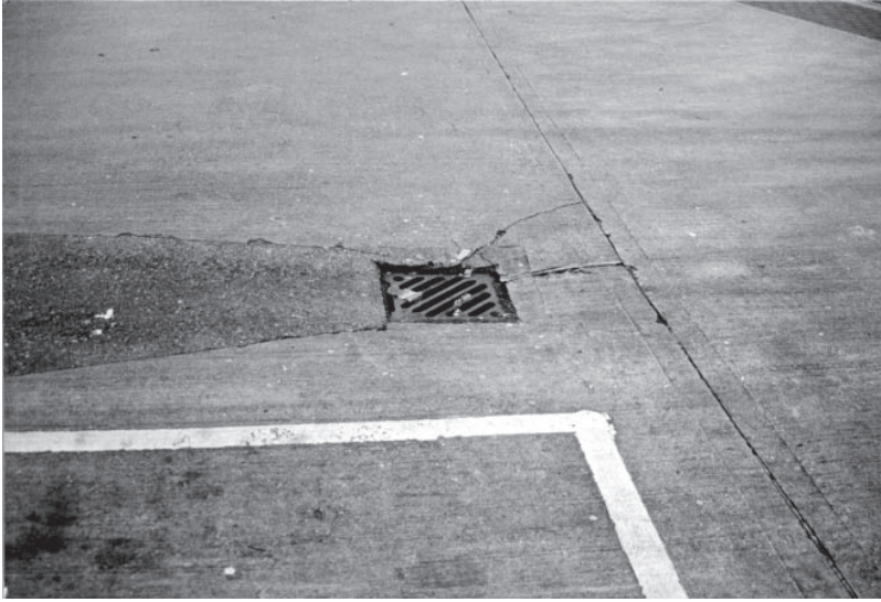
Figure 22.16 Poor detailing.
