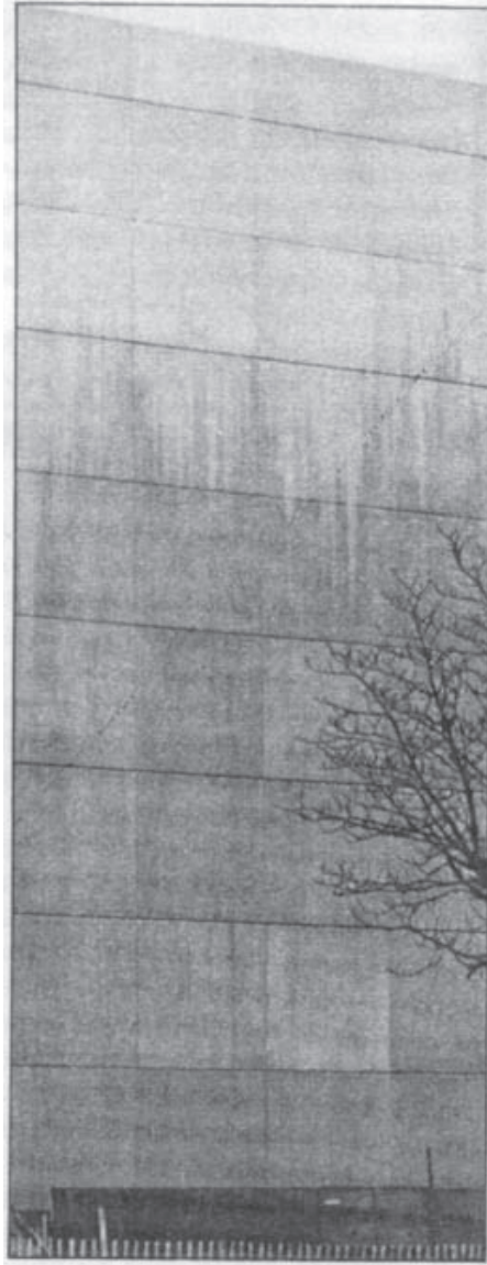
Figure 19.15 Partial washing of large facade caused by variation in amount of rain reaching the facade.
