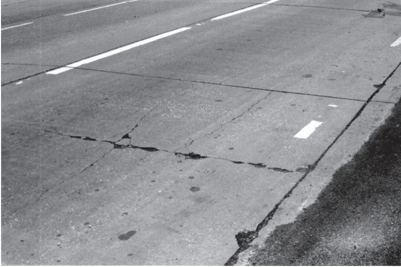
Figure 22.7 Fatigue cracking.
