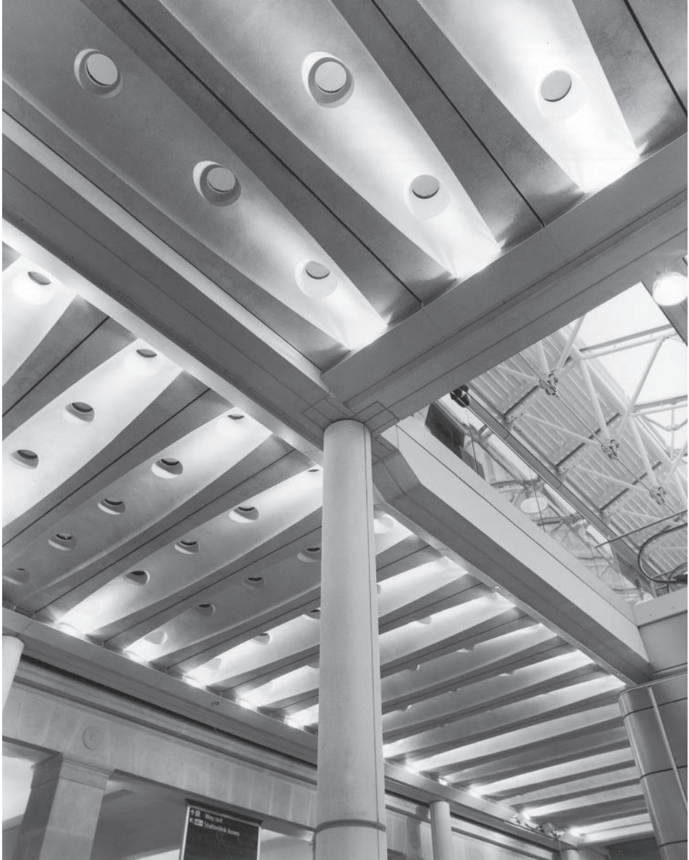
Figure 21.3 Paddington Station, London: Structural steel combined with precast and in-situ concrete, joints first bolted then welded, an elegant example of hybrid construction. (Courtesy Railtrack, Taylor Woodrow Construction and Trent Concrete Ltd.)
