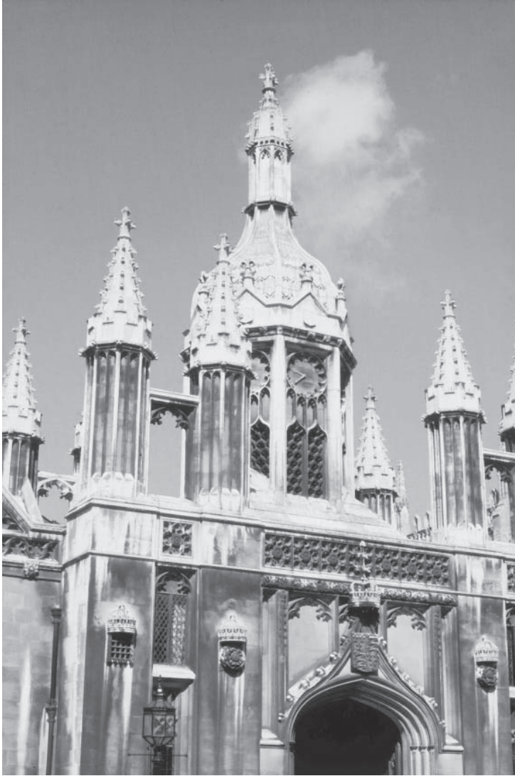
Figure 19.1 Weathering affects all buildings.
