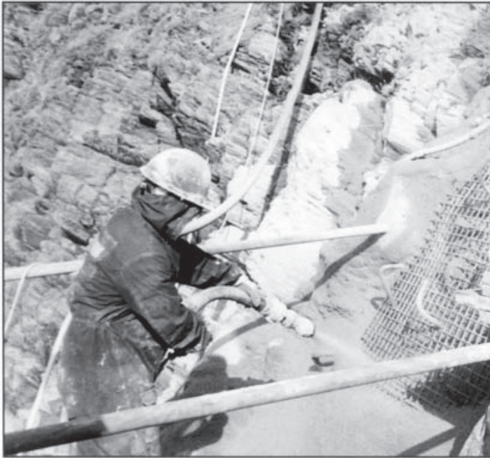
Figure 10.5 Nozzleman at work.
