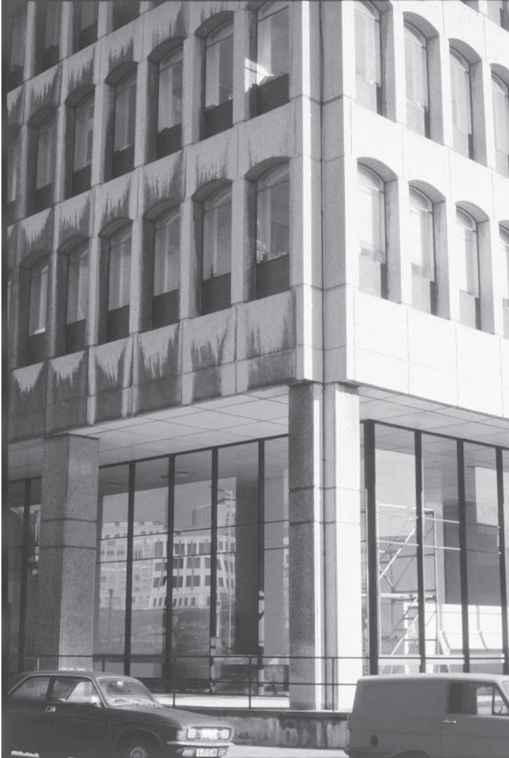
Figure 19.11 North, west and south-west facades with identical materials and details.
