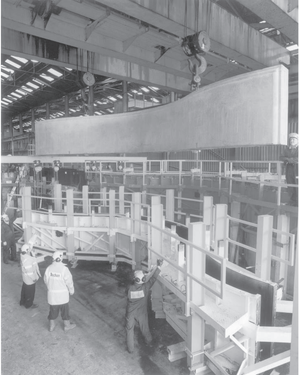
Figure 21.6 Gatwick Airport: Acoustic wall. Stripping a freshly cast element from a purpose-made steel mould. (Courtesy Gatwick Airport Ltd (BAA plc), The Pavement Team (AMECJV) and C.V. Buchan.)
