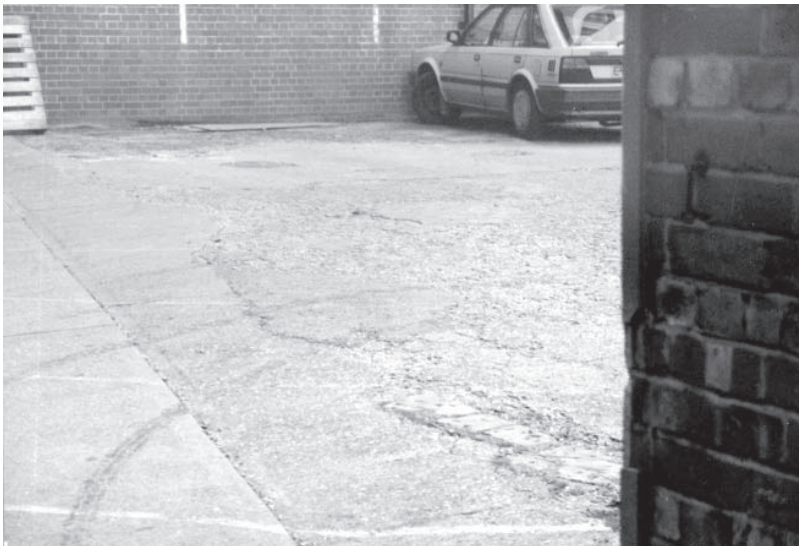
Figure 22.9 Surface abrasion.
