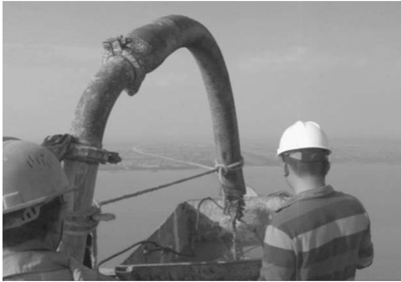
Figure 3-20 Pumping of fiber-reinforced concrete to a height of 306 m at Su-Tong Bridge, Suzhou, China (photo provided by Jinyang Jiang)
