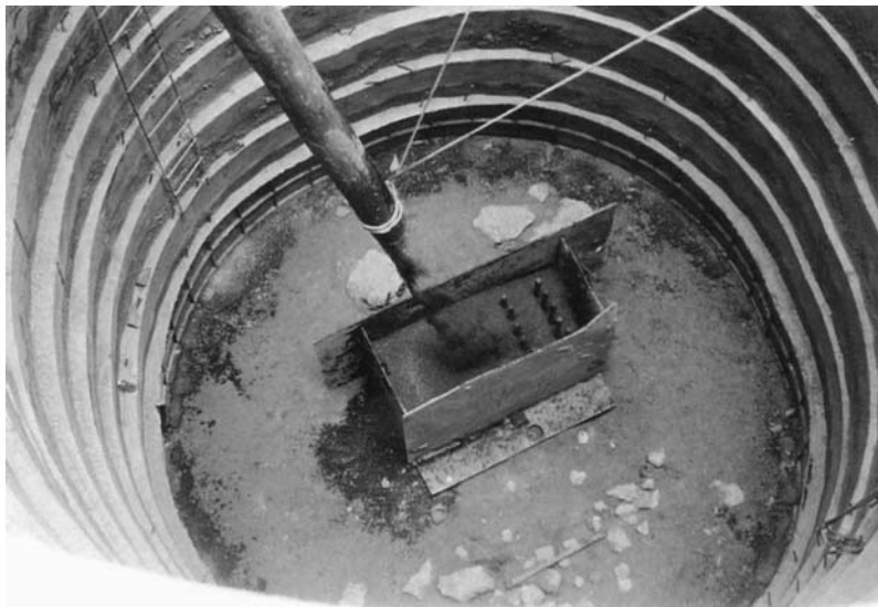
Figure 3-21 Drop chute-guided concrete fall
