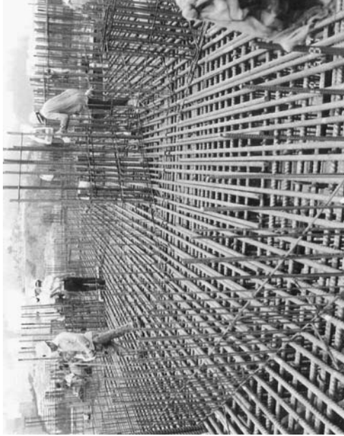
Figure 3-16 Reinforcing steel framework (photo provided by Mr. Peter Allen)
