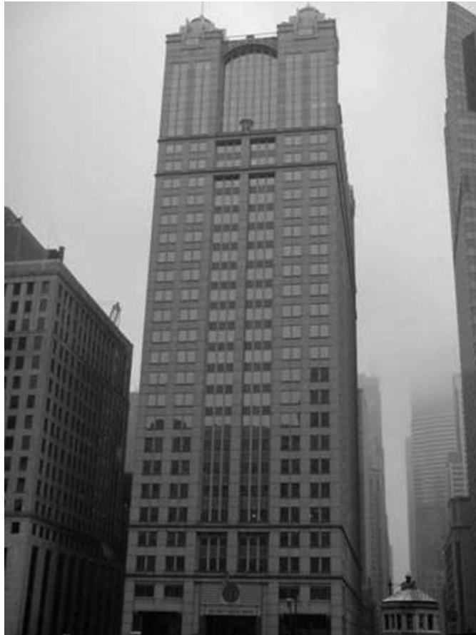
Figure 1-5 The 225 West Whacker Drive building in Chicago, Illinois, USA (Photo provided by Xiaojian Gao)
