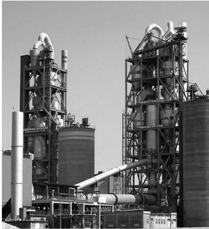
Figure 2-8 A production line of 10,000 metric tons per day (Hai Luo Cement Company, China)
