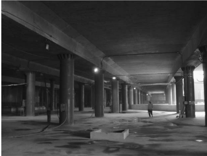
Figure 6-53 Application of CFST as a short axially loaded column in Tianjin Station, China (Photo provided by Linhai Han)
