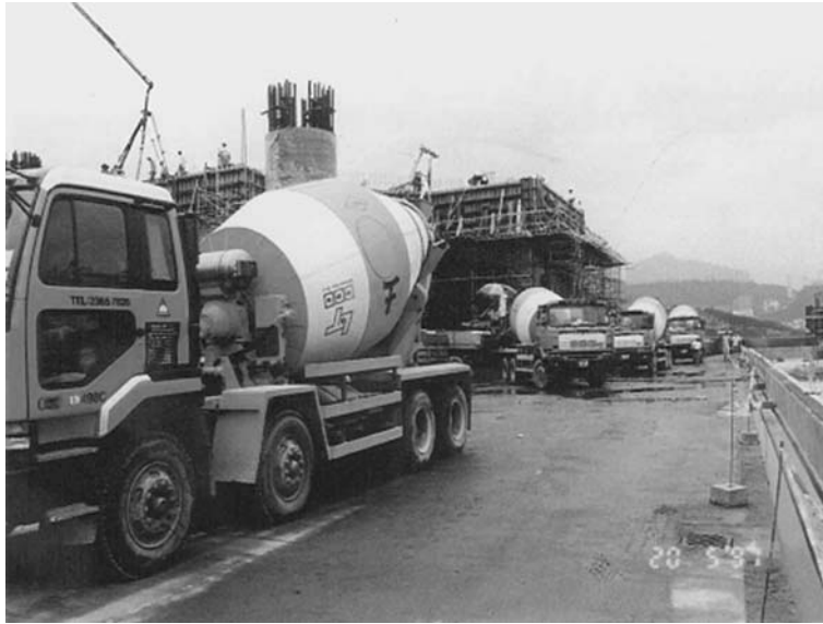
Figure 3-13 Delivery of concrete by truck
