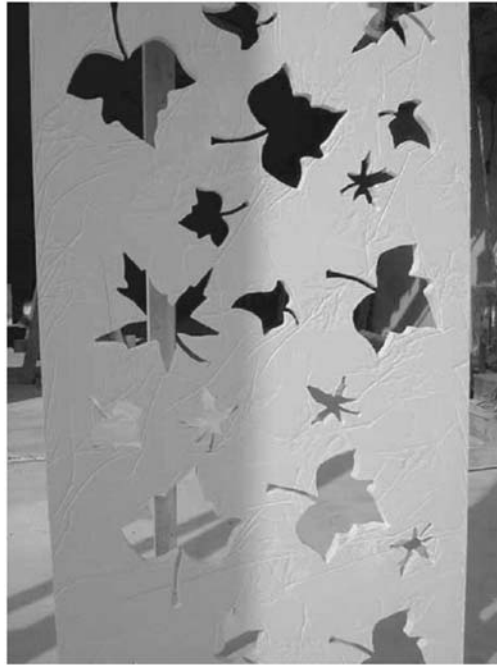
Figure 3-23 Decoration effect of concrete
