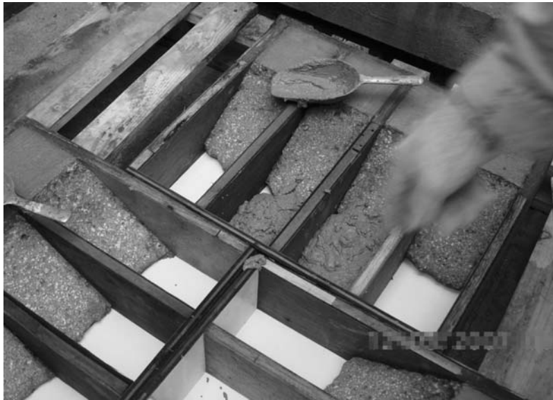
Figure 6-38 Casting of prisms for slant shear measurement
