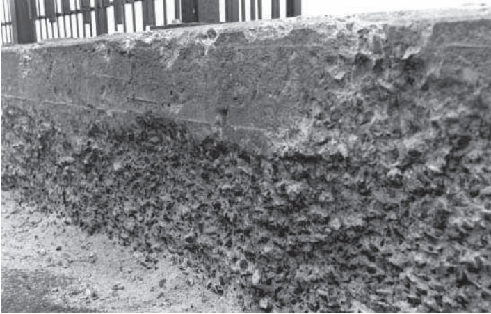
Figure 11.7 Scaling on a wall exposed to de-icing salts during winter. In addition to architectural damage, severe scaling can lead to progressive structural deterioration.
