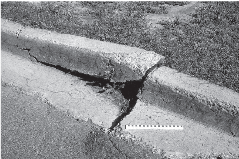
Figure 13.7 ACR in a pavement (sidewalk) and kerb in Ontario, Canada.
