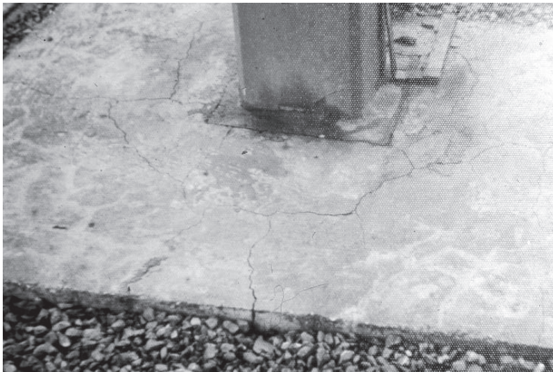
Figure 13.11 Concrete bases in Plymouth, Devon: first identified case of ASR in the UK.
