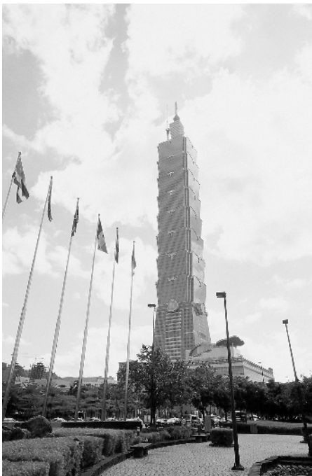
2.15 Taipei 101 Building (Courtesy of Shaw Shieh, Evergreen Structural Engineers and Partners).
