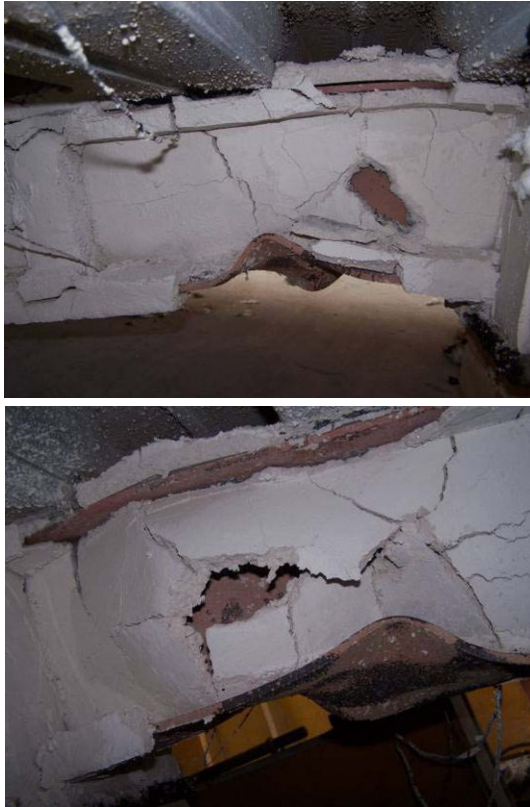
Fig. 7.43 Local buckling of the flange of in test CB125
