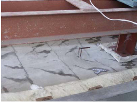
Fig. 7.39 Water exudes through cracks in the slab in the test CB150 (mm)
