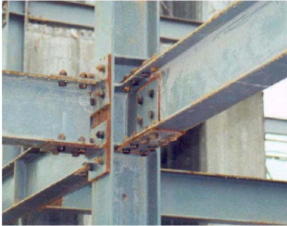
Fig. 8.1 Typical beam-column connection in a framed structure
