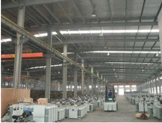
Fig. 11.1 Application of the steel portal frame
