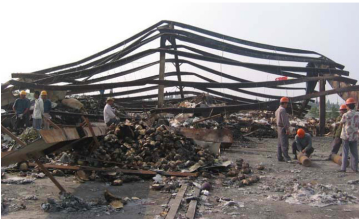
Fig. 1.1 Collapse of an industrial building caused by fire
