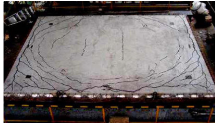
Fig. 9.27 Cracks on S-4 after the test
