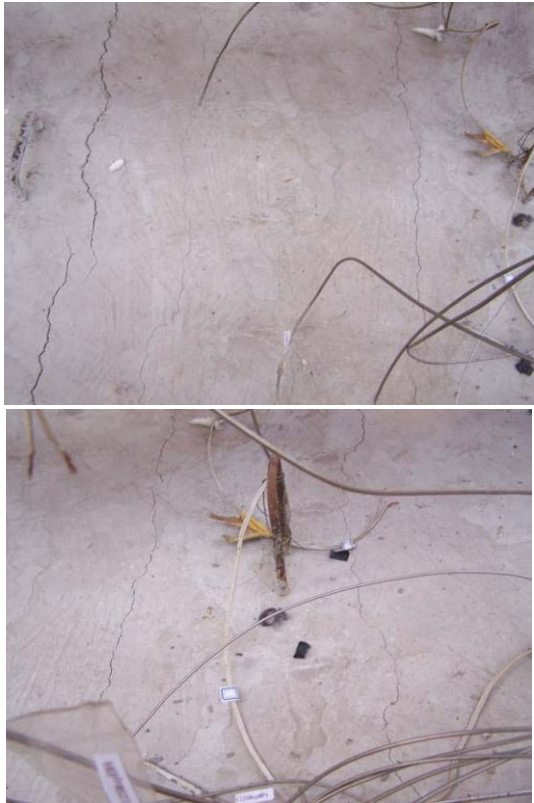
Fig. 7.44 Cracks in the concrete slab in test CB125
