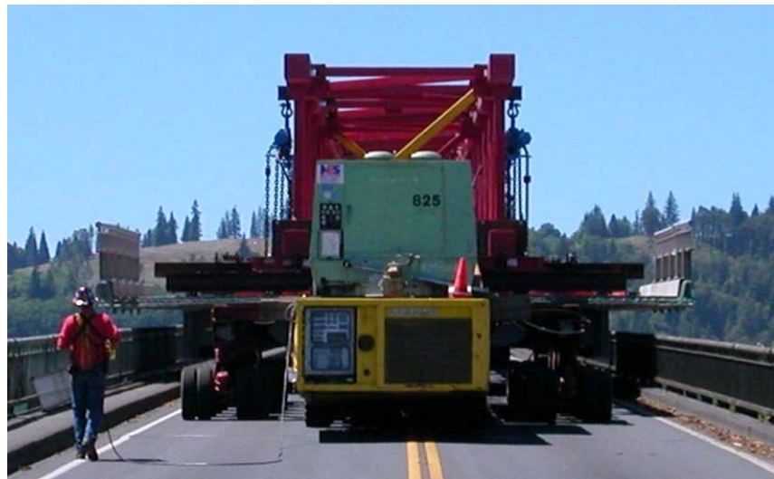
Figure 2.4.4-4 Delivery of Modular Unit using a Gantry Frame
