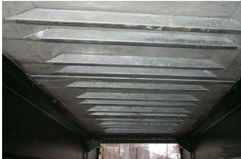
Figure 5.2.3.2.2-3 Underside of the Effideck™ system (source: The Fort Miller Company)
