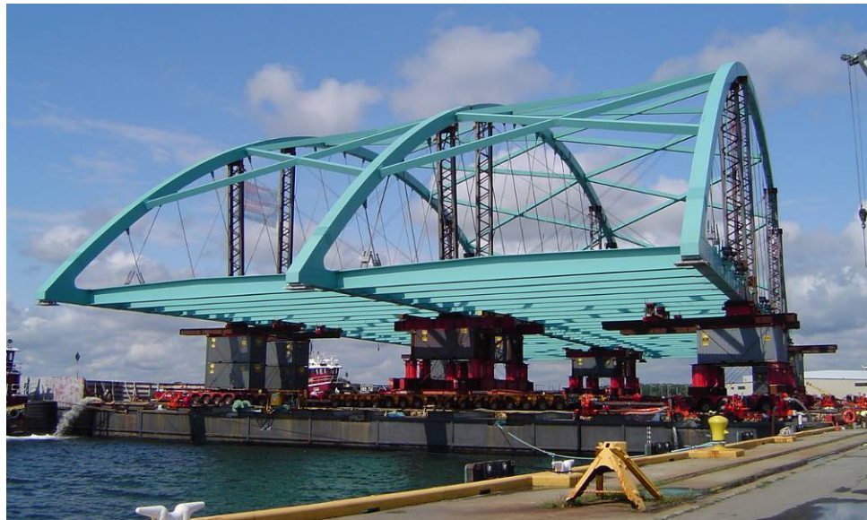
Figure 2.4.1-3 SPMT Bridge Move in Rhode Island
