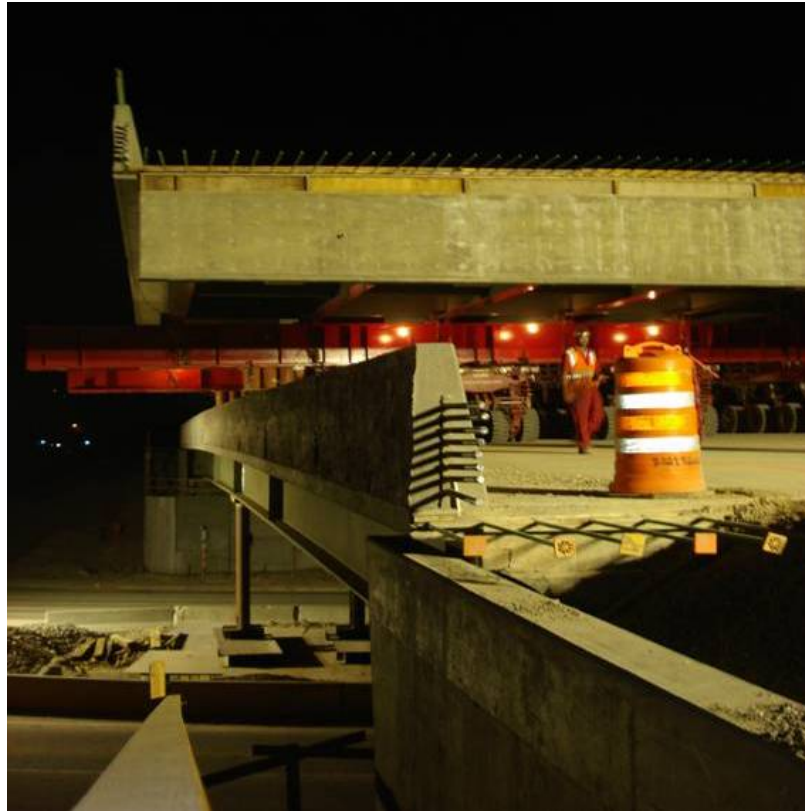
Figure 3.2.1.3-1 SPMT Bridge Move over another Bridge (source: Utah DOT)
