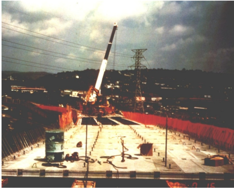
Figure 1.2.1.4-1 Precast Deck Construction in 1990
