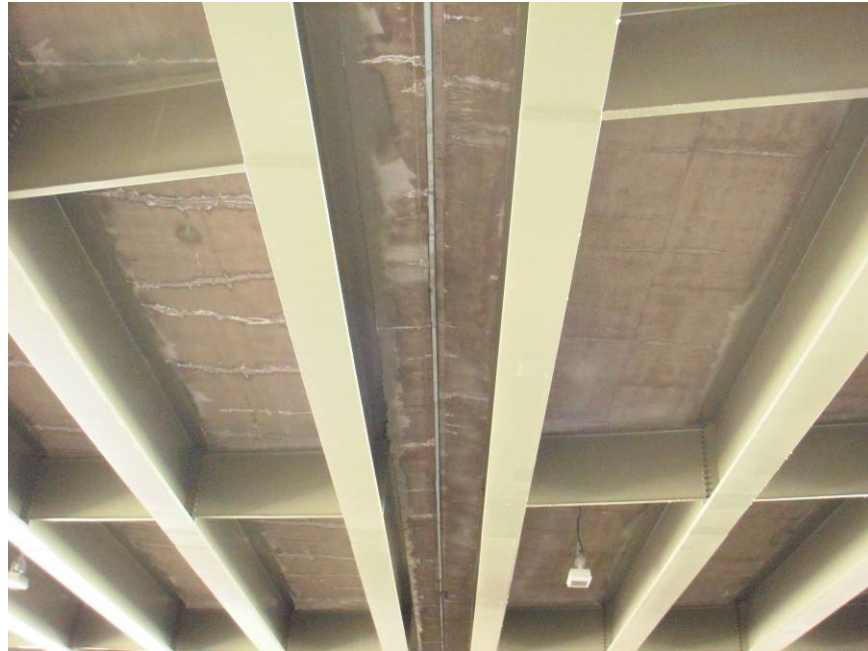
Figure 8.2.1.3-3 Side-by-side Comparison Bridge on right installed with SPMTs Bridge on left built with conventional construction methods (source: Utah DOT)
