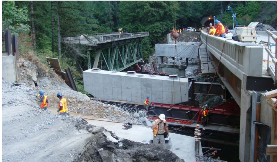
Figure 2.4.3-2 Lateral Bridge Slide in Oregon
