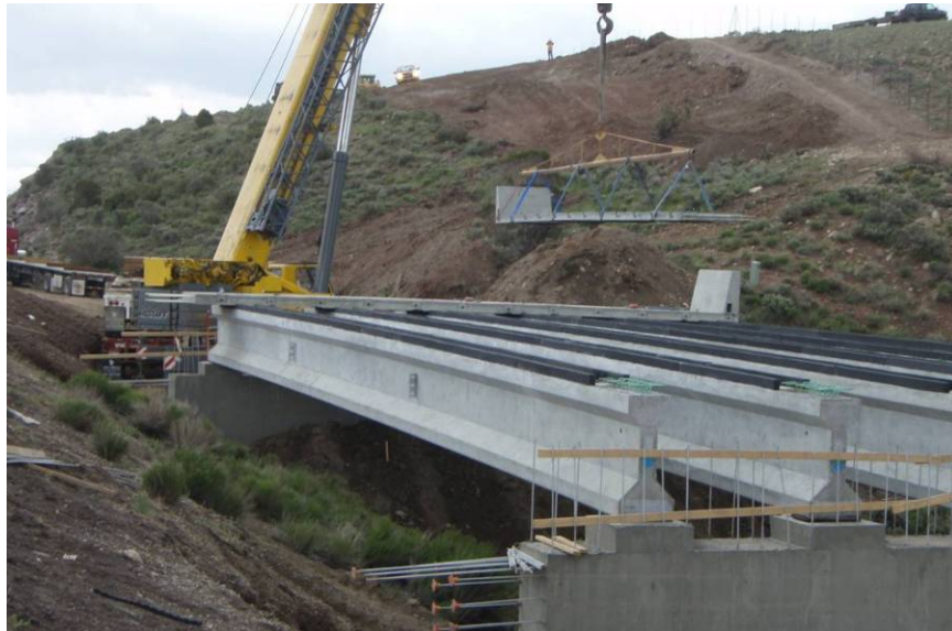
Figure 2.4.5-1 Precast Deck Panel Installation using Cranes (source: Utah DOT)
