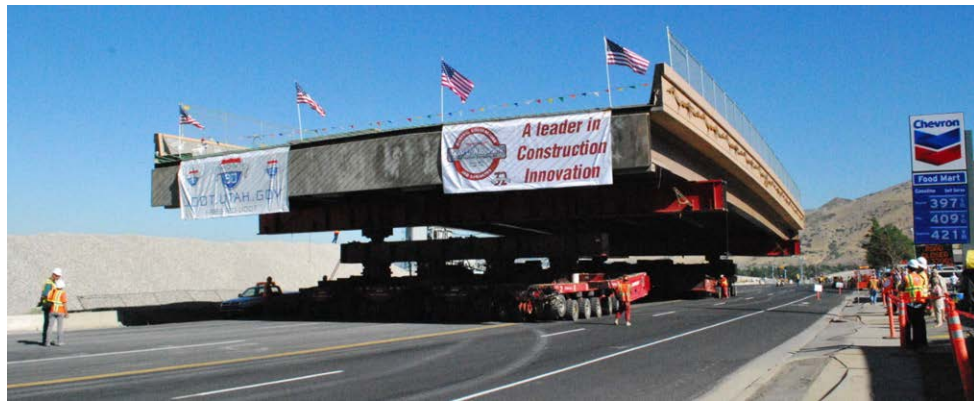
Figure 2.4.1-2 SPMT Bridge Moves in Utah
