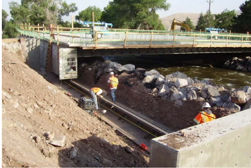
Figure 2.4.3-1 Lateral Bridge Slide in Utah
