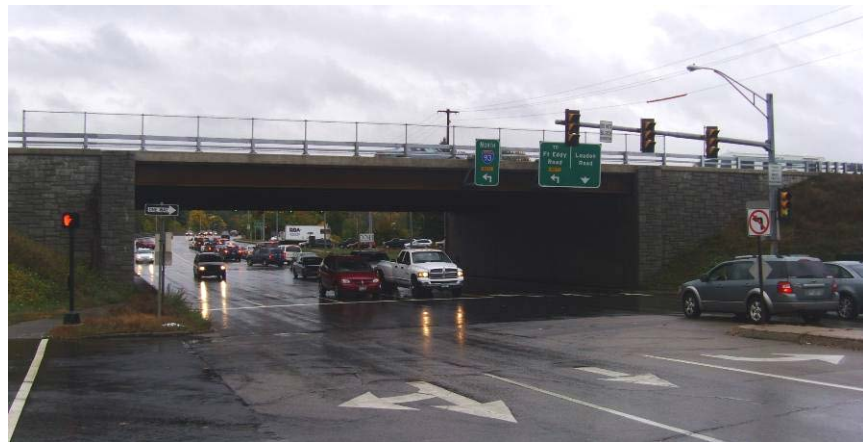
Figure 2.6.1.2-2 Completed Superstructure Replacement Constructed with Prefabricated Elements
