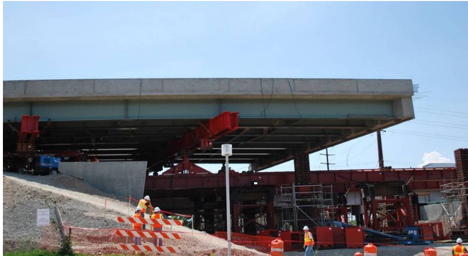
Figure 2.4.2-1 Longitudinal Launching of a Utah Bridge (source: Utah DOT)
