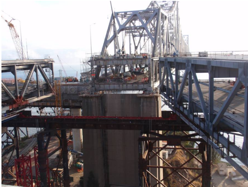
Figure 2.4.3-3 Lateral Bridge Slide of the Oakland Bay Bridge Approach (source: Mammoet)
