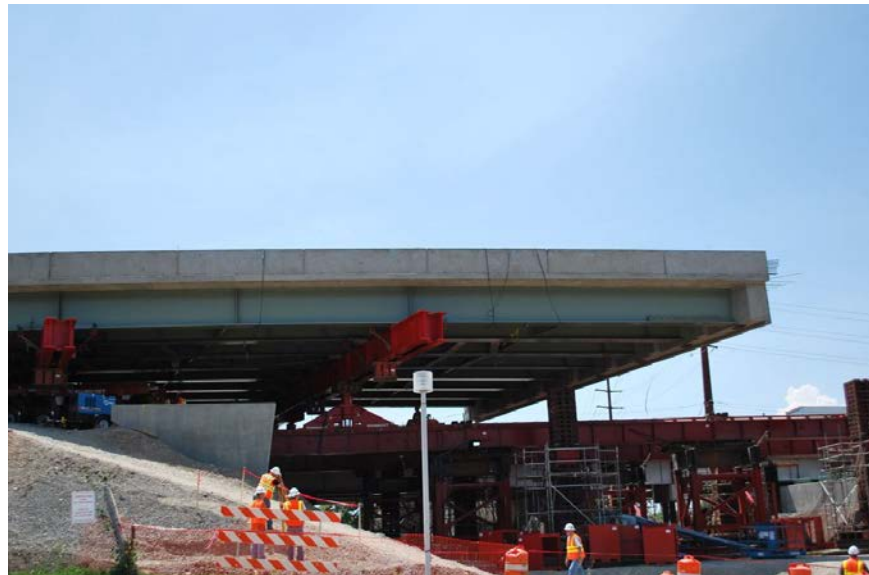
Figure 8.2.1.3-1 Utah DOT I-80 Westbound Bridge Installation (source: Utah DOT)
