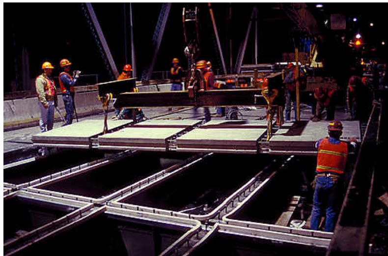
Figure 5.2.3.2.2-2 Exodermic Deck Installation (source: D.S. Brown Company)
