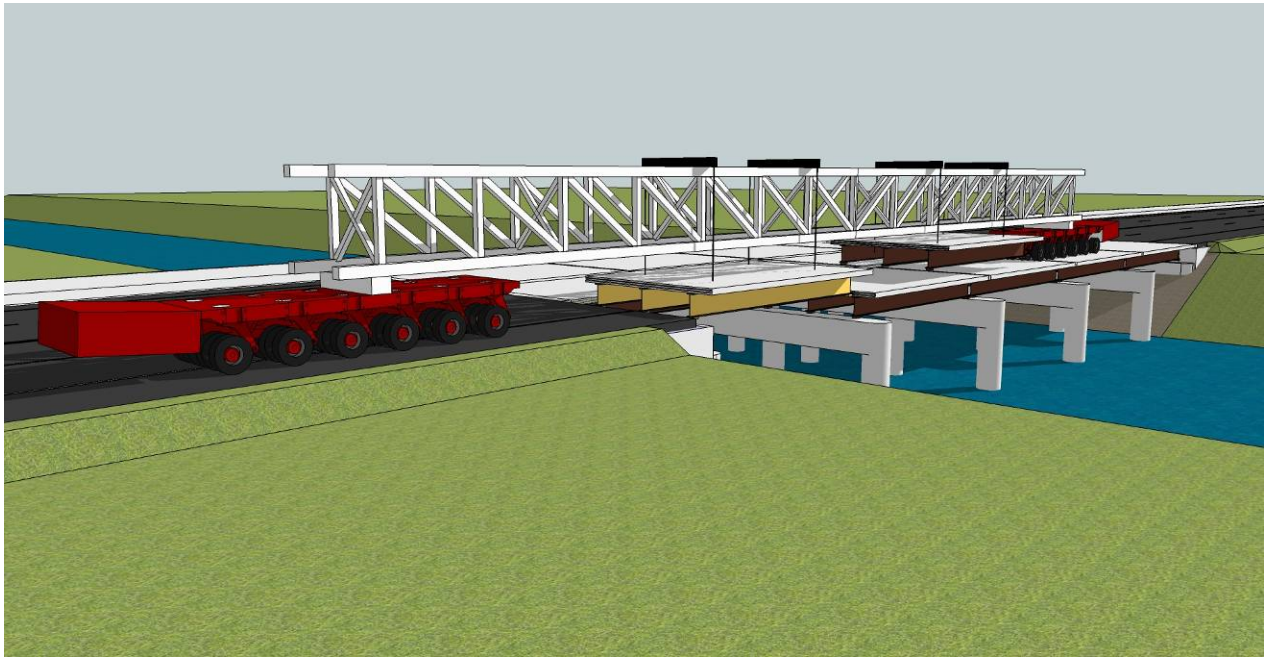
Delivery of New module and Removal of Portion of Bridge using the Gantry Frame
