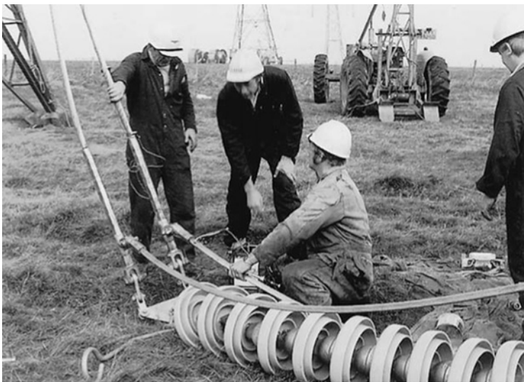
Figure 17.15 400 kV cap and pin insulator set. Low resistance 'ducter' testing on connections in progress
