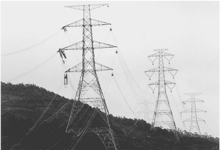
Figure 18.20 Conductor stringing, 500 kV double circuit, quad conductor, Daya Bay, China
