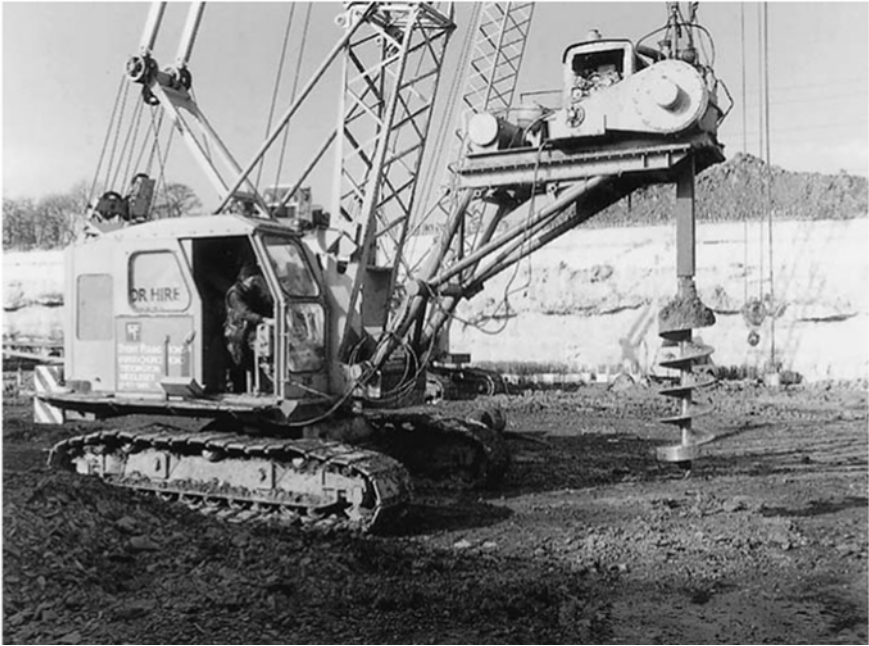
Figure 15.5(a) Auger for forming bored cast- in-situ concrete piles (courtesy of Stent Foundations, Balfour Beatty)
