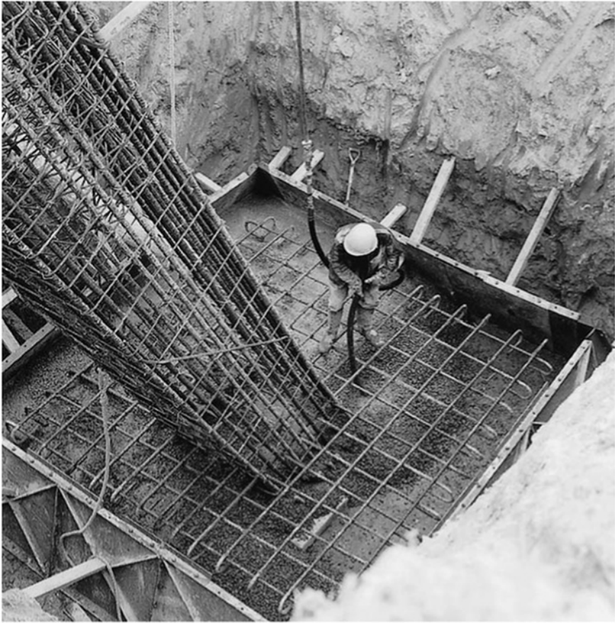
Figure 15.4(b) Pad and chimney foundation steelwork – concrete pour in progress
