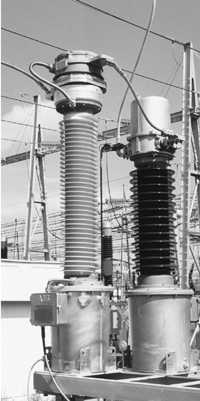
Figure 5.7 Optical CT HV installation (courtesy of ABB)
