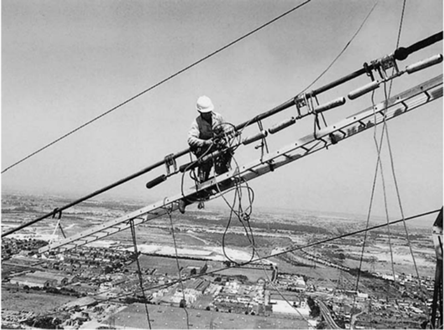
Figure 18.19 Vibration damper replacement, 400 kV Thames crossing reinsulation
