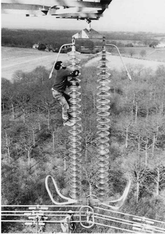
Figure 18.18 400 kV Lydd-Bolney (UK) overhead line—quad conductor glass insulators showing arcing horns and stockbridge dampers
