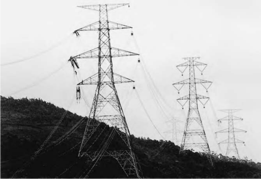
Figure 18.20 Conductor stringing, 500 kV double circuit, quad conductor, Daya Bay, China
