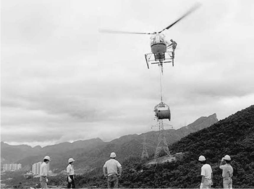
Figure 16.3 Helicopter assisted conductor stringing – Hong Kong (courtesy of Balfour Beatty)
