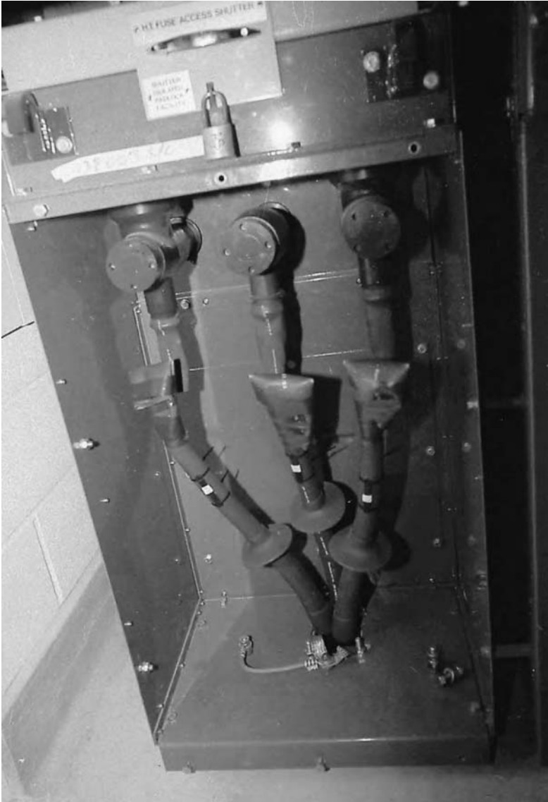
Figure 12.2 24kV heat shrink sleeve termination awaiting final connections
