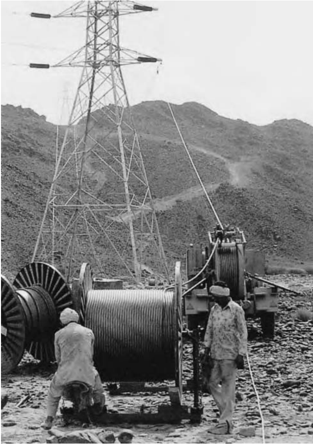
Figure 18.21 Conductor running out in progress. Tensioner and drums at 60 degrees angle tower. United Arab Emirates – 132kV East Coast Transmission
