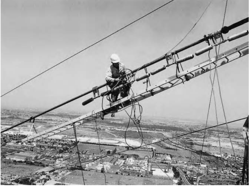
Figure 18.19 Vibration damper replacement, 400 kV Thames crossing reinsulation
