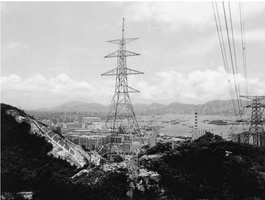
Figure 17.16 500 kV double circuit tower erection in progress, China
