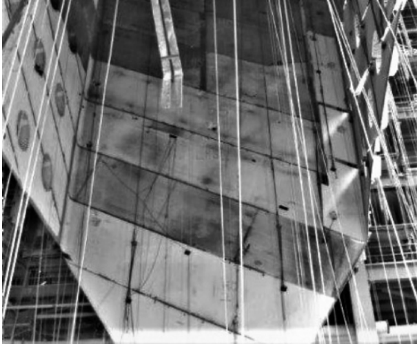
Figure 2.4 A once-through boiler's spiral water walls. Photo courtesy of Doosan Babcock
