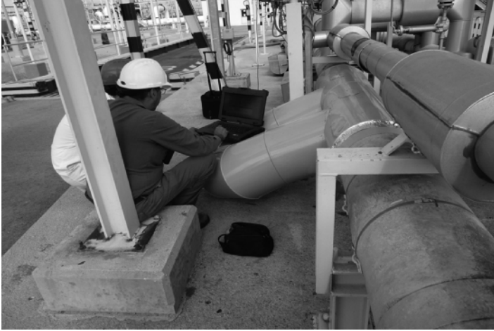
Figure 5.31 Coriolis meter used for gas flow. © Emerson, reproduced with permission
