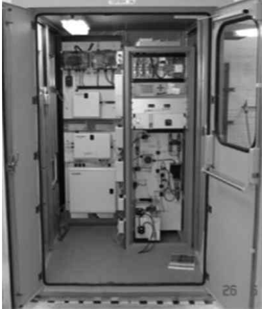
Figure 5.46 Typical extractive CEM. © Servomex, reproduced with permission
