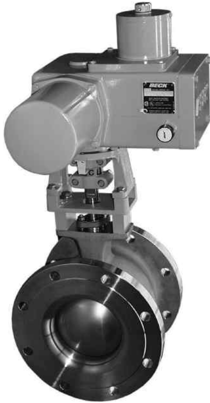
Figure 8.9 Beck electric actuator on quarter turn valve. © Beck, reproduced with permission
