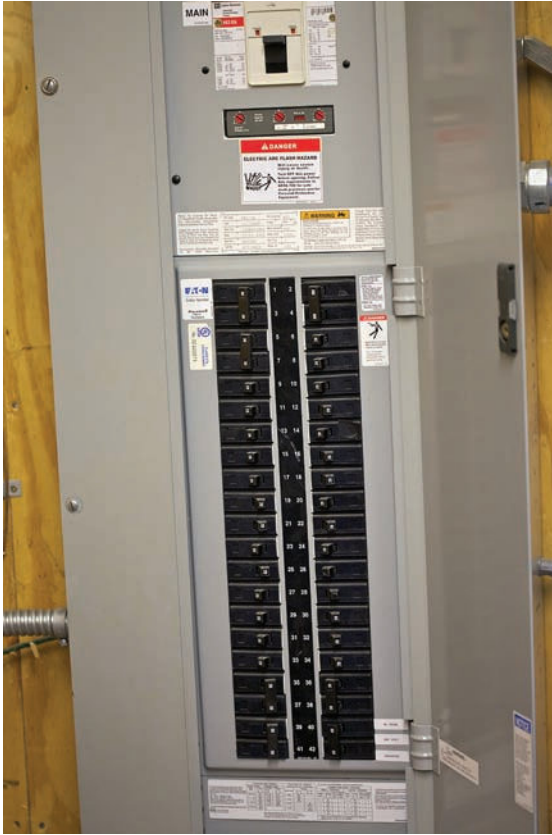
FIGURE 3-5 A 200-amp entrance panel with double-pole main breaker and main bonding jumper.
