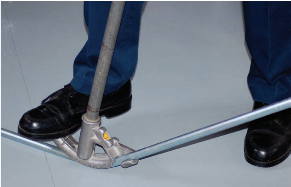
FIGURE 7-11 Bending EMT.
