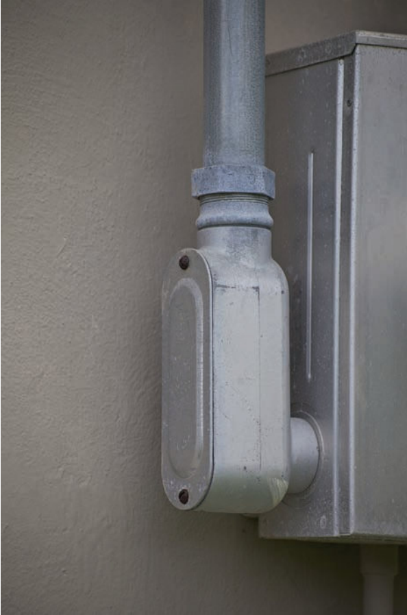
FIGURE 4-8 An LB, available in metal or PVC, is used where an underground service lateral enters the building.
