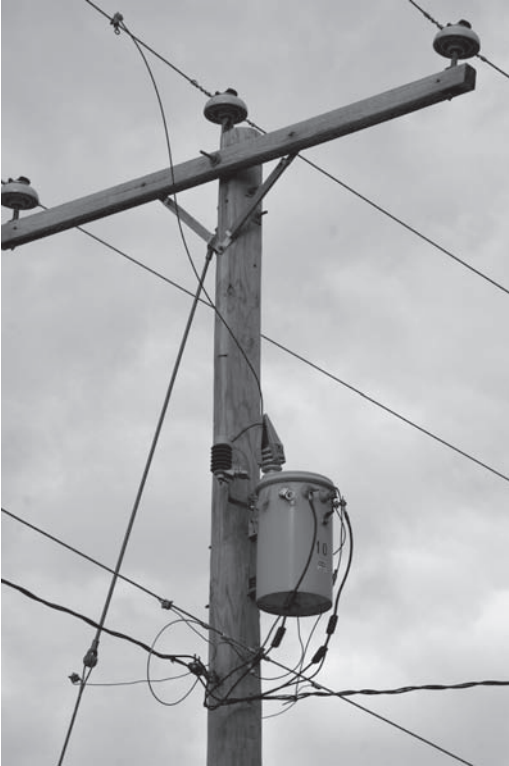
FIGURE 7-1 When designing an aerial service, a clear shot at the transformer is needed.
