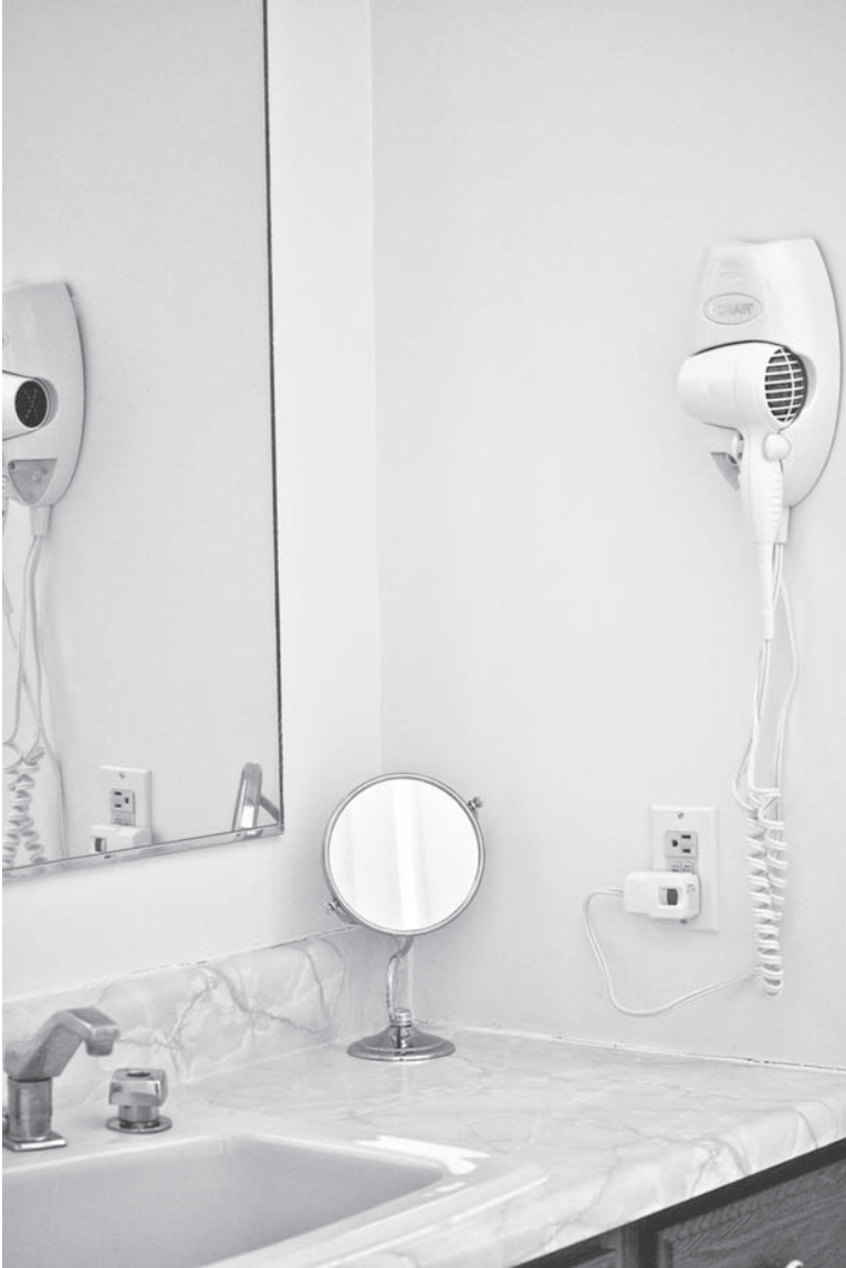
FIGURE 1-5 A hair dryer with a cord-type GFCI is plugged into a receptacle-type GFCI.
