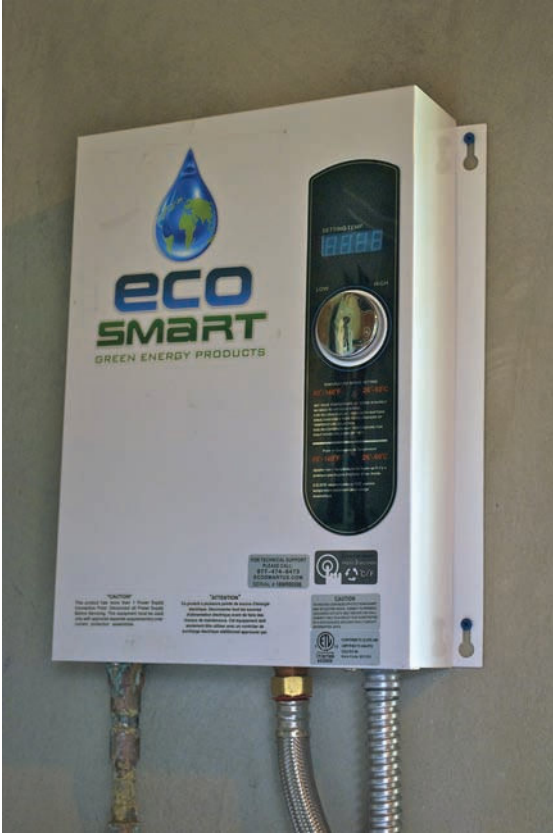
FIGURE 5-11 A tankless (quick-recovery) hot-water heater draws more current but for shorter durations than a conventional hot-water heater.
