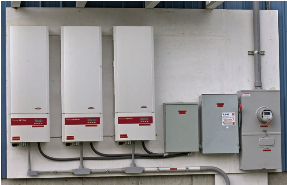
FIGURE G-24 A utility-interactive synchronous inverter. (Courtesy of Kaco.)
