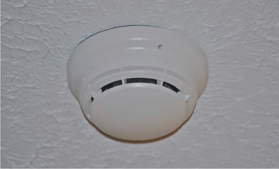
FIGURE 1-3 A smoke detector powered by a 9-volt battery and an ac branch circuit.
