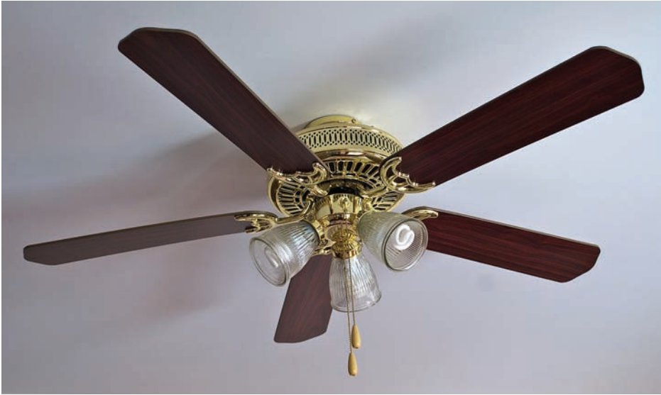
FIGURE 5-9 A paddle-fan luminaire requires special mounting arrangements to make sure that it is secure. Consult the manufacturer's documentation before installing the ceiling box.
