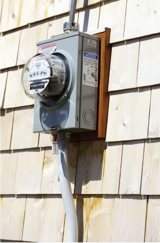
FIGURE 4-6 PVC conduit for the grounding-electrode conductor can be bent by hand after heating it over a charcoal grill. (Practice on scraps first!)
