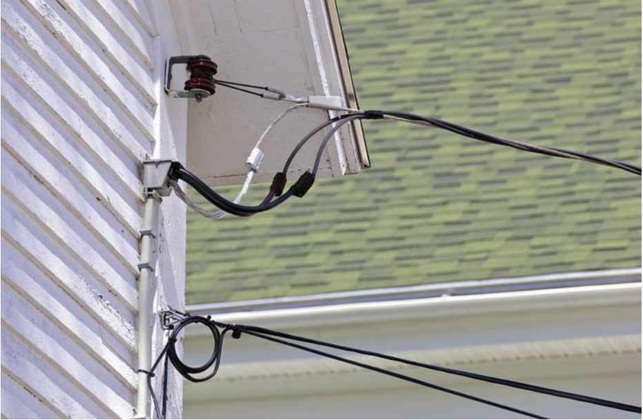
FIGURE G-18 Service drop with point of connection and weatherhead.
