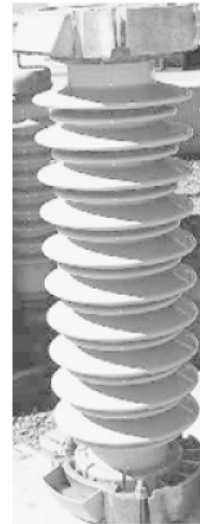
FIGURE 4.28 Post insulators.
