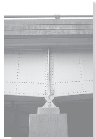
Typical pin used to support the steel girder of a railroad bridge.
