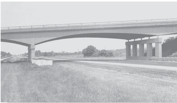
A continuous, reinforced-concrete highway bridge.
