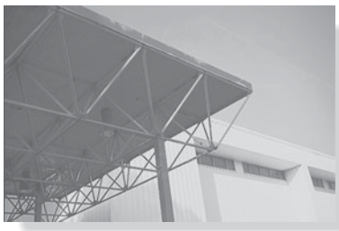
The roof of this pavilion is supported using a system of space trusses.
