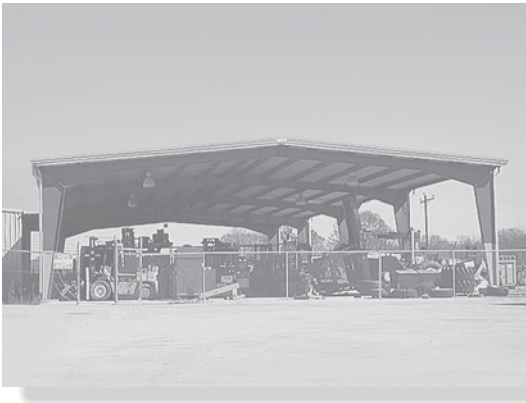
Light-weight metal buildings are often designed using frame members having variable moments of inertia.
