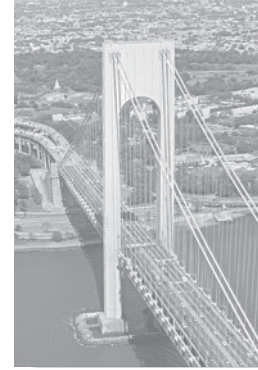
The Verrazano-Narrows Bridge at the entrance to New York Harbor has a main span of 4260 ft (1.30 km).
