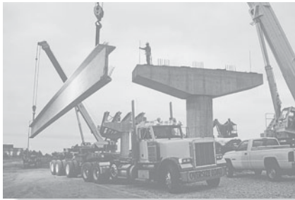
The tapered concrete bent is used to support the girders of this highway bridge.
