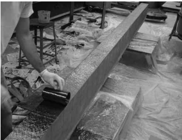
FIGURE 1.1 Strengthening the soffit of inverted reinforced concrete beam with CFRP.
