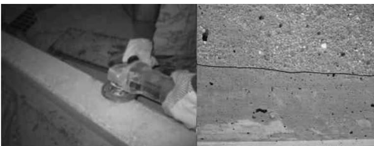
FIGURE 8.3 Grinding of concrete substrate surface (left) roughened vs. original concrete surface (right).
