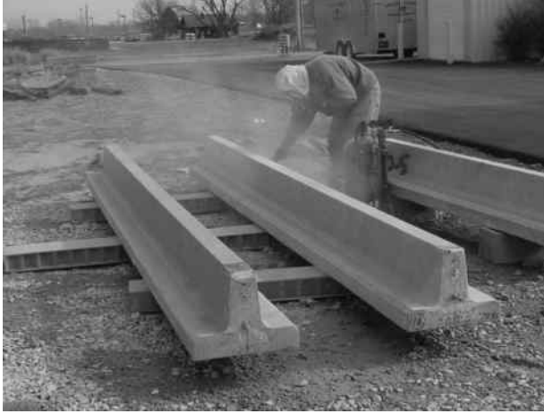
FIGURE 8.4 Surface preparations by sandblasting.
