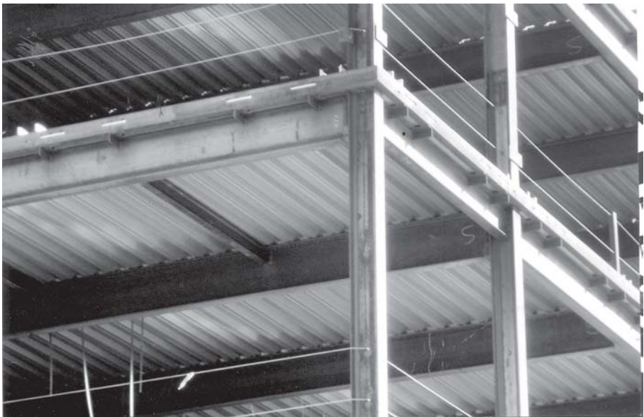
Close-up view of the column of the above building
