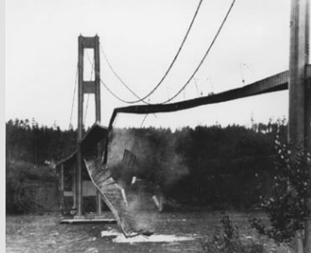
Collapse of the Tacoma Narrows Bridge, (Source: Smithsonian Institution)
