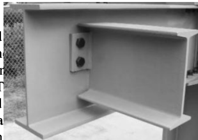
End plate shear connection; the plate in this connection is welded to the web only and bolted to the other member at site (© American Institute of Steel Construction, Inc., Reprinted with permission. All rights reserved.)
