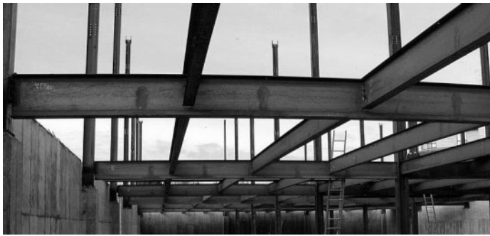
Cross beams bracing main beams (e)
