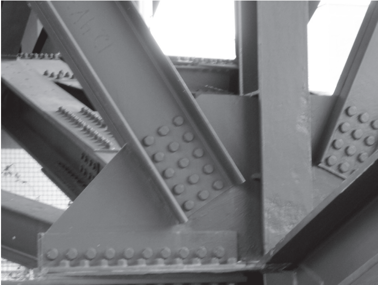
Fig. 10.16 Example of a connection using HSFG bolts
