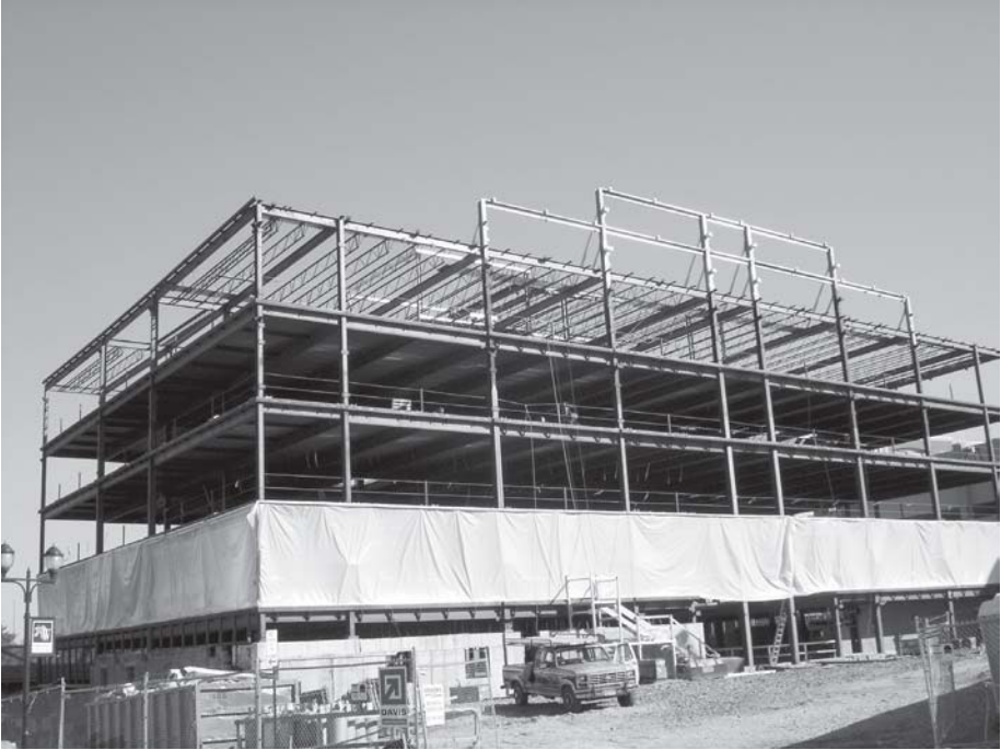
Multi-storey steel building under construction in Maryland, USA
