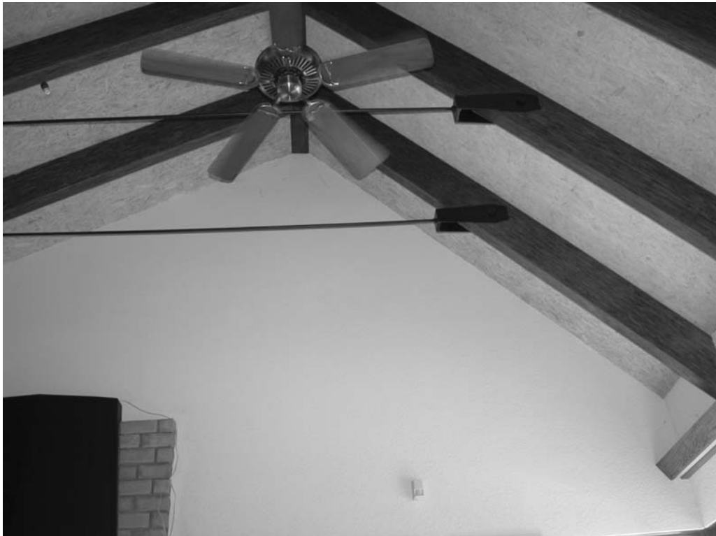
Figure 7.3 Exposed beam ceiling inside of 45° slope roof.
