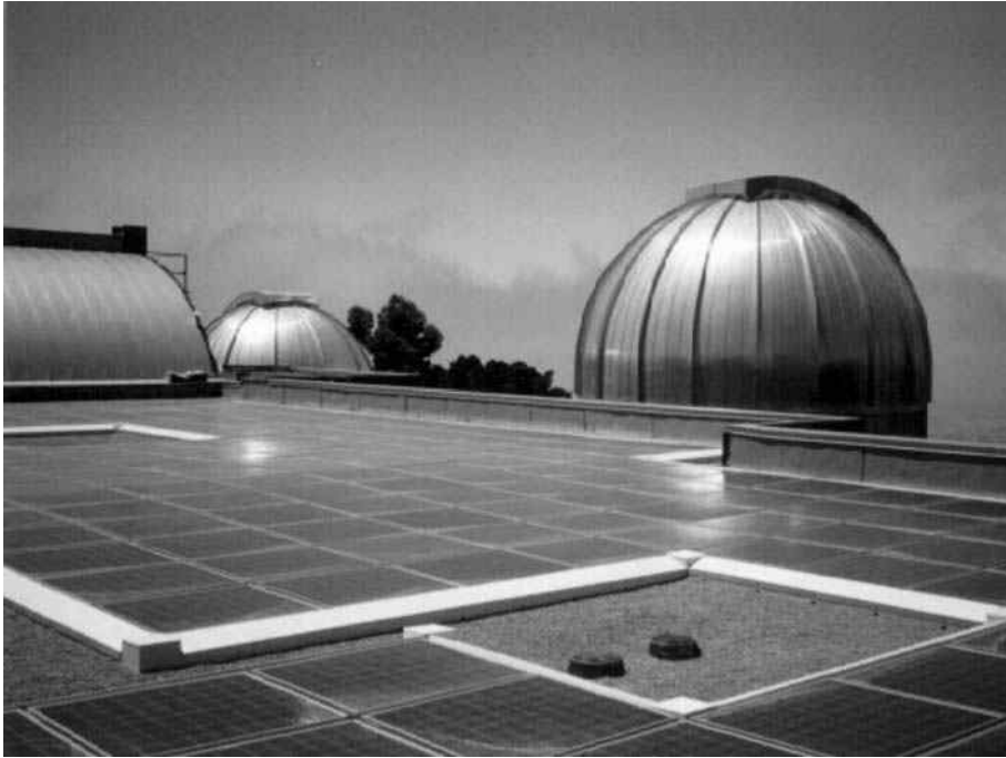
Figure 14.1 Powerlight foam solar PV collector roof tiles.
