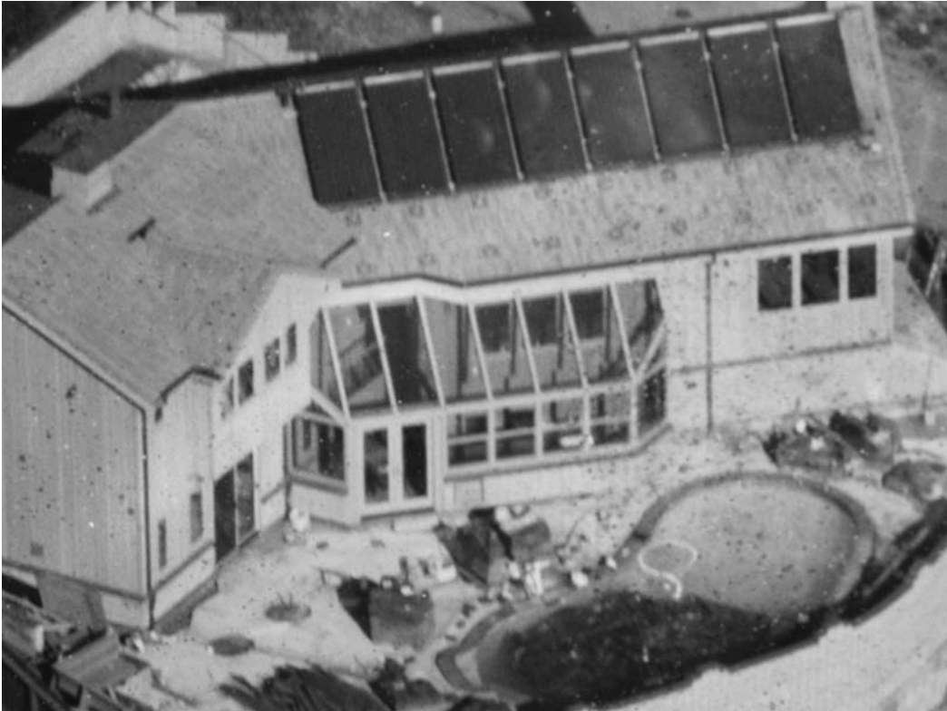
Figure 4.2 Aerial view of solar greenhouse from outside.
