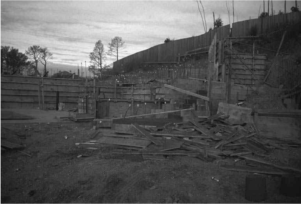
Figure A.1 Foundation concrete pour and start of framing.
