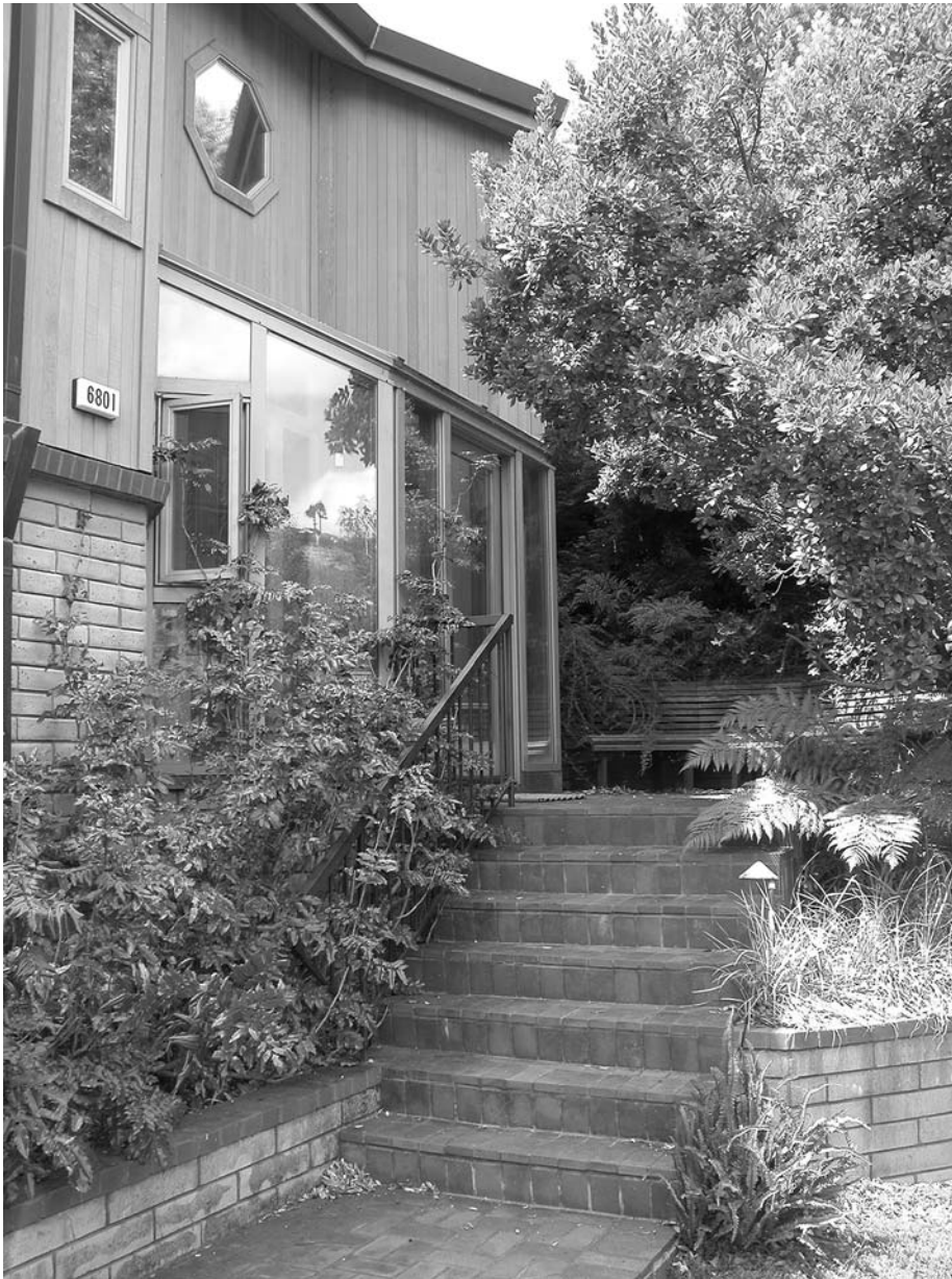
Figure 7.14 Photograph of entry sunroom.
