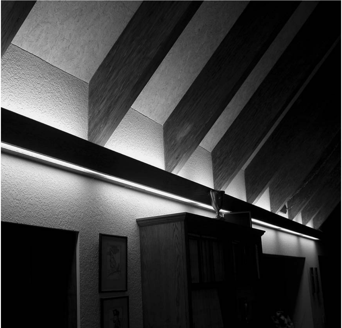
Figure 7.13 Photograph showing soffit lighting of ceiling rafters.
