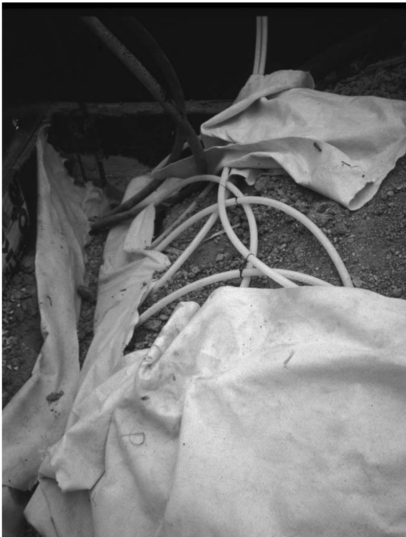
Figure 7.7 Photograph showing installation of ground coils.
