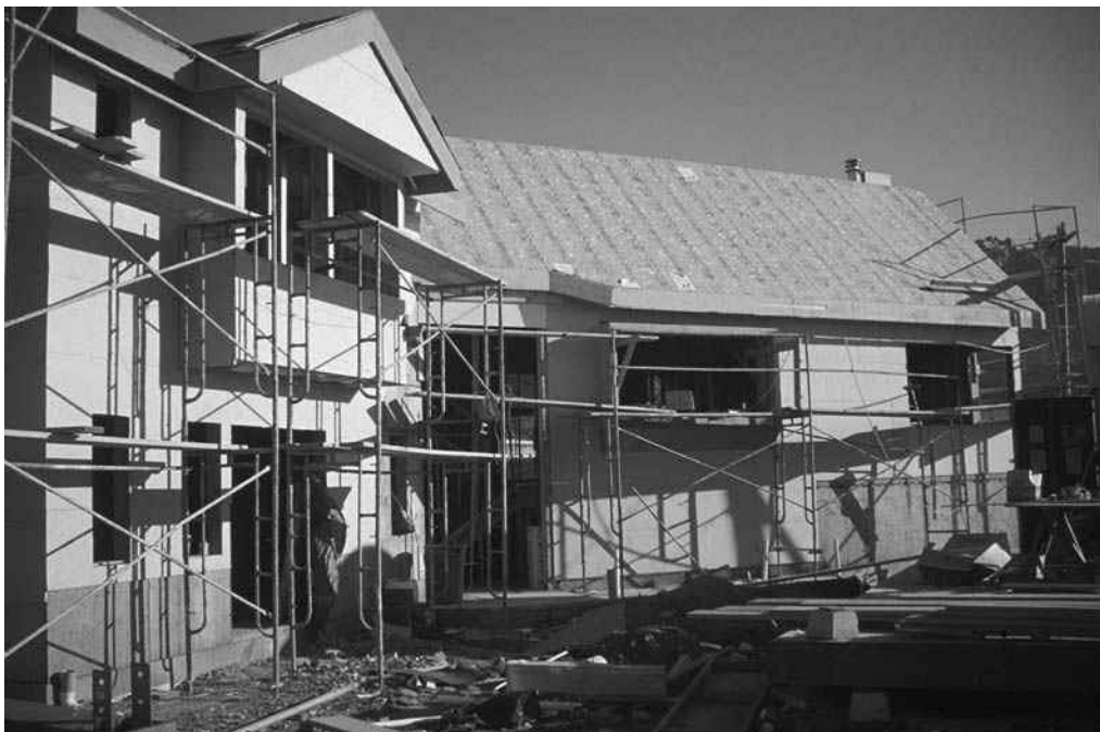
Figure A.8 Completion of the solar roof construction by placement of the R-control panels over the long roof rafters to produce the interior exposed beam vaulted ceiling.
