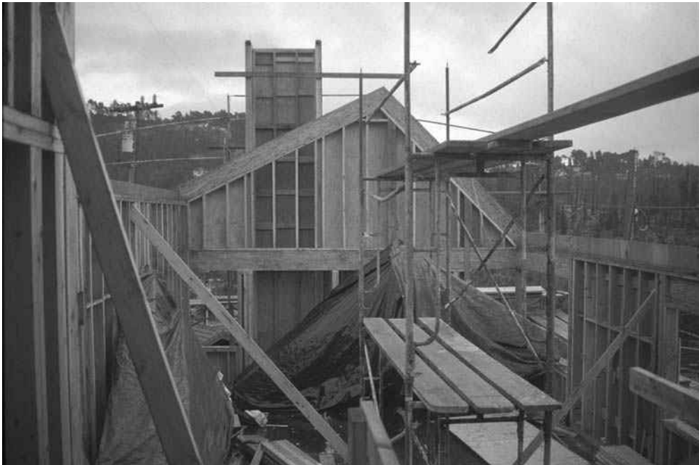
Figure A.6 Inside view of living/kitchen/dining section ready to install long rafters for solar roof.
