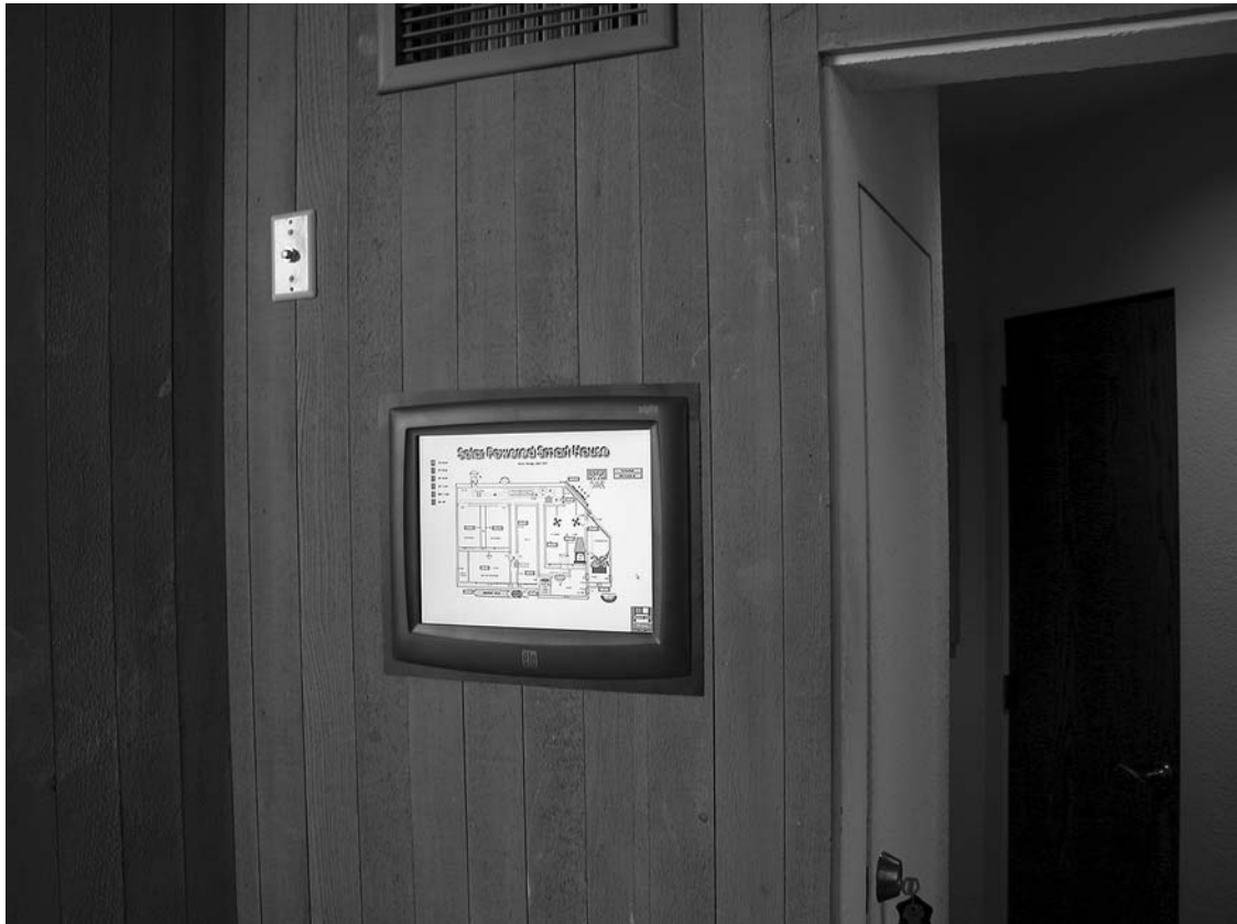
Figure 7.10 Photograph showing color touch screen wall mount.
