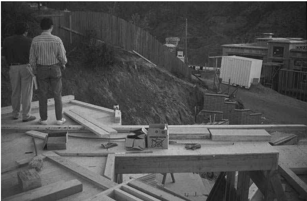
Figure A.2 Architect Ed Nold (left) and general contractor Gary Gerber (right) standing on the start of the second floor on the bridge between the main living/kitchen/dining section to the second floor bedrooms.
