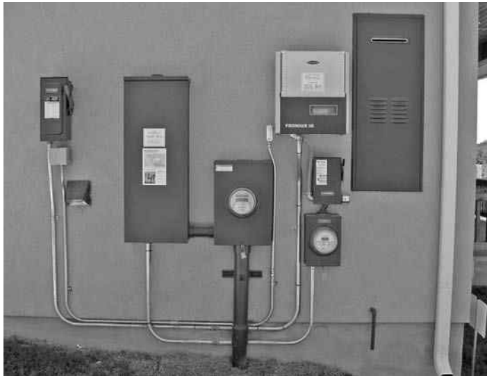
FIGURE 6.14 Utility interactive PV system installation in Austin, Texas (2008). Note the DC and AC disconnects, electric meters, and Fronius inverter.
