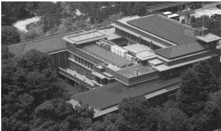
FIGURE 8.2 Installed grid-tied PV array on Japanese prime minister's official residence (Sishokante) signals to the country the government's deep commitment to solar energy.
