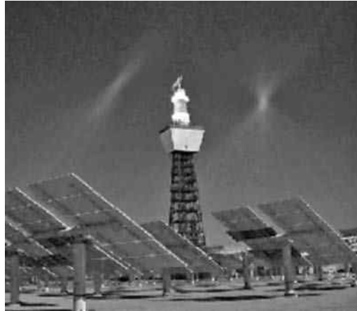
FIGURE 4.19 Primary and secondary focal points seen in the air at the Barstow power tower in California (Courtesy DOE).
