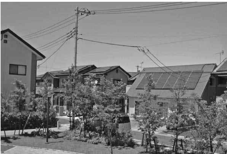
FIGURE 8.1 Ohta City has the highest concentration of grid-tie PV homes, with over 500 homes installed in this neighborhood.
