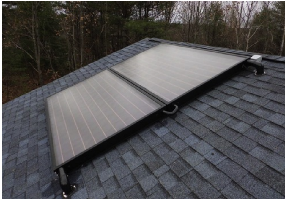
FIGURE 4.10 Wagner solar DHW flat plate collector array. Photo courtesy of ReVision Energy Corp. (For color version of this figure, the reader is referred to the online version of this book.)
