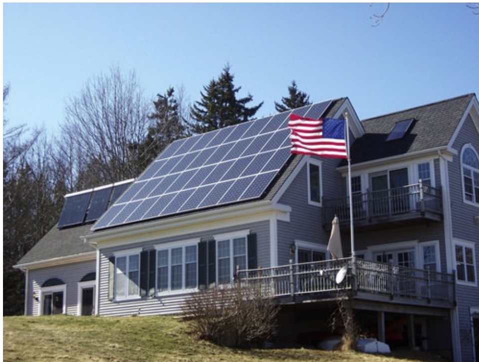
FIGURE 5.4 8.64 kW array composed of 36 Canadian Solar CSP6M
