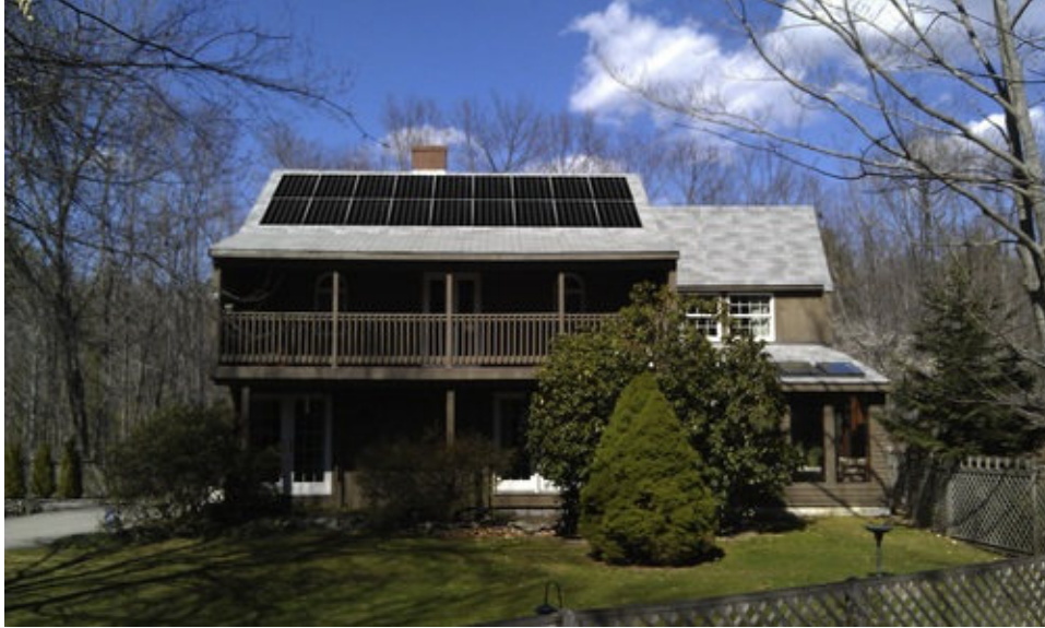
FIGURE 8.2 Proposed 18-panel PV array, New England region. Rendering courtesy of ReVision Energy. (For color version of this figure, the reader is referred to the online version of this book.)
