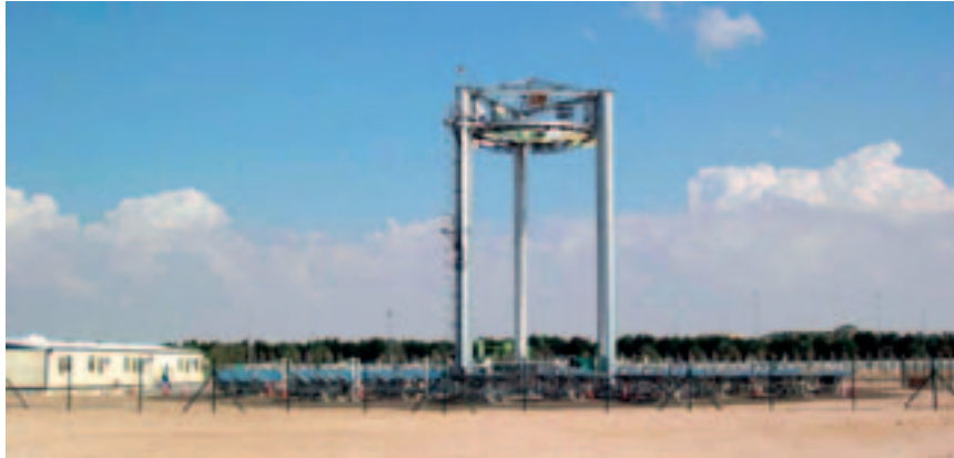
Photo 7.8 Experimental beam-down solar tower in Abu Dhabi
