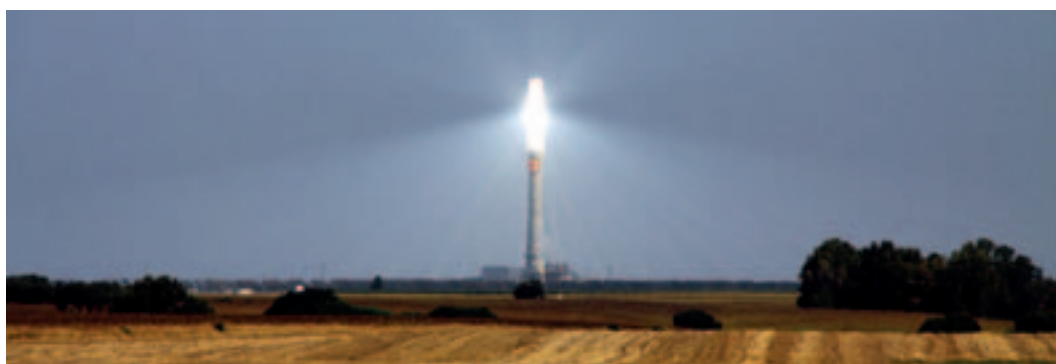
Photo 3.1 The Gemasolar power tower near Sevilla (Spain)
