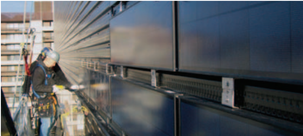
Photo 4.8 Installing a solar air heating system
