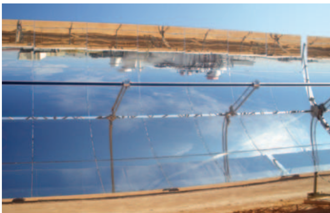
Photo 8.4 A parabolic trough and, reflected, the power block of the Integrated solar combined cycle plant at Ain Beni Mathar, Morocco
