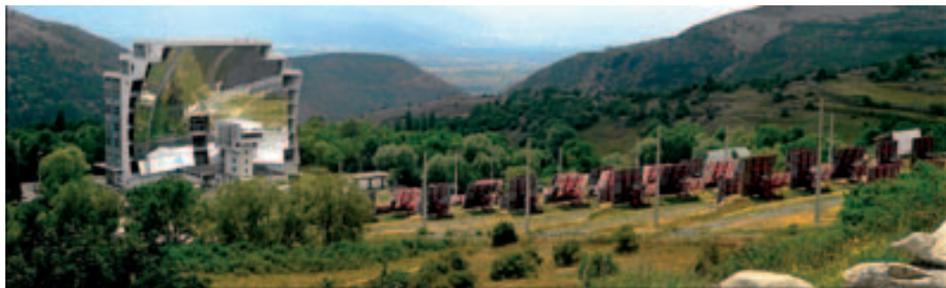
Photo 7.5 The solar oven at Odeillo (France)
