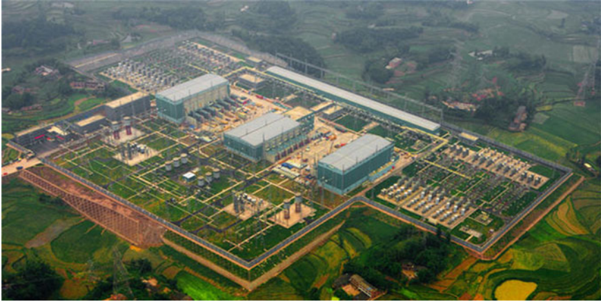
Fig. 3.49 The \pm 800 kV converter substation Fulong-Xiangjiaba-Shanghai (Source ABB AG)
