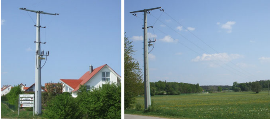
Fig. 4.16 Transition from 20 kV overhead lines to cable at the border of urban areas
