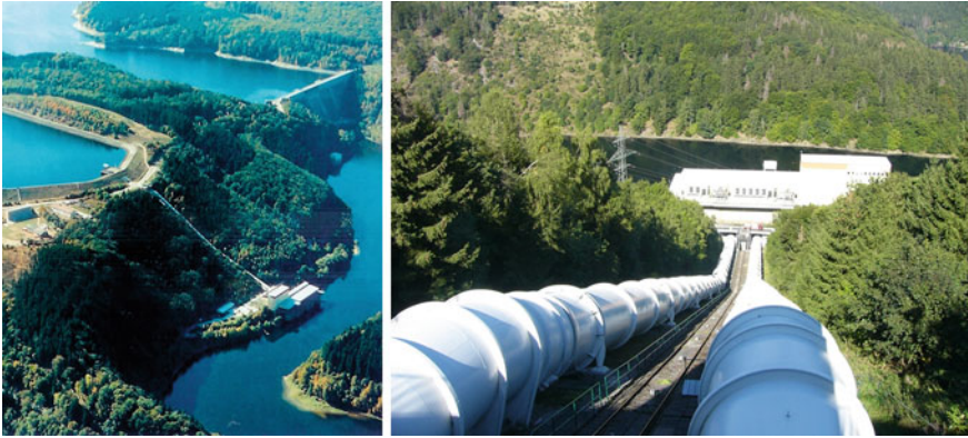
Fig. 2.23 Views of the Wendefurth pump storage landscape and of the tube system ( Source Regenerativ-Kraftwerk Harz GmbH and Co.KG)
