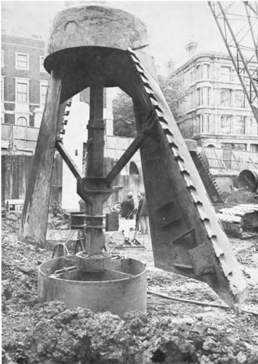
Figure 3.30 Top-hinged under-reaming bucket.
