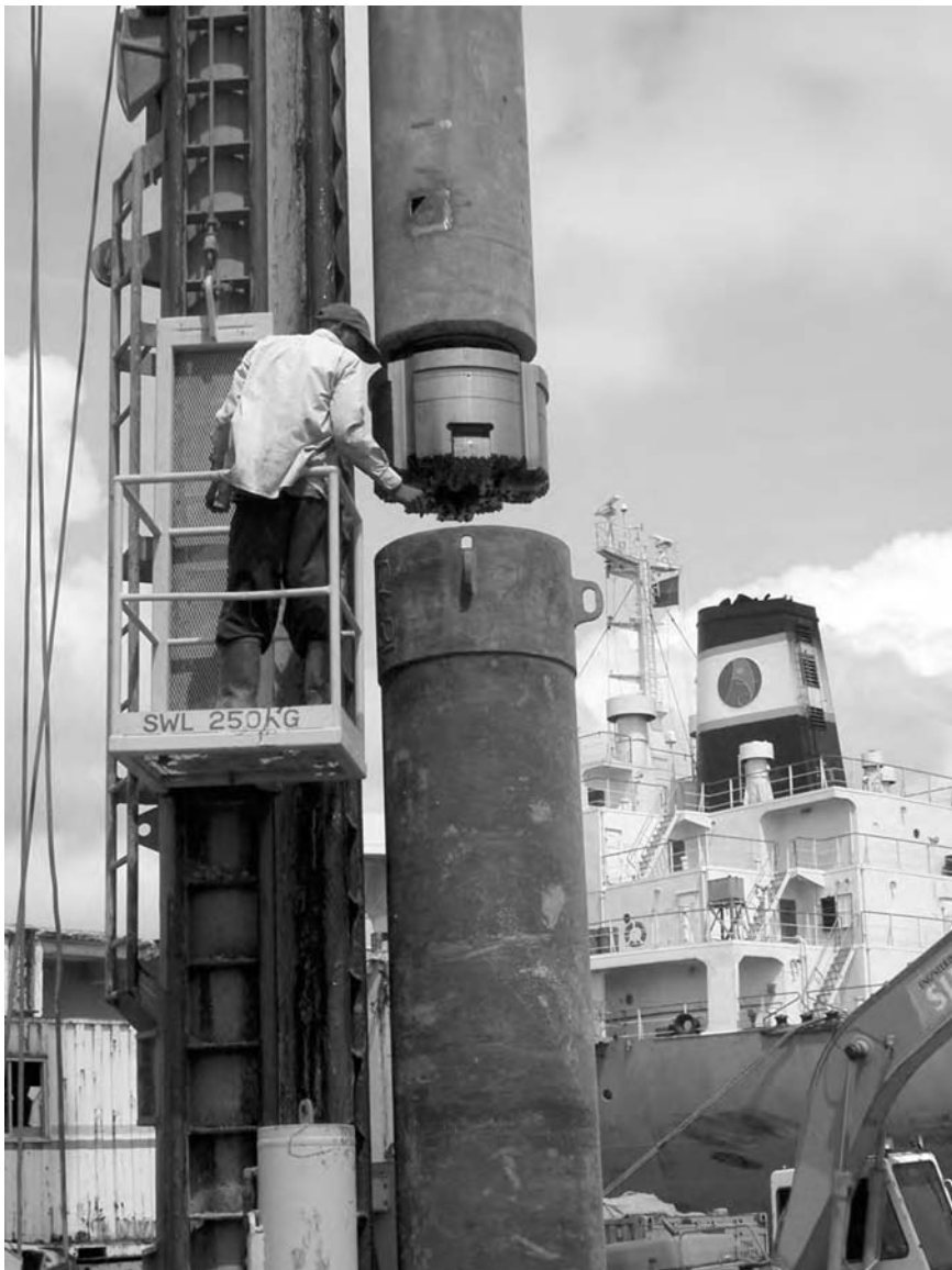
Figure 3.32 Numa hammer with extending under-reaming drill bit for simultaneously drilling and inserting casing (courtesy Numa Hammers).
