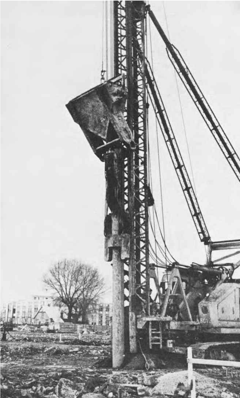
Figure 3.24 Discharging concrete into the driving tube of a withdrawable tube pile. Concreting skip travelling on pile frame leaders.
