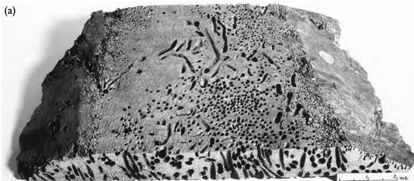
Figure 10.2 Attack on timber piles by marine borers (Crown copyright reproduced with permission of BRE) (a) Attack by Teredo (b) Attack by limnoria .
