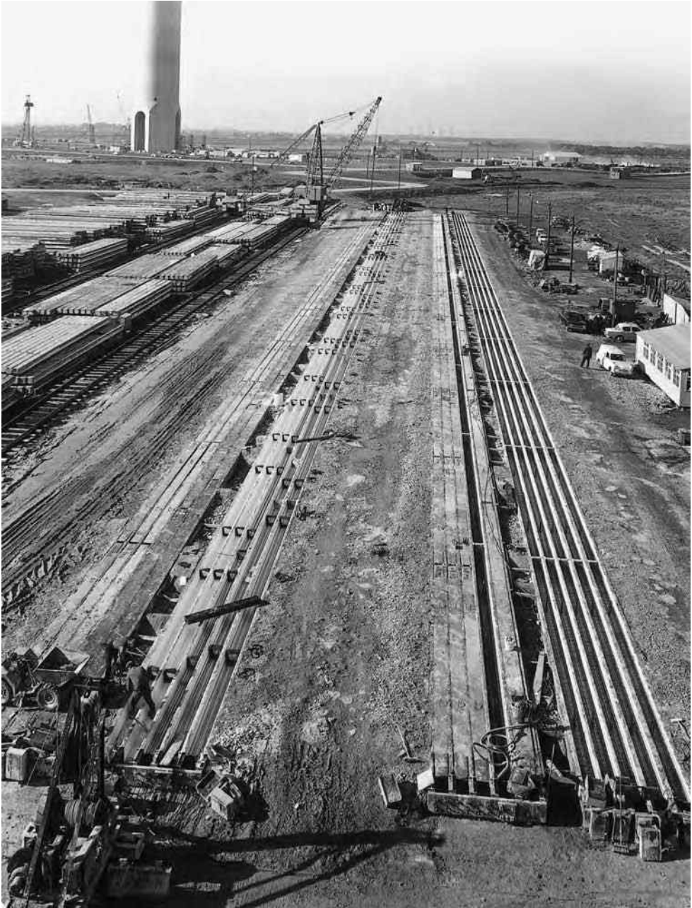
Figure 2.11 Casting yard for prestressed concrete piles at Drax Power Station.
