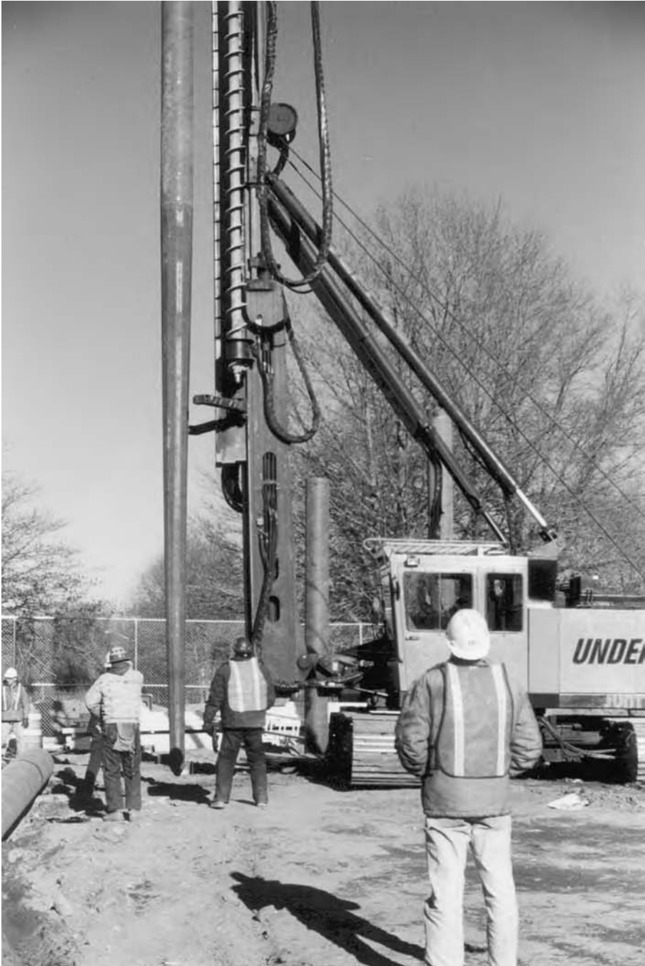
Figure 2.28 The TaperTube pile.
