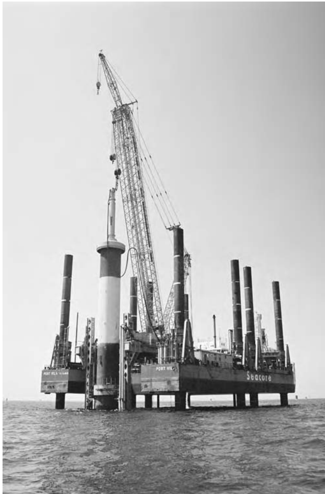
Figure 3.13 Driving a 4 m dia monopile foundation for North Hoyle offshore wind farm using a Menck MHU 500T hammer with large diameter pile sleeve and anvil adapter (courtesy Seacore Ltd).
