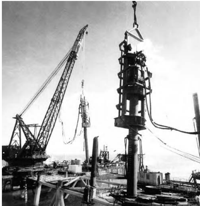
Figure 3.12 MRBS air/steam single-acting hammer with stabilizing cage driving 54 inch diameter piles in legs of offshore jacket platform (courtesy Menck GmbH).
