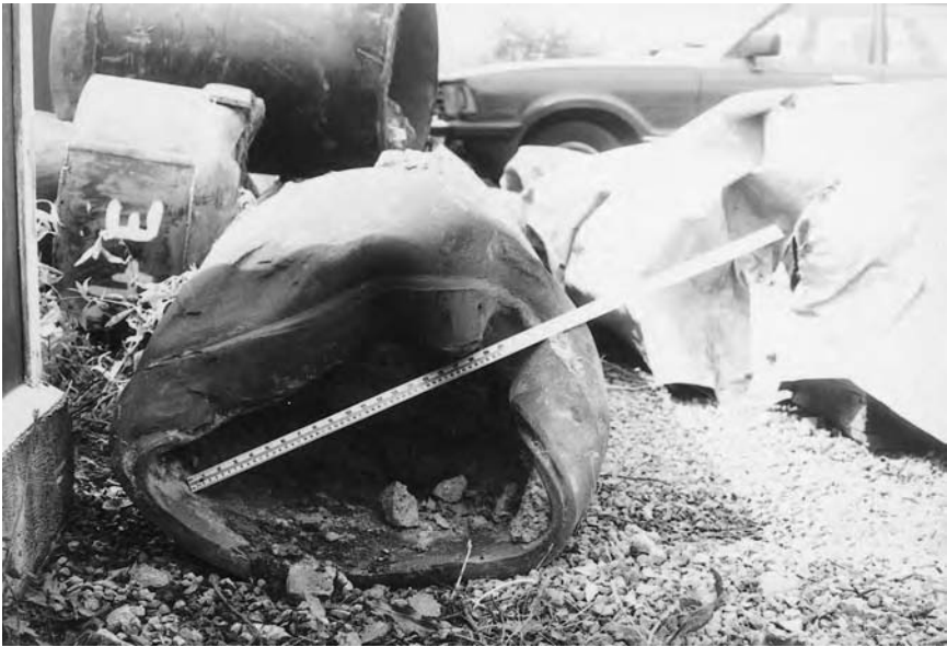
Figure 2.24 (a) Strengthening shoe of tubular steel pile by cruciform plates (b) Buckling and tearing of welded-on external stiffening ring to tubular steel pile driven on to sloping rock surface.
