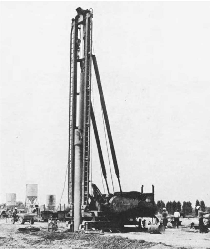
Figure 3.23 Franki pile-driving rig.
