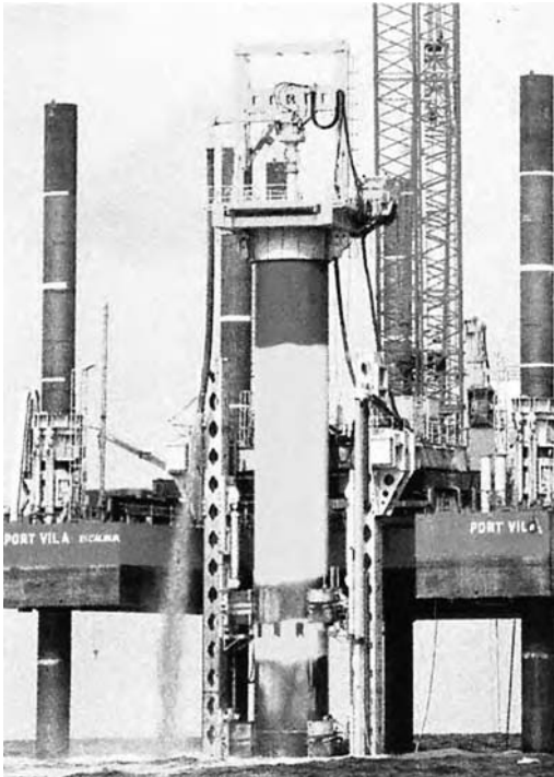
Figure 3.7 Installing a 4 m dia monopile foundation for North Hoyle offshore wind farm with pile top rig and specially designed leader leg pile frame (courtesy Seacore Ltd).
